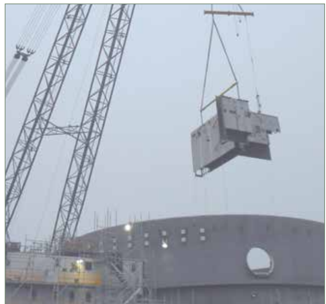
The CA05 structural module is placed at V.C. Summer Unit 2.
