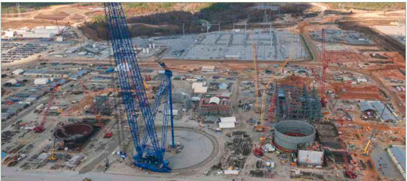
An aerial perspective of the Vogtle Unit 3 and 4 construction site.
