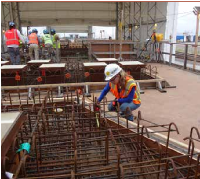
Top, the Vogtle Unit 4 containment vessel bottom head.
