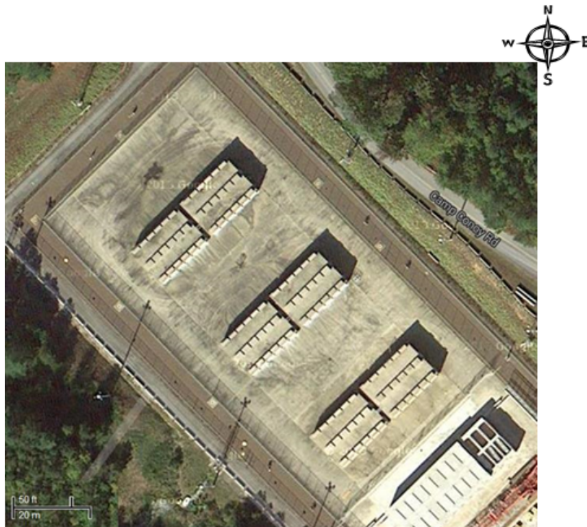
Figure 2-1. Aerial view of the Calvert Cliffs Nuclear Power Station ISFSI housing HSM-1 and HSM-15 modules [imagery © U.S. Geological Survey, Map Data © Google Inc. 2013]
