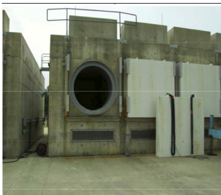
Figure 1-1. NUHOMS horizontal storage modules in Calvert Cliffs Nuclear Power Station ISFSI [from Suffield et al. 2012]
