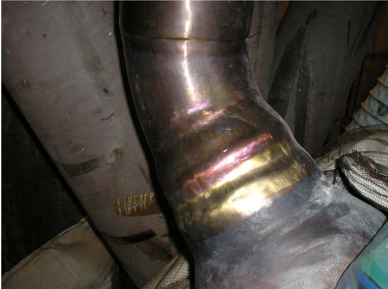
Figure C.8 Photograph of Pressurizer Safety and Relief Nozzle, Nozzle Weld, and Safe End
