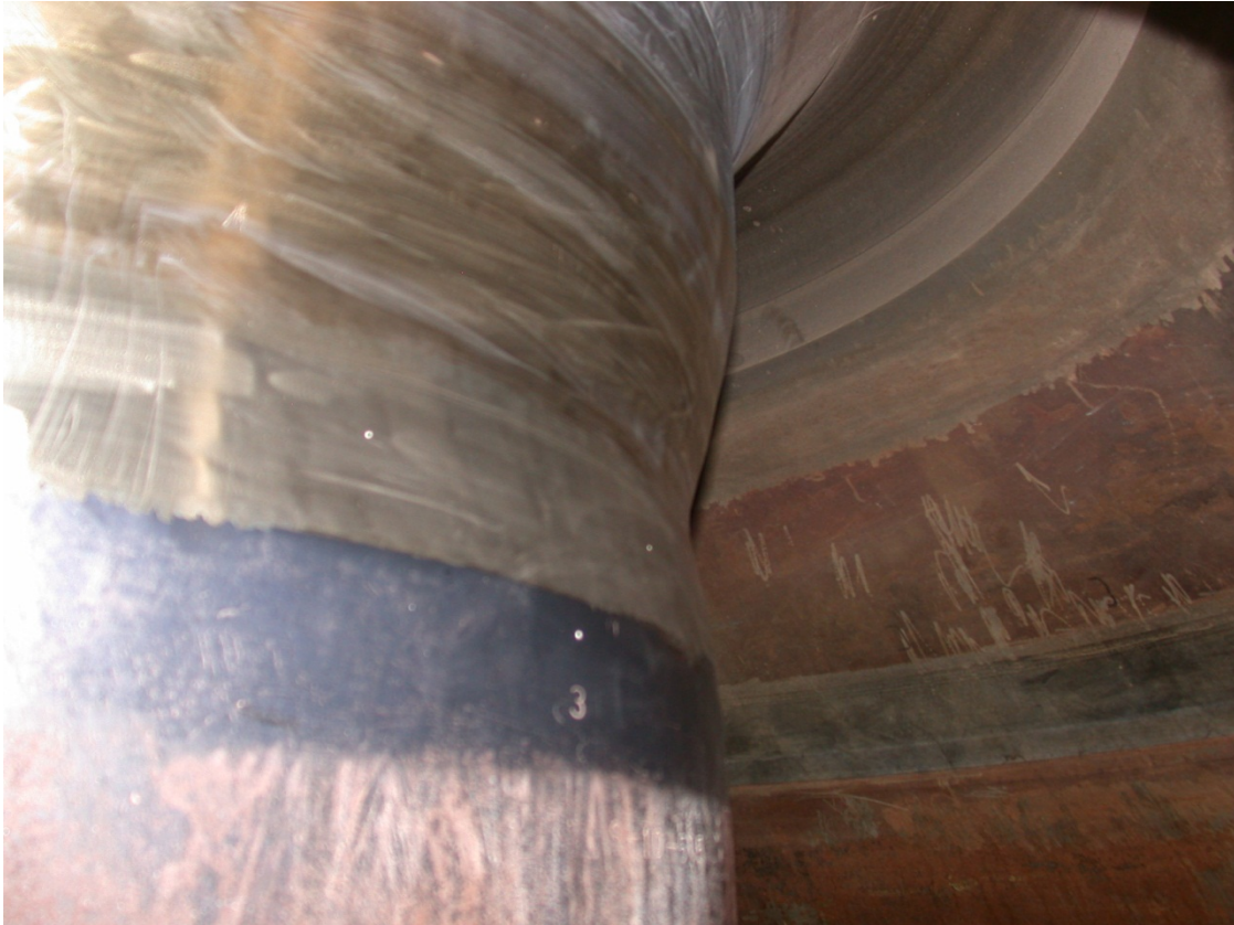
Figure D.2 Photograph of RCP Suction Nozzle, Nozzle Weld, and Safe End
