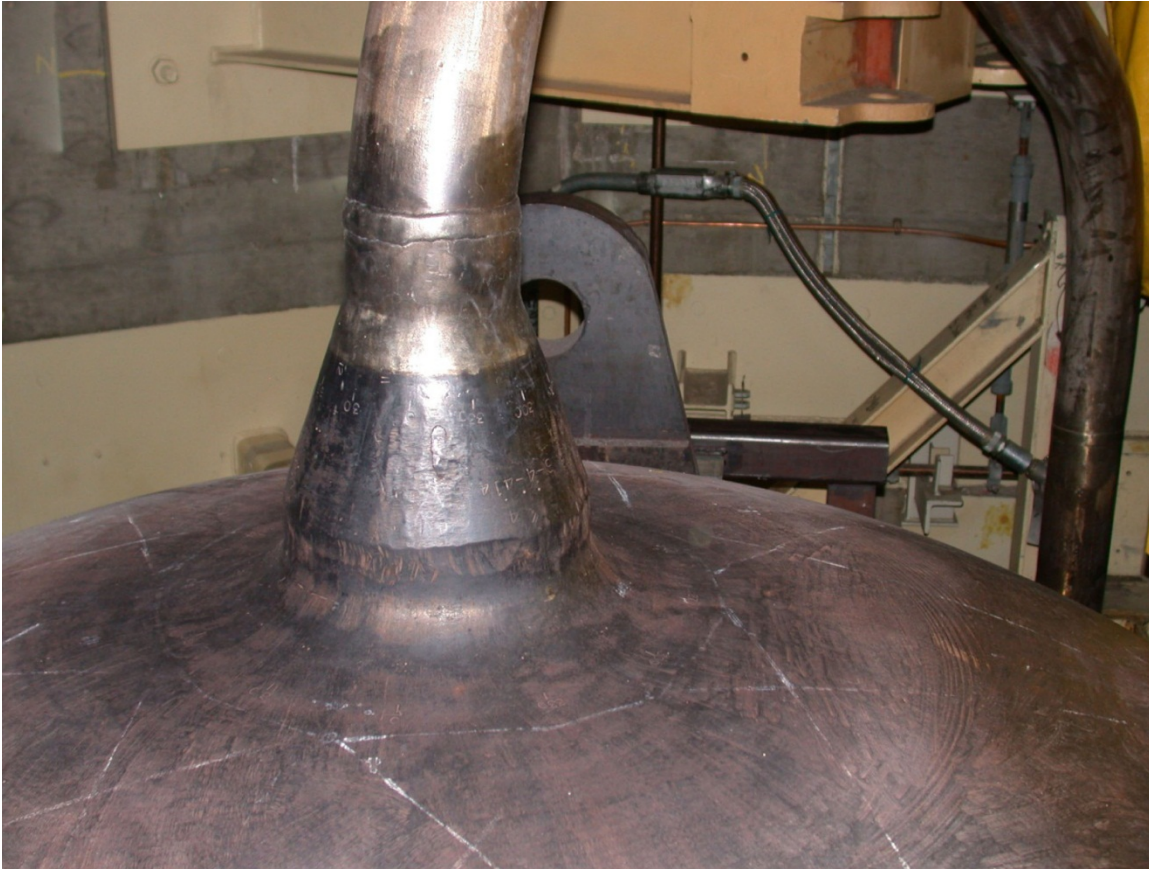
Figure D.32 Photograph of Pressurizer Spray Nozzle, Nozzle Weld, and Safe End
