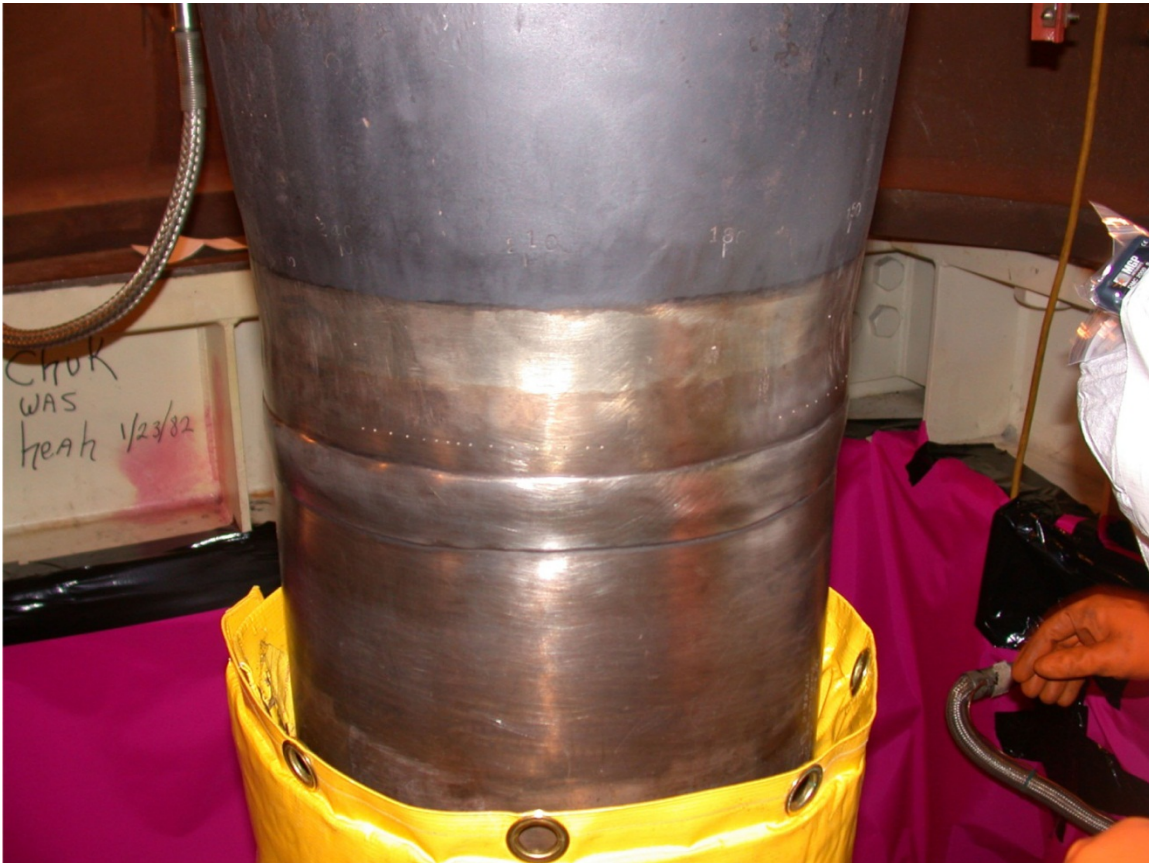
Figure D.29 Photograph of Pressurizer Surge Nozzle, Nozzle Weld, and Safe End
