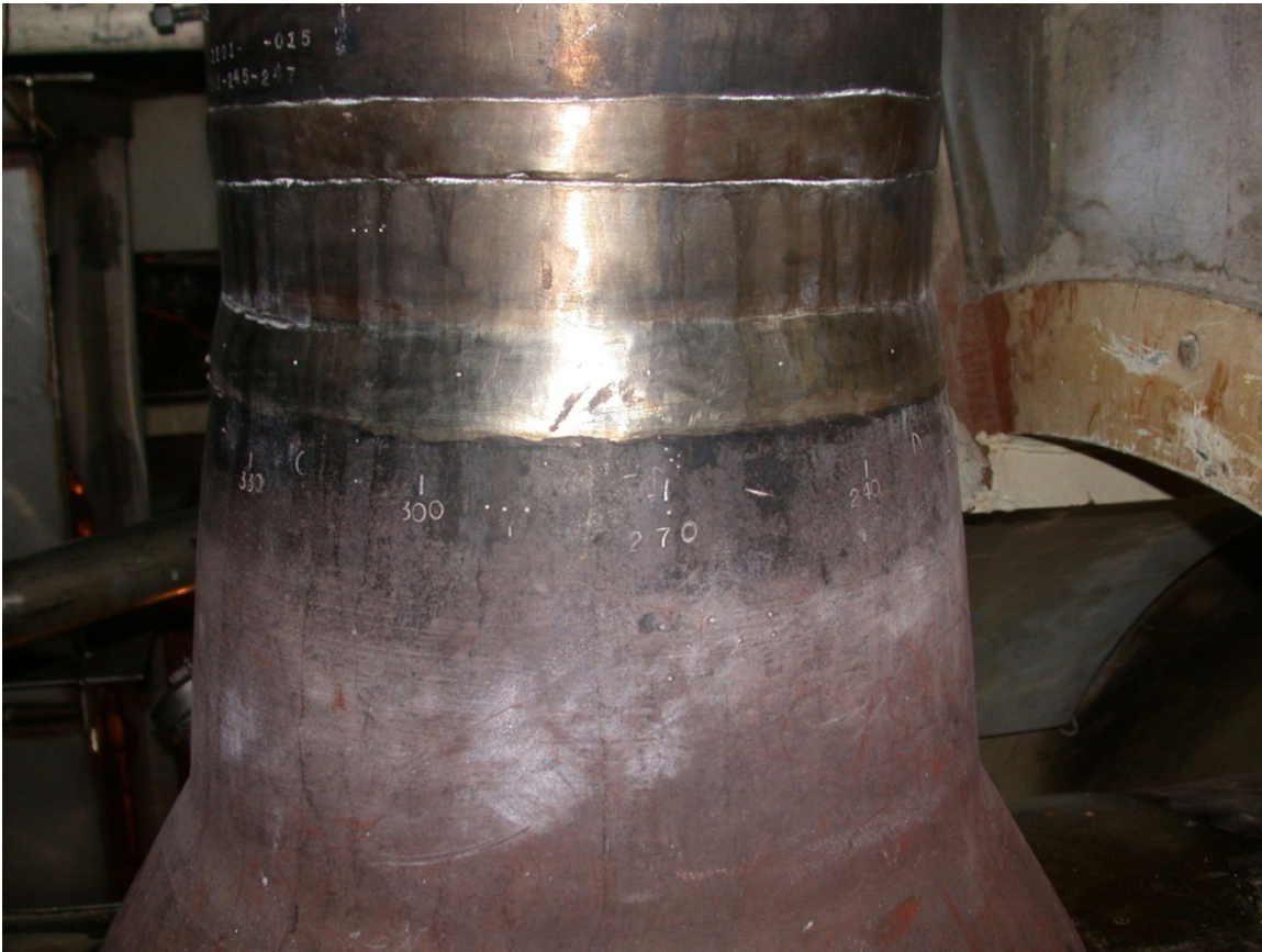
Figure D.8 Photograph of Surge Nozzle, Nozzle Weld, and Safe End
