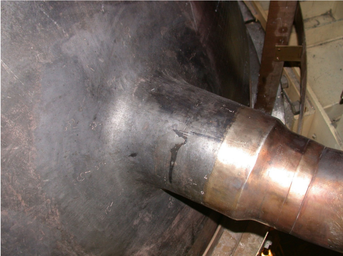
Figure D.35 Photograph of Pressurizer Safety & Relief Nozzle, Nozzle Weld, and Safe End
