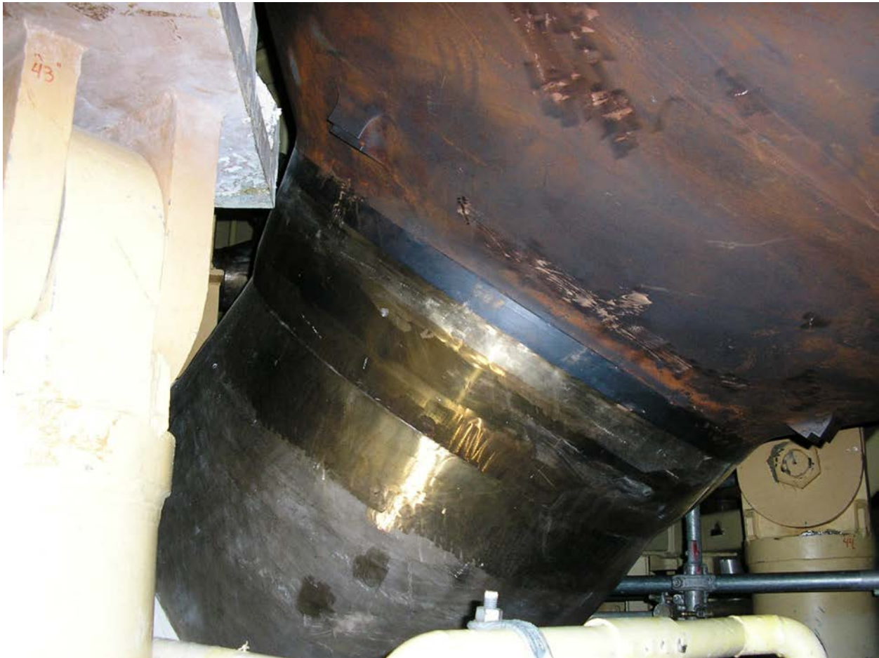
Figure C.16 Photograph of Steam Generator Cold Leg Nozzle, Nozzle Weld, and Safe End
