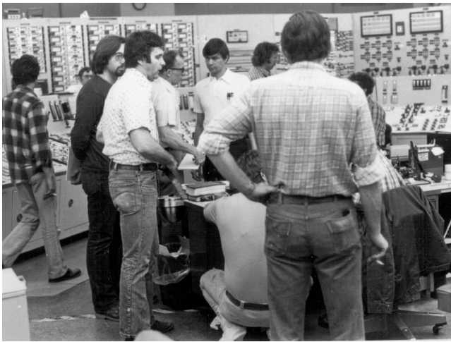
Figure 12: Adding to the confusion reactor operators experienced during the accident at Three Mile Island was a noisy and crowded control room environment.
