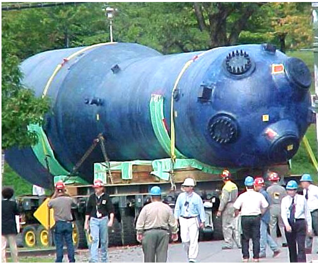
Figure 5: Despite their size and their permanent appearance, most aging components in a nuclear power plant can be replaced. Pictured above is a new steam generator to be installed at the Indian Point Energy Center in New York.
