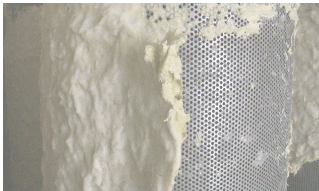
Figure 9: Testing revealed that fine particulates from reactor piping insulation could break loose after a loss-of-coolant event, clog sump screens, and limit the sump systems' performance. This long-standing generic issue was resolved for all nuclear power plants.
