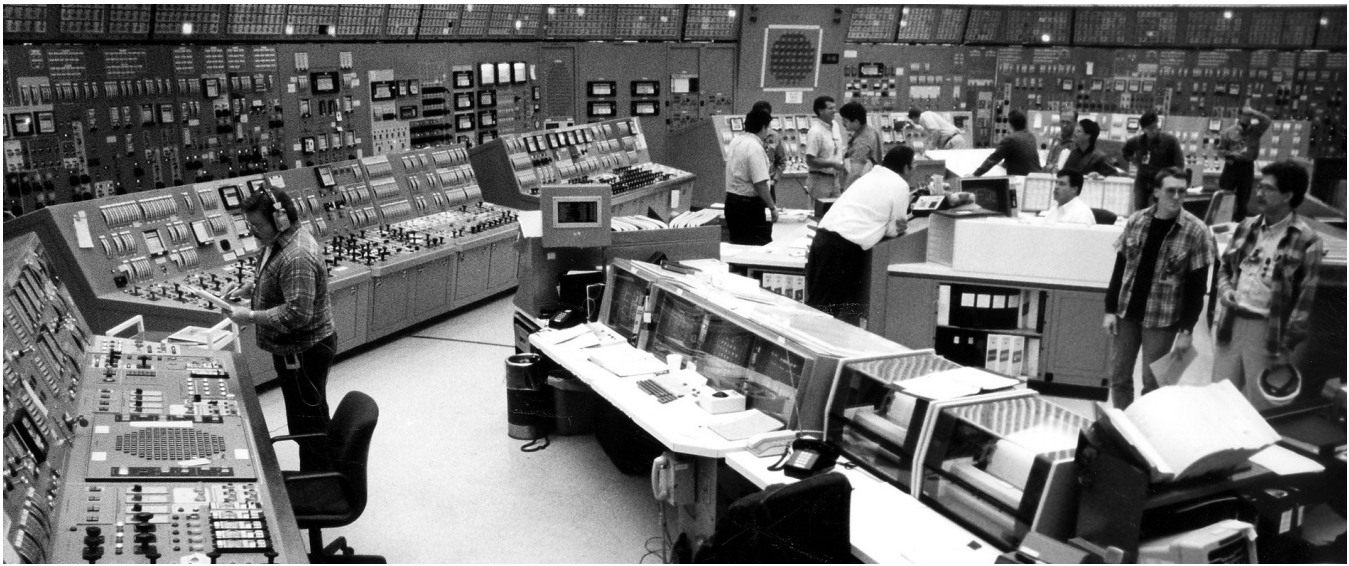
Figure 11: By the 1970s, reactor plant control rooms had become very complex and contributed to operator error, most notably during the Three Mile Island accident in 1979.
