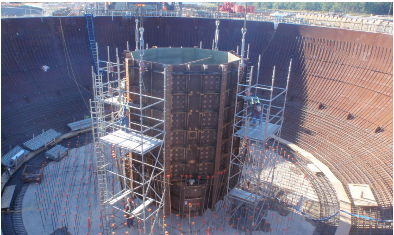
At the site, located near Jenkinsville, SC, the V.C. Summer Unit 2 reactor vessel cavity is moved into place.
