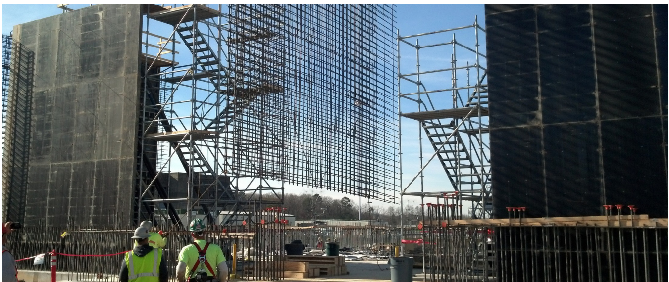
Rebar placement for a “flex” building wall at the Watts Bar Unit 2—one of several enhancements to the facility that the Tennessee Valley Authority is undertaking as part of the NRC’s Fukushima Order.
