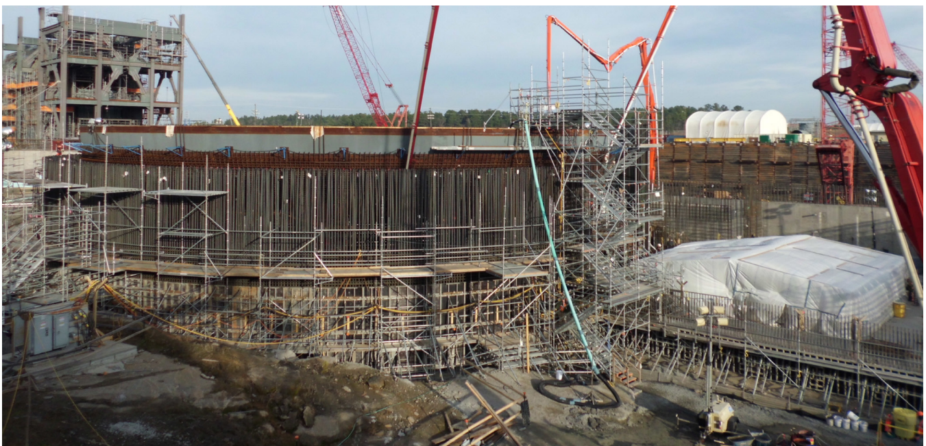
At the V.C. Summer site in South Carolina, a look at the concrete pump truck setup for under containment vessel bottom head Layer A.
