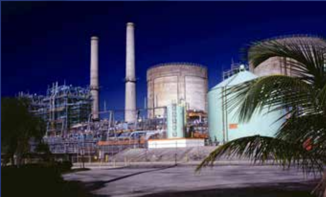
Photo courtesy of Florida Power & Light Company
