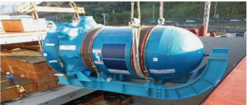
Vogtle Unit 3 (AP1000) nuclear island; rebar placement in preparation for concrete basemat pour (Top). Vogtle Unit 3 reactor pressure vessel arrives in the United States (Bottom). Courtesy of Georgia Power, a Southern Company.
