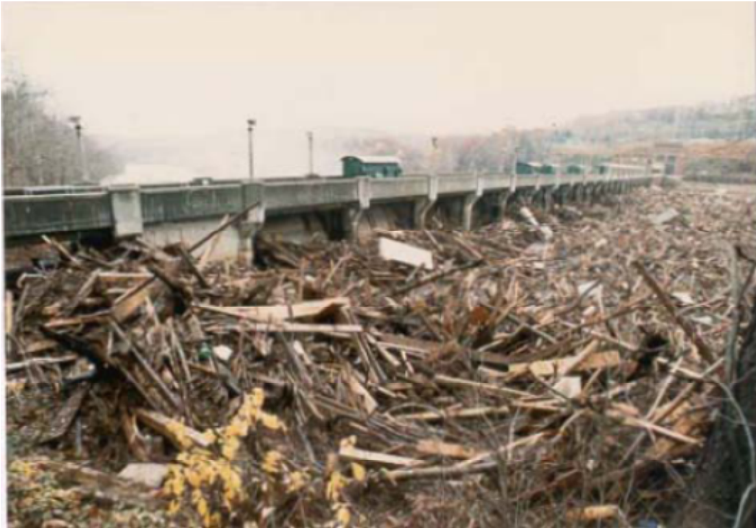
Figure 17. Debris Upstream of Lake Lynn Dam after 1985 Flood Event (Schadinger et al., 2012)
