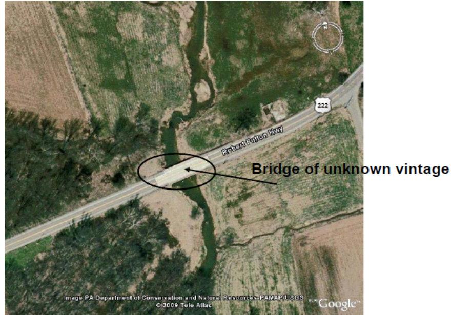
Figure 6-16 Bridge along Robert Fulton Highway
