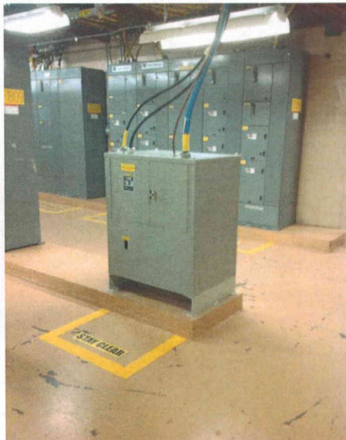
File Name: 2-62-10-1-06.jpeg Description: General view of component
