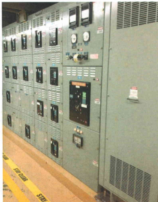
File Name: 2-62-2-4-06.jpeg Description: General view of component
