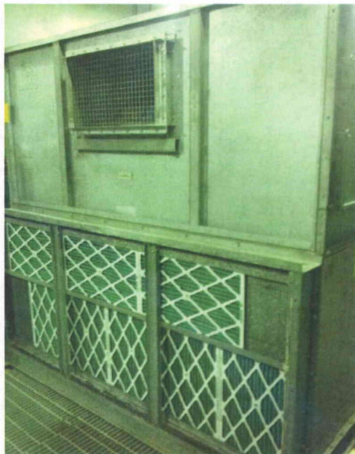
File Name: 2-62-15-4-18.jpeg Description: General view of Component
