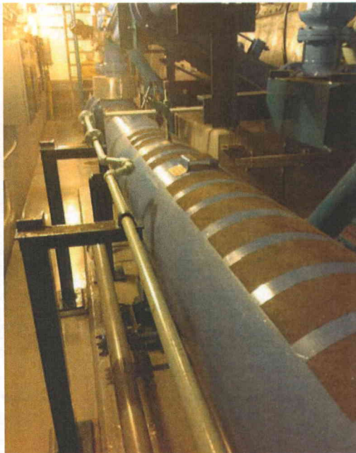
File Name: 2-62-9-4-08.jpeg Description: General view of Component
