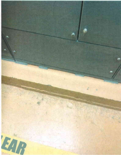
File Name: 2-63-5-4-22.jpeg Description: View of base anchorage detail
