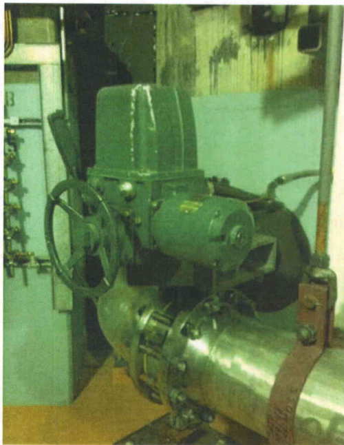
File Name: 2-62-1-4-16.jpeg Description: General view of Component
