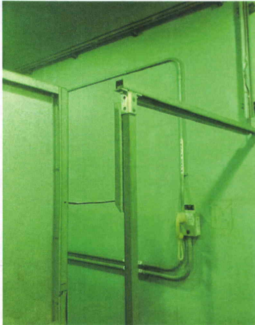
File Name: 2-95-9-4-18.jpeg Description: View of component wall mounted bracing
