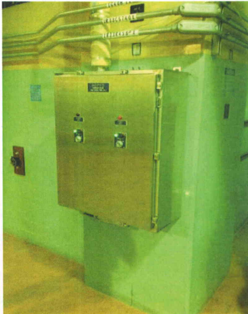
File Name: 2-62-3-4-22.jpeg Description: General view of component
