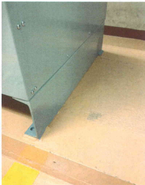
File Name: 2-64-13-4-06.jpeg Description: View of base anchorage detail
