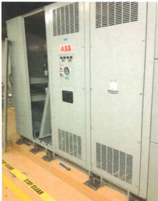
File Name: 2-62-1-4-06.jpeg Description: General view of component
