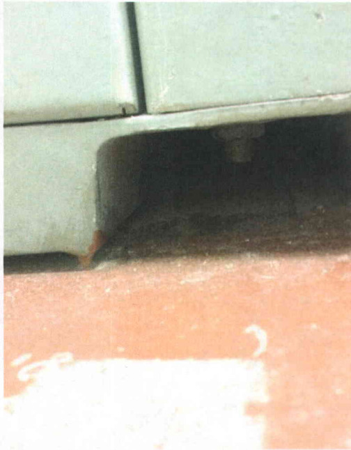
File Name: 2-63-9-4-22.jpeg Description: View of anchor bolts at base
