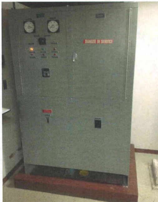
File Name: 2-62-2-4-02.jpeg Description: General view of component
