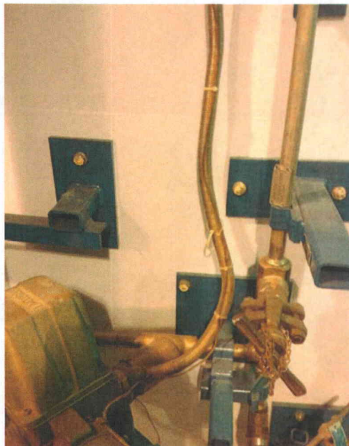
File Name: 2-64-2-4-14.jpeg Description: View of wall support HSS members
