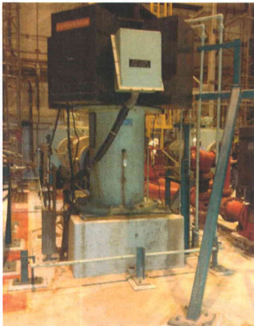
File Name: 2-62-7-4-05.jpeg Description: General view of component
