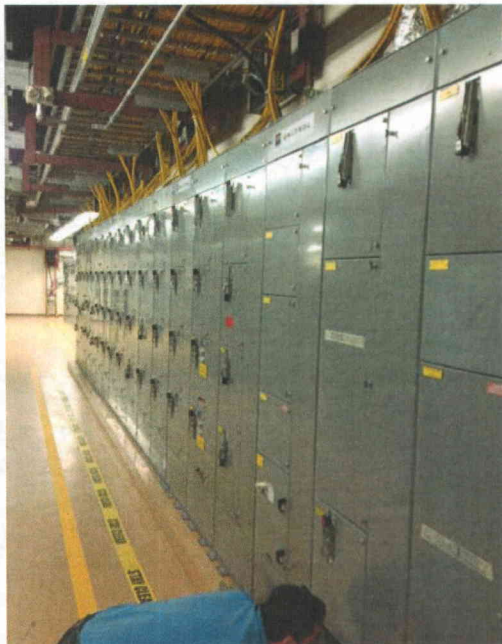
File Name: 2-62-8-4-06.jpeg Description: General view of component
