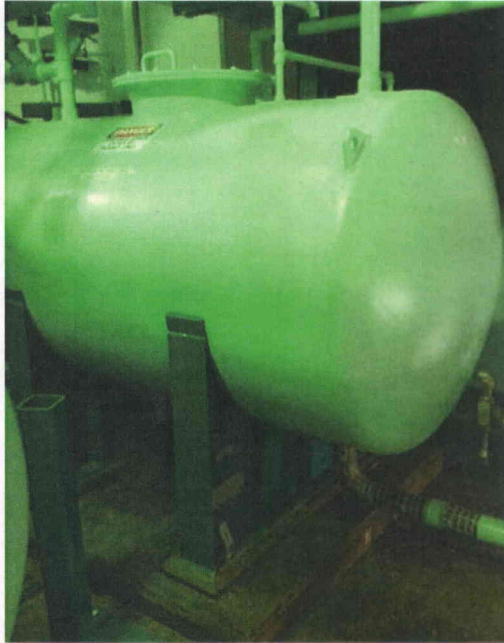
File Name: 2-61-1-4-11.jpeg Description: General view of component
