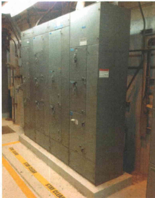
File Name: 2-62-1-4-05.jpeg Description: General view of component
