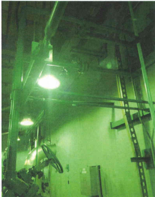
File Name: 2-94-9-4-18.jpeg Description: View of pipe line wall supported bracing
