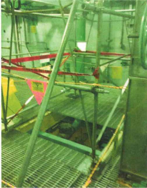
File Name: 2-95-15-4-18.jpeg Description: Scaffolding located near component
