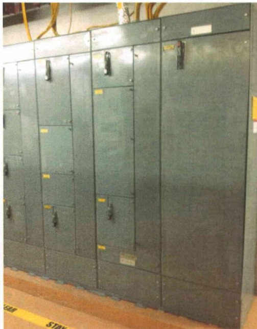
File Name: 2-62-12-4-06.jpeg Description: General view of component
