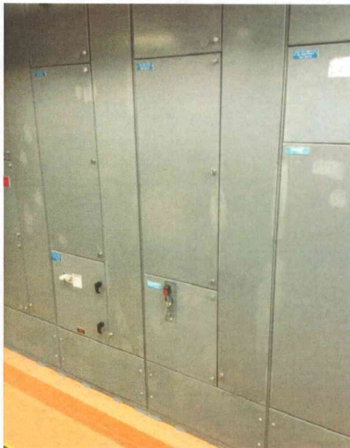
File Name: 2-62-6-4-22.jpeg Description: General view of component
