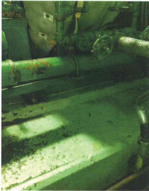
File Name: 2-63-2-4-18.jpeg Description: View of anchorage configuration
