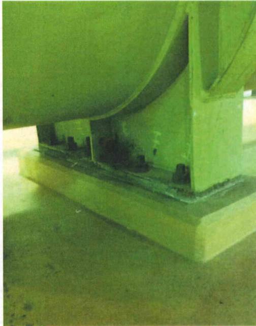
File Name: 2-73-4-4-01.jpeg Description: View of anchorage detail
