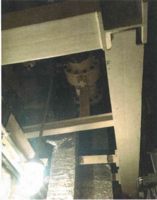
File Name: 2-61-6-4-12.jpeg Description: General view of component location
