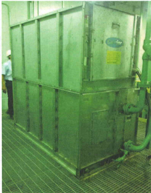
File Name: 2-62-9-4-18.jpeg Description: General view of Component
