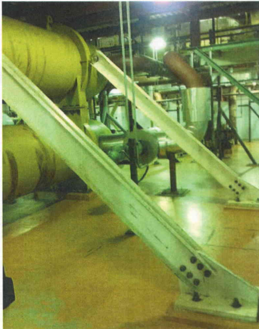
File Name: 2-94-4-4-01.jpeg Description: View of lateral bracing
