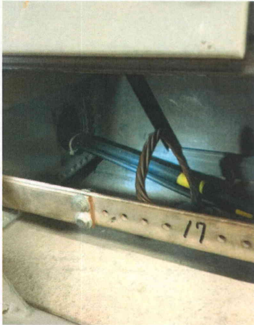
File Name: 2-63-8-4-06.jpeg Description: Inside view of component
