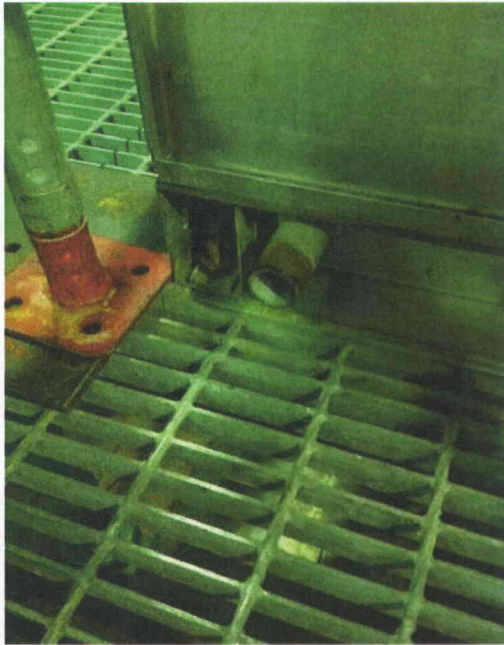
File Name: 2-63-5-1-19.jpeg Description: View of anchorage detail
