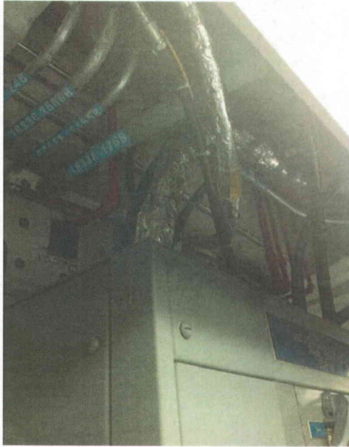
File Name: 2-73-9-4-22.jpeg Description: View of top attached lines
