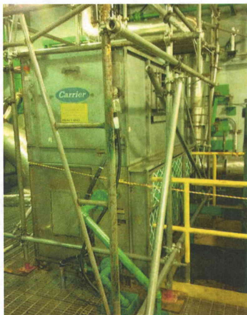
File Name: 2-62-5-1-19.jpeg Description: General view of component
