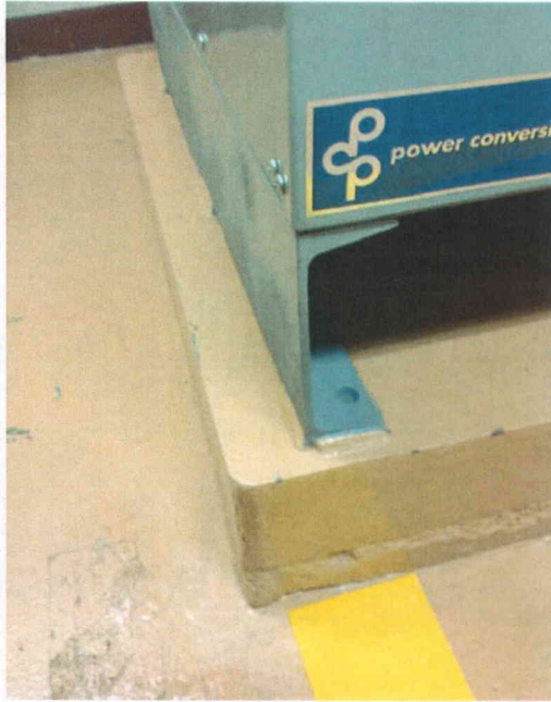
File Name: 2-63-13-4-06.jpeg Description: View of base anchorage detail
