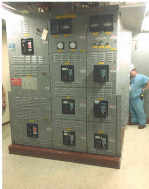
File Name: 2-62-3-4-02.jpeg Description: General view of component
