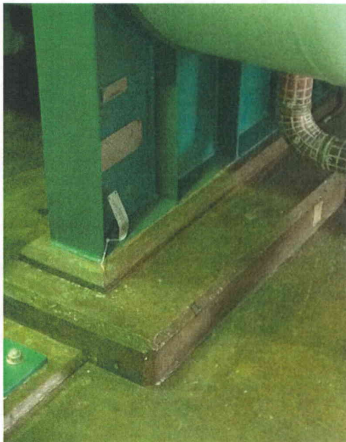
File Name: 2-62-1-4-11.jpeg Description: View of anchorage detail
