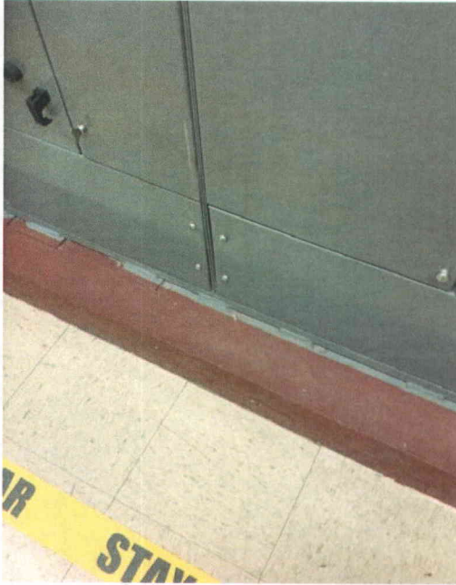
File Name: 2-63-7-4-22.jpeg Description: View of base anchorage detail
