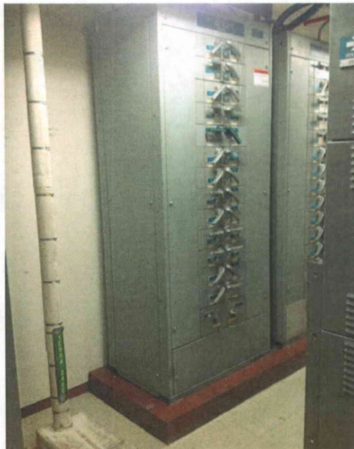
File Name: 2-62-9-4-22.jpeg Description: General view of component
