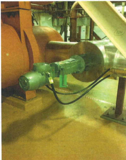
File Name: 2-62-2-1-01.jpeg Description: General view of component
