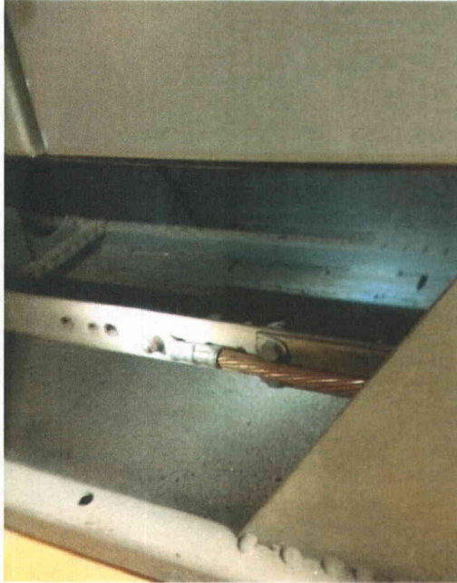
File Name: 2-63-3-4-06.jpeg Description: View of center weld detail at base
