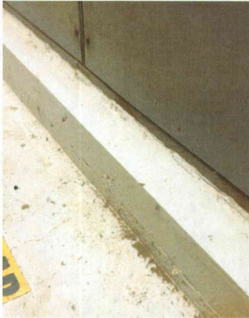
File Name: 2-64-1-4-05.jpeg Description: Close up view of component concrete pad
