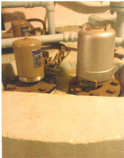
File Name: 2-64-4-4-08.jpeg Description: Overall view of top of component
