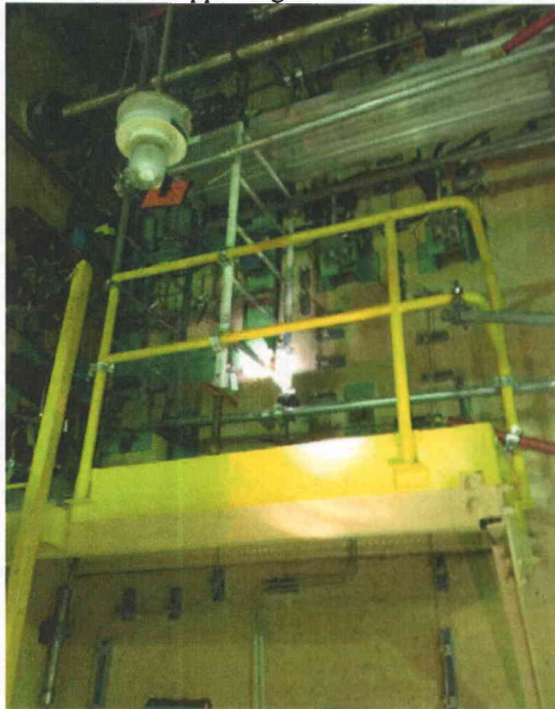
File Name: 2-61-4-4-18.jpeg Description: General view of component location
