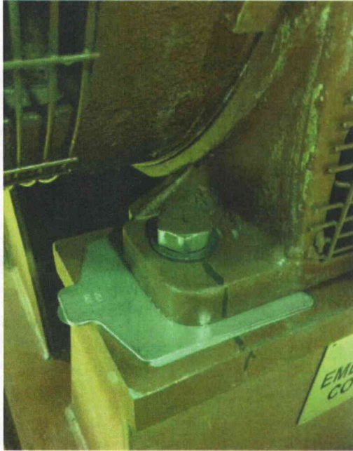
File Name: 2-63-9-1-01.jpeg Description: Typical anchorage for pump to skid
