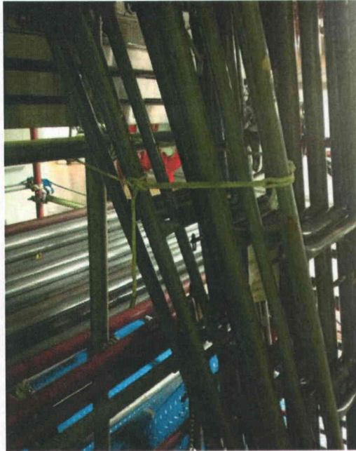
File Name: 2-73-2-4-22.jpeg Description: View of ties for scaffolding staging
