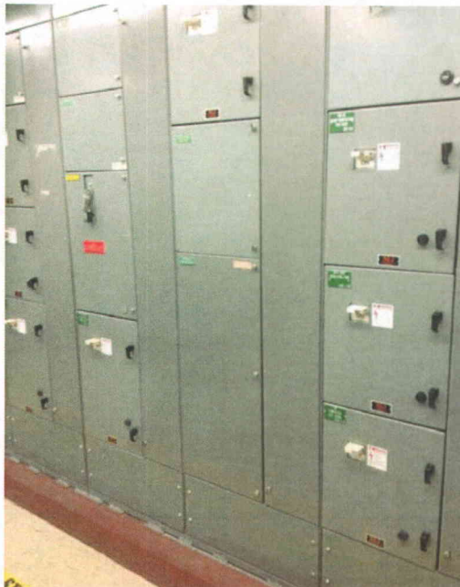
File Name: 2-62-7-4-22.jpeg Description: General view of component
