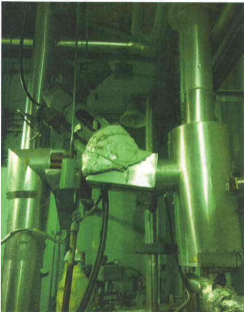
File Name: 2-62-1-4-18.jpeg Description: General view of component
