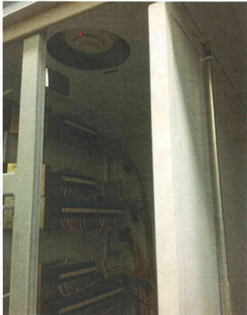
File Name: 2-63-1-4-02.jpeg Description: Inside view of component
