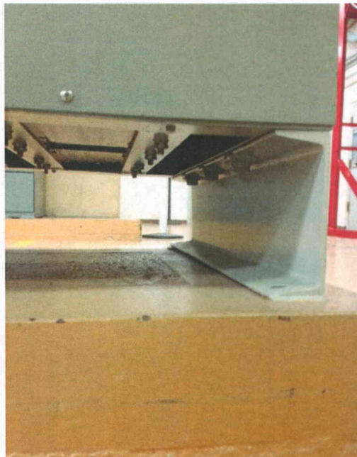
File Name: 2-64-10-1-06.jpeg Description: View of base anchorage detail
