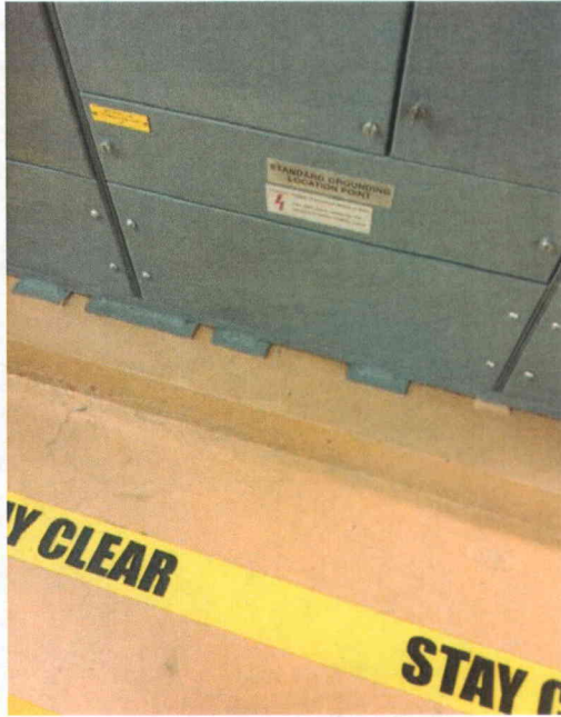
File Name: 2-63-12-4-06.jpeg Description: View of base anchorage detail
