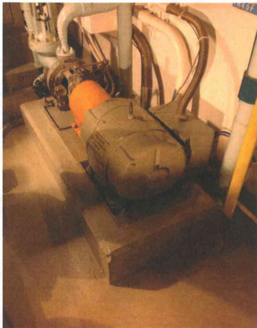
File Name: 2-62-16-4-08.jpeg Description: General view of Component
