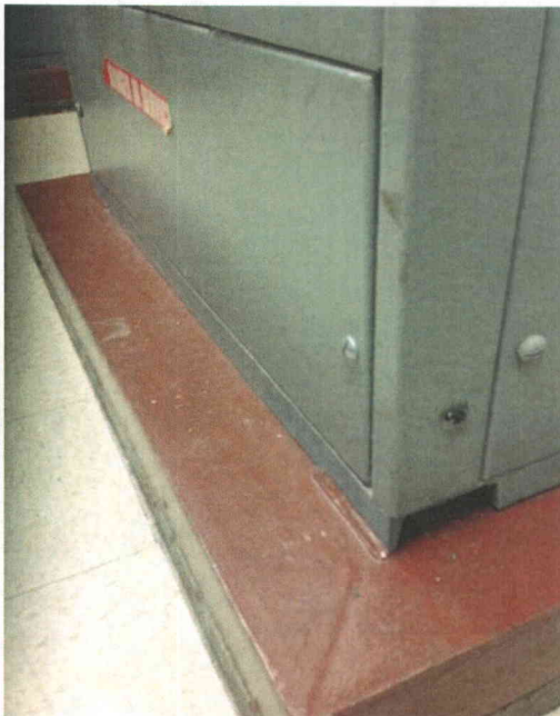
File Name: 2-64-8-4-22.jpeg Description: View of base anchorage detail
