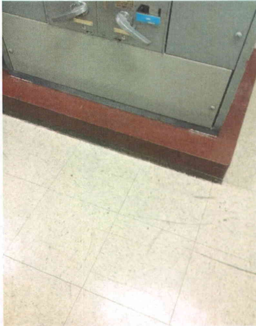
File Name: 2-63-10-4-22.jpeg Description: View of base anchorage detail
