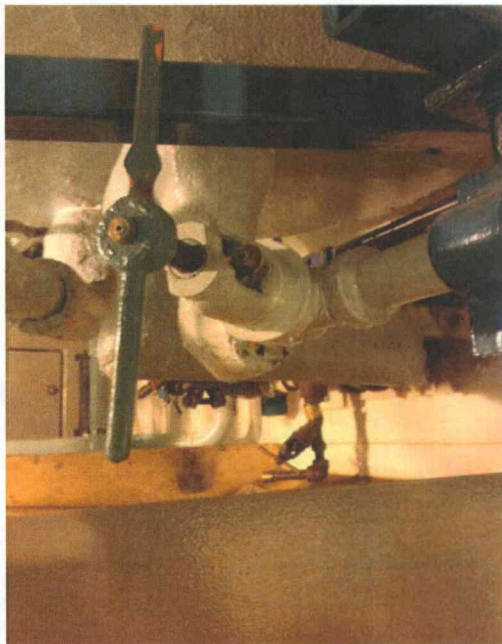
File Name: 2-62-4-4-08.jpeg Description: View of attached lines below tank
