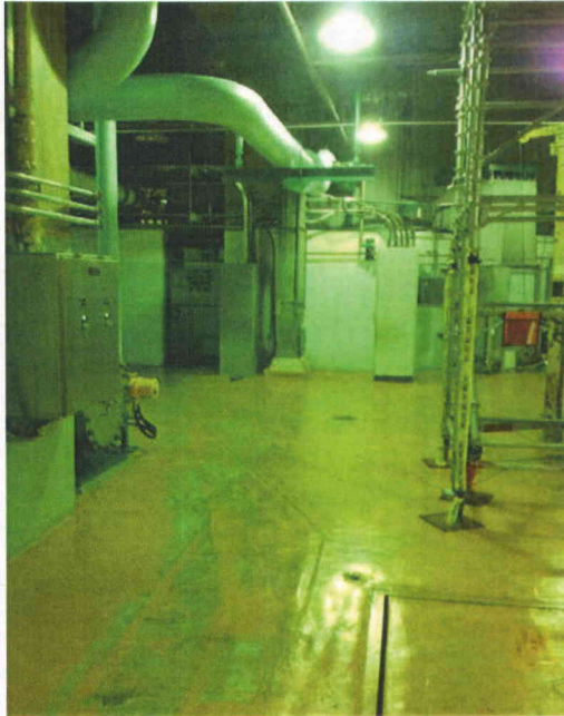
File Name: 2-73-3-4-22.jpeg Description: Scaffolding located in the area
