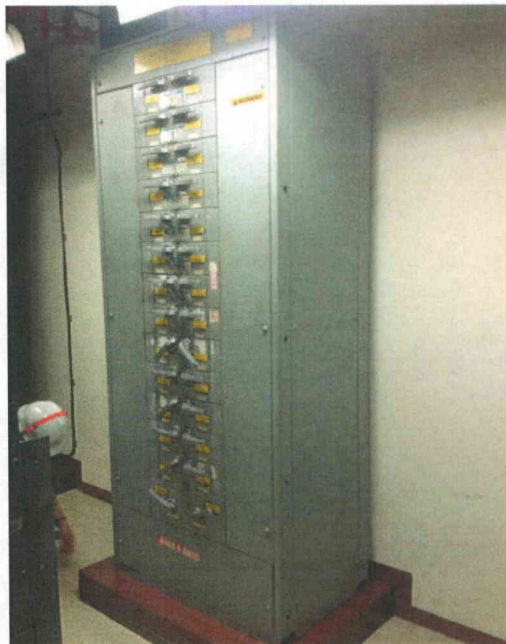
File Name: 2-62-8-4-22.jpeg Description: General view of component
