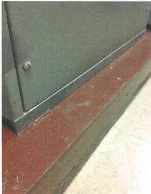
File Name: 2-64-9-4-22.jpeg Description: View of base anchorage detail
