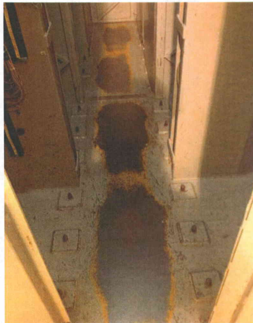
File Name: 2-94-10-4-08.jpeg Description: View of anchorage from inside of cabinet
