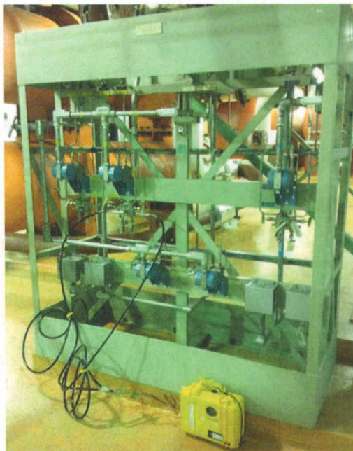
File Name: 2-62-6-4-01.jpeg Description: General view of component
