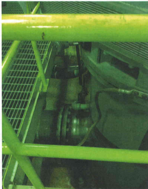
File Name: 2-64-14-4-18.jpeg Description: View of attached lines to component
