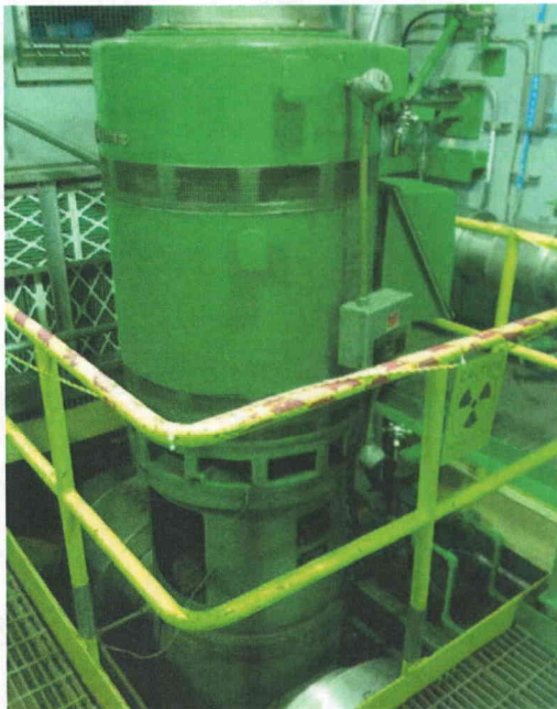
File Name: 2-62-2-4-19.jpeg Description: General view of component
