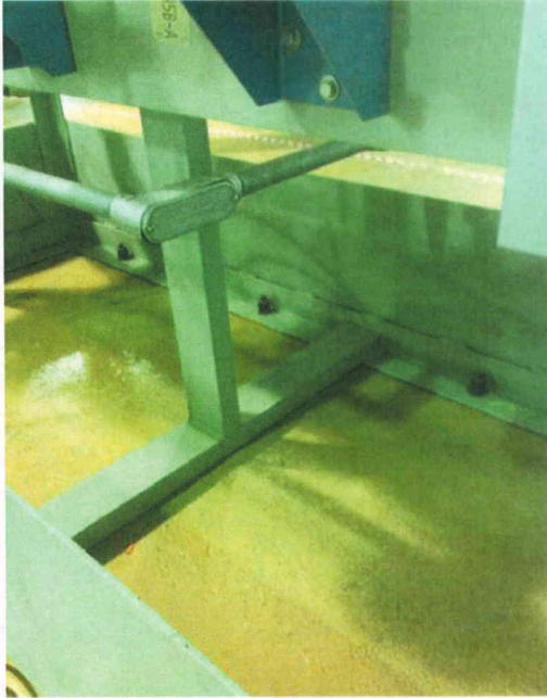
File Name: 2-63-6-4-01.jpeg Description: Anchorage view of component
