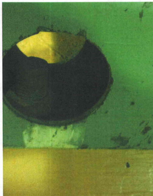
File Name: 2-94-8-4-01.jpeg Description: View of anchorage condition
