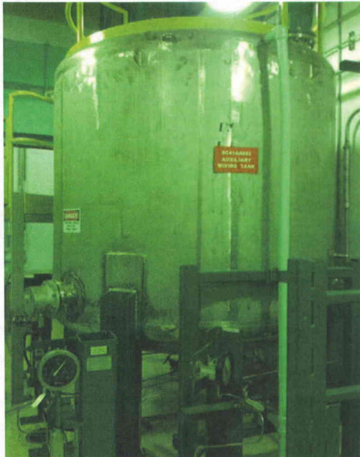
File Name: 2-62-1-4-09.jpeg Description: General view of Component
