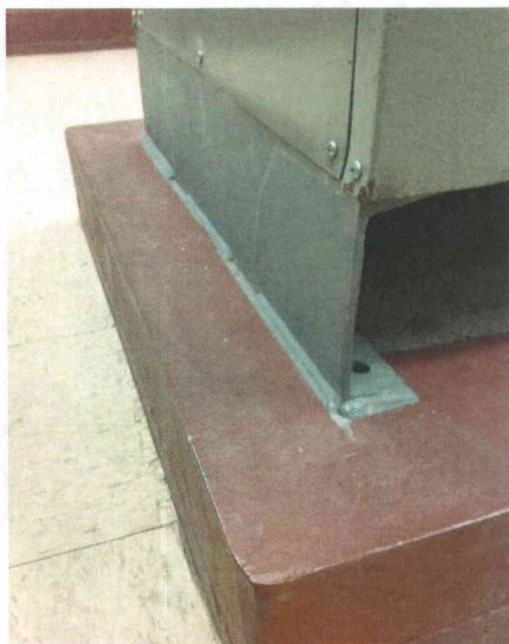
File Name: 2-64-6-1-06.jpeg Description: View of base anchorage detail
