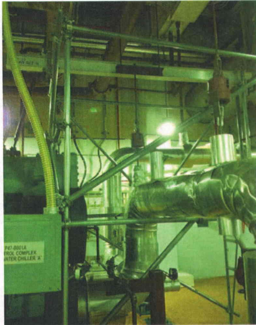
File Name: 2-63-8-4-01.jpeg Description: Scaffolding located in the area
