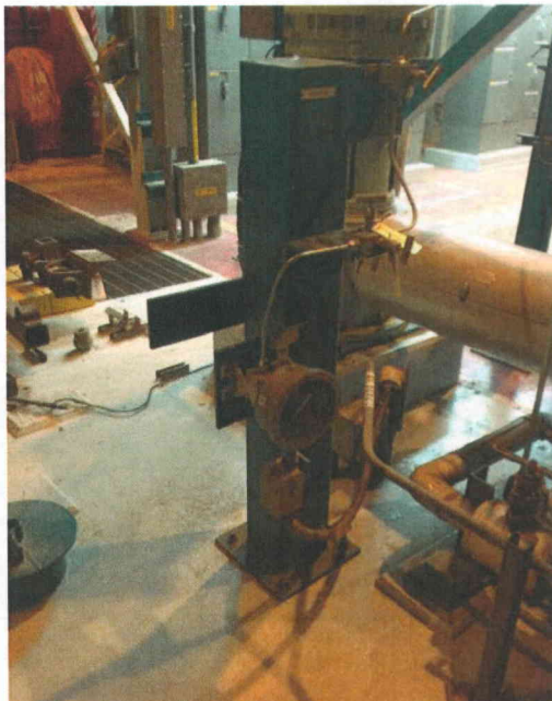
File Name: 2-62-3-1-05.jpeg Description: Attached lines with adequate flexibility
