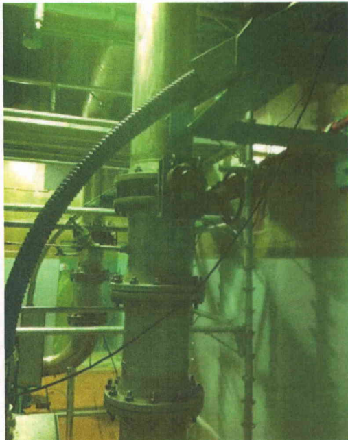
File Name: 2-62-7-1-21.jpeg Description: General view of component
