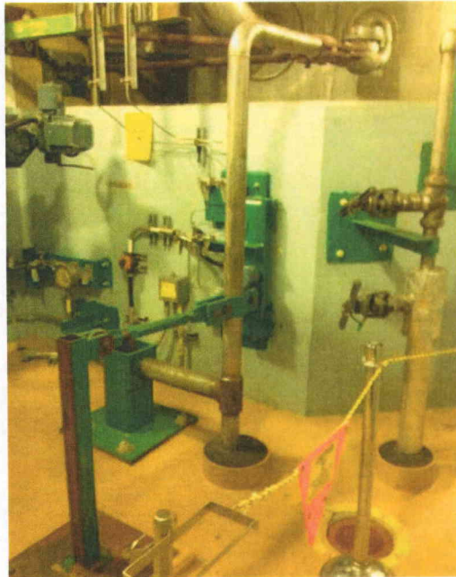
File Name: 2-63-1-4-22.jpeg Description: View of attached lines to component
