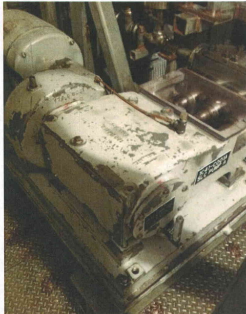
File Name: 2-62-1-4-12.jpeg Description: General view of Component
