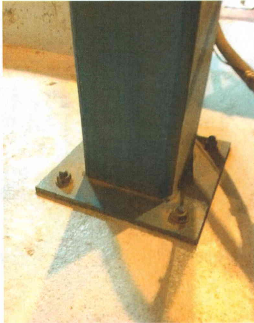
File Name: 2-63-3-1-05.jpeg Description: Anchorage view of component
