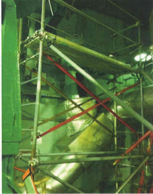
File Name: 2-61-3-4-20.jpeg Description: Scaffolding located in the area
