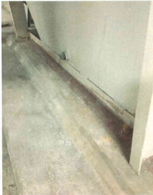
File Name: 2-63-3-4-04.jpeg Description: General view of anchorage
