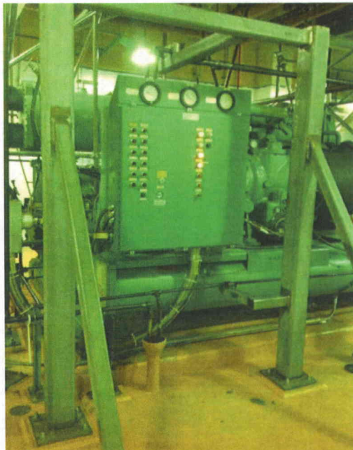
File Name: 2-62-1-1-01.jpeg Description: General view of component
