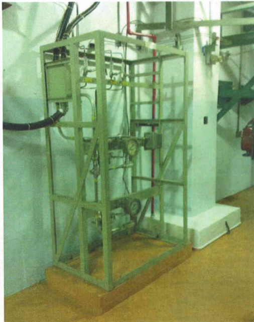
File Name: 2-62-7-4-01.jpeg Description: General view of component
