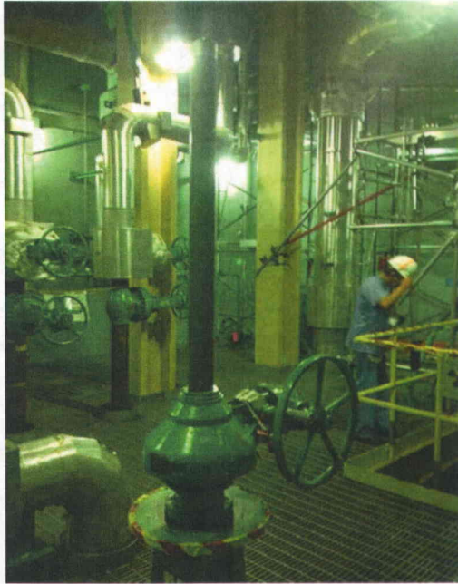
File Name: 2-63-1-4-19.jpeg Description: General view of component
