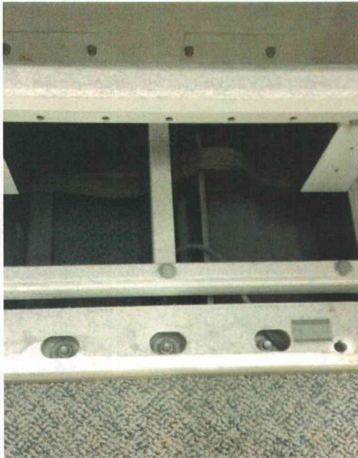
File Name: 2-61-1-4-03.jpeg Description: Anchorage view
