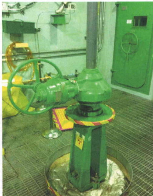
File Name: 2-62-1-4-19.jpeg Description: General view of component
