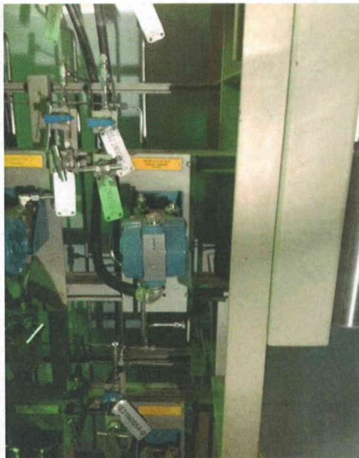
File Name: 2-62-7-4-18.jpeg Description: General view of Component
