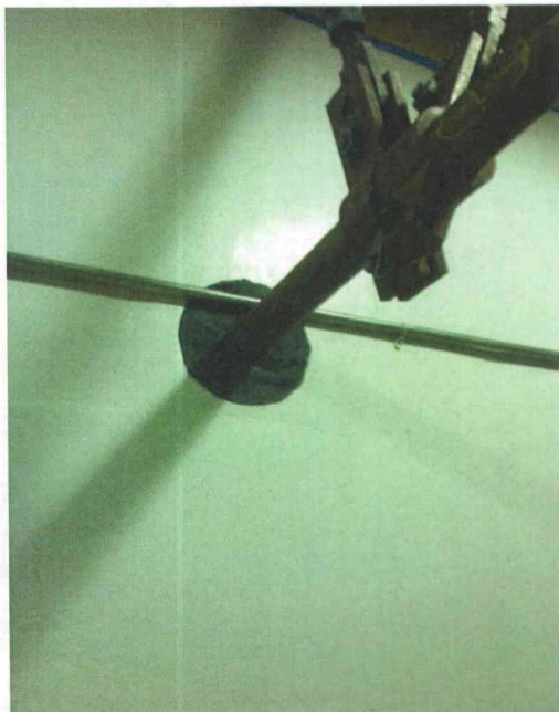
File Name: 2-64-8-4-01.jpeg Description: View of insulation material in concrete wall
