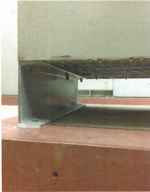
File Name: 2-73-6-1-06.jpeg Description: View of base anchorage detail
