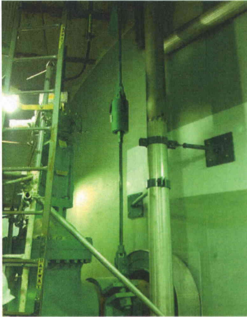
File Name: 2-73-8-4-18.jpeg Description: View vertical support for main line
