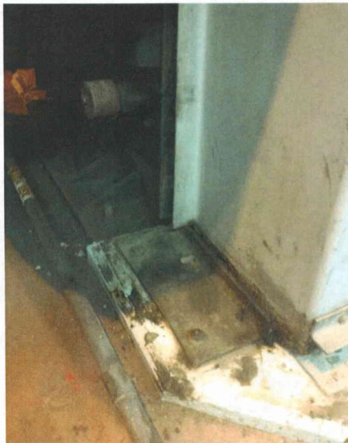
File Name: 2-64-2-4-05.jpeg Description: Anchorage view of component
