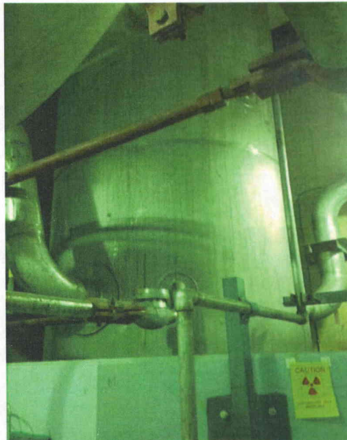
File Name: 2-62-1-4-22.jpeg Description: General view of component
