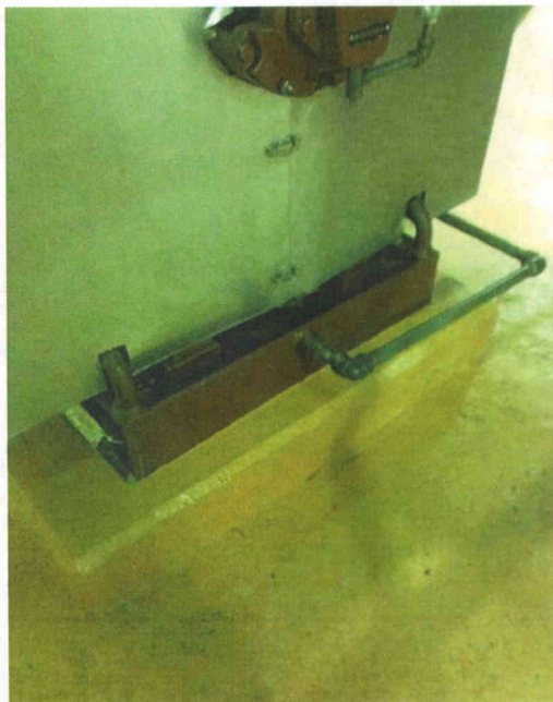
File Name: 2-64-5-4-01.jpeg Description: View of attached lines at component base
