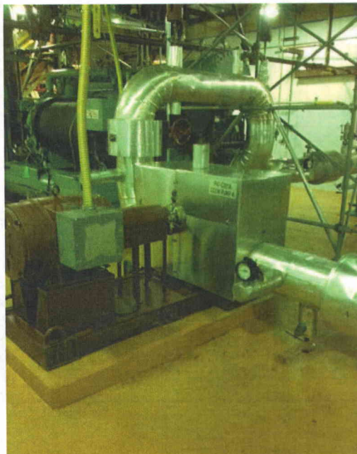
File Name: 2-62-5-4-01.jpeg Description: General view of component
