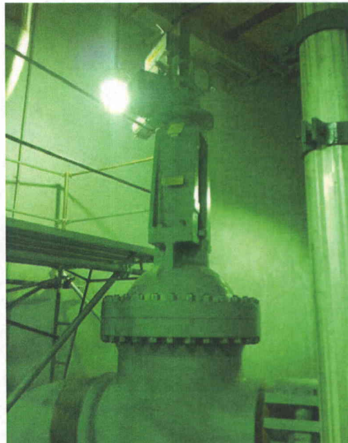
File Name: 2-62-8-4-18.jpeg Description: General view of Component
