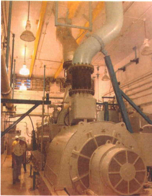
File Name: 2-63-12-4-08.jpeg Description: View of top conduits
