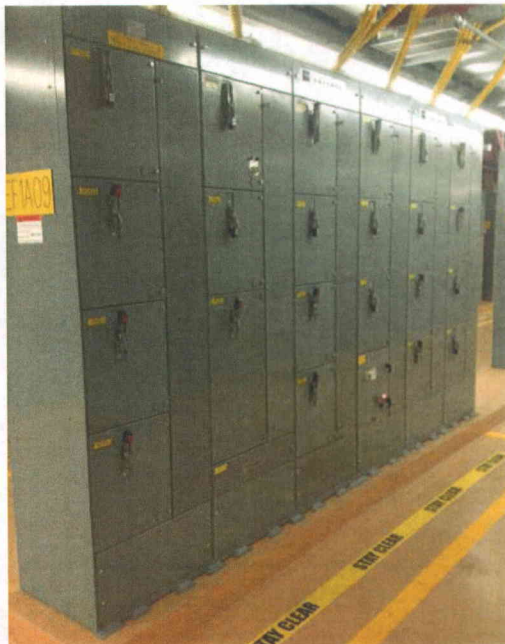
File Name: 2-62-11-4-06.jpeg Description: General view of component
