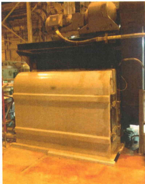
File Name: 2-62-2-4-05.jpeg Description: General view of component
