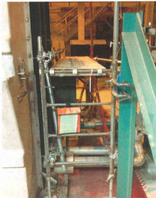
File Name: 2-94-2-4-05.jpeg Description: Scaffold located near component
