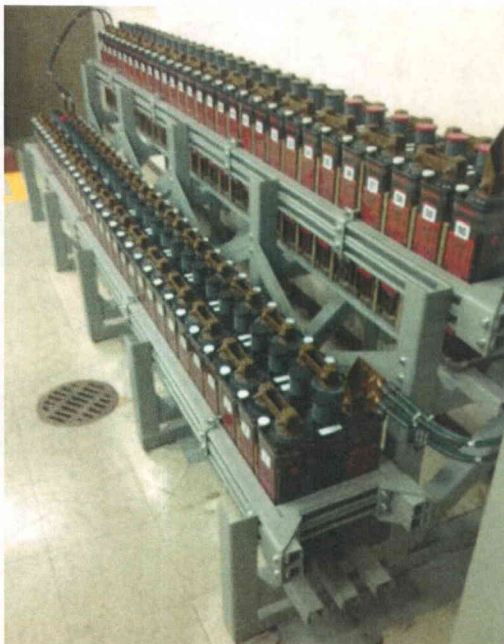
File Name: 2-62-5-4-06.jpeg Description: General view of Component
