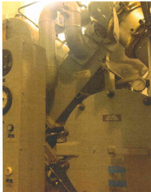
File Name: 2-62-13-4-08.jpeg Description: General view of Component
