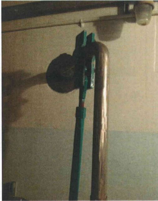
File Name: 2-73-1-4-17.jpeg Description: View of pipe line support
