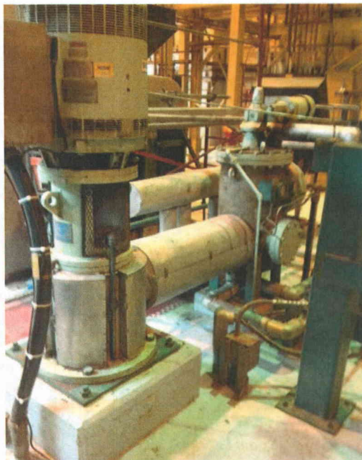
File Name: 2-62-6-1-05.jpeg Description: General view of component
