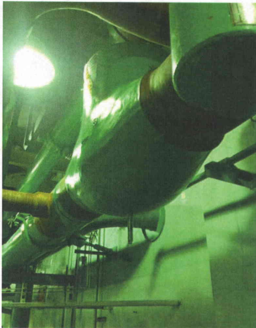
File Name: 2-62-13-4-18.jpeg Description: General view of Component
