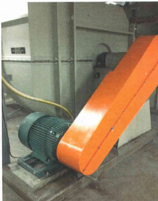
File Name: 2-64-3-4-04.jpeg Description: General view of Component
