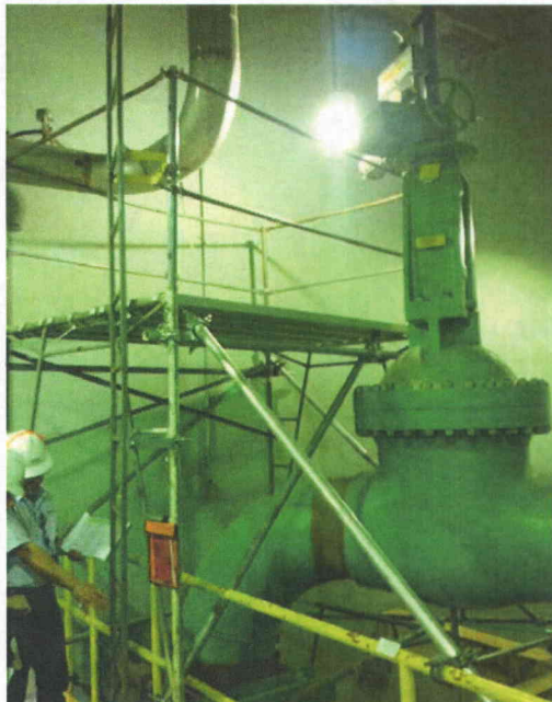
File Name: 2-64-8-4-18.jpeg Description: Scaffolding located in the area
