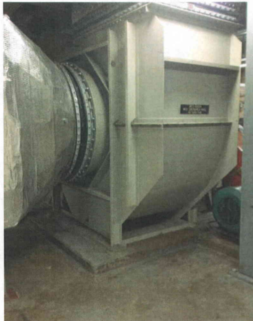
File Name: 2-62-3-4-04.jpeg Description: General view of Component
