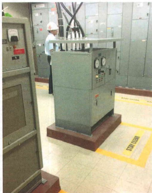
File Name: 2-63-6-1-06.jpeg Description: General view of component
