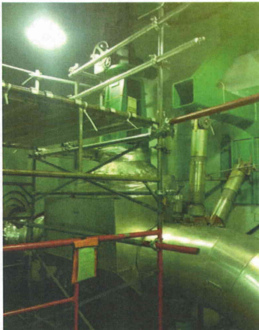
File Name: 2-62-4-4-19.jpeg Description: General view of component
