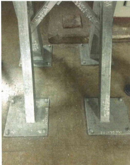
File Name: 2-64-1-4-04.jpeg Description: General view of anchorage
