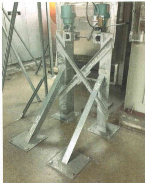
File Name: 2-62-1-4-04.jpeg Description: General view of Component
