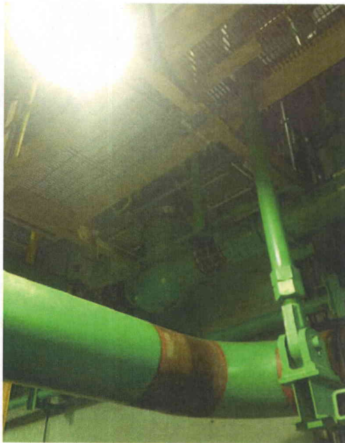
File Name: 2-62-12-4-18.jpeg Description: General view of Component
