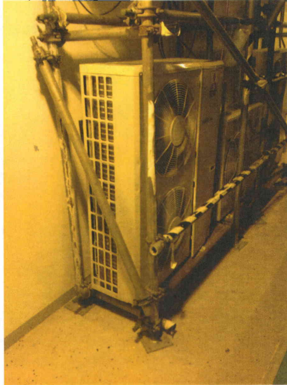
Figure 6-8: View of scaffolding structure for chiller unit
