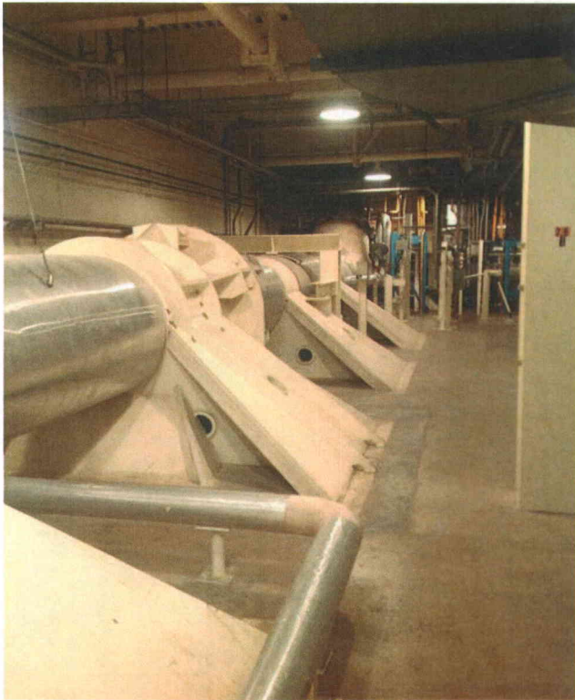
Photo 1 General View of Room 601
