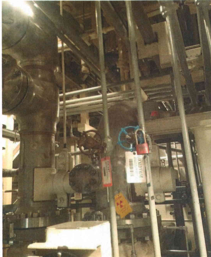
Photo 1 General View of Room 105 Area
