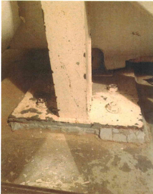
Photo 1 Damaged Grout
