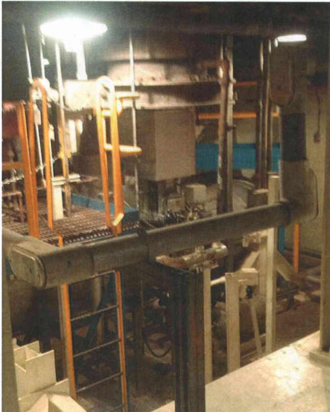
Photo 1 General View of Room 602
