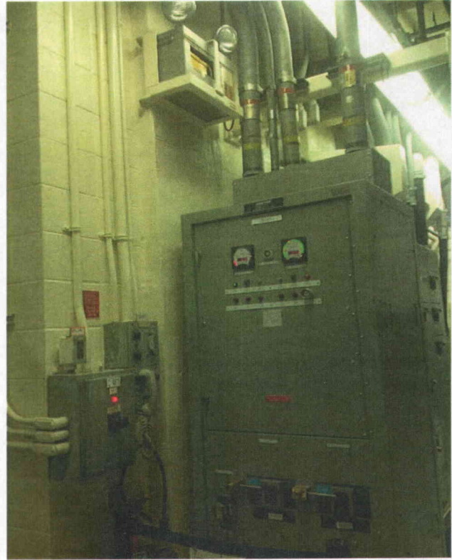
Photo 2 Masonry Wall Adjacent to Components
