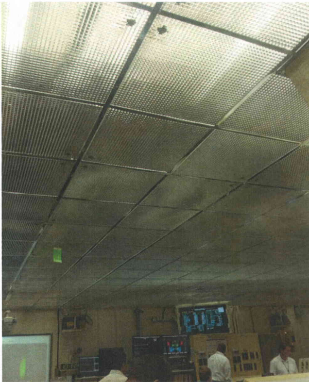
Photo 1 Ceiling Tiles and Lighting Fixtures Anchored
