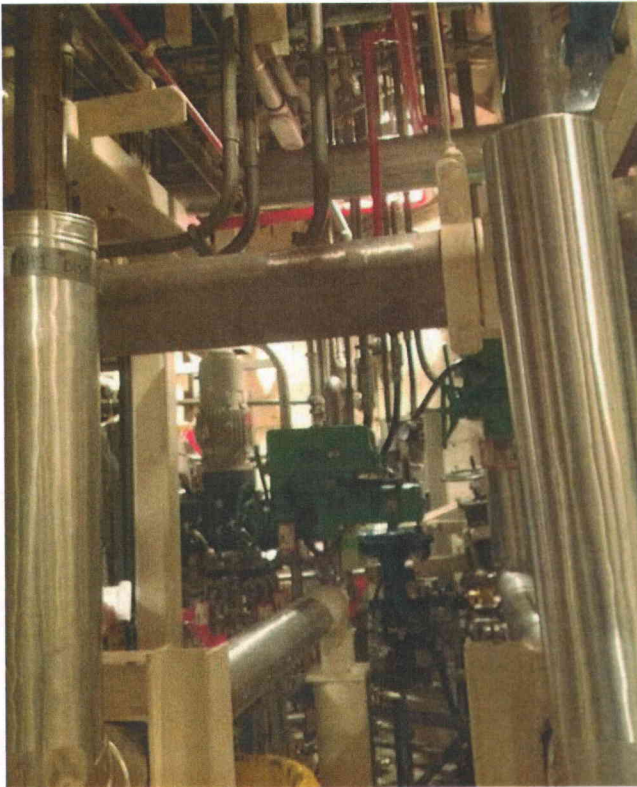
Photo 1 General View of Room 236
