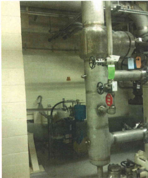
Photo 1 General View of Room 312 Showing Masonry Walls
