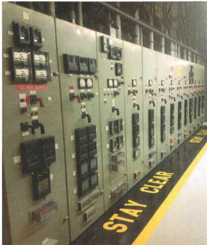
General View of Room 325
