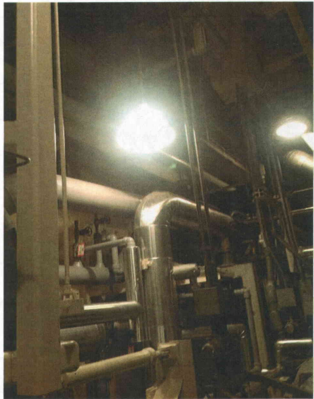
Photo 2 General View of Room 237
