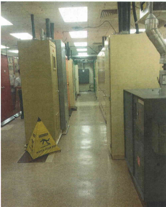
Photo 1 General View of Room 502
