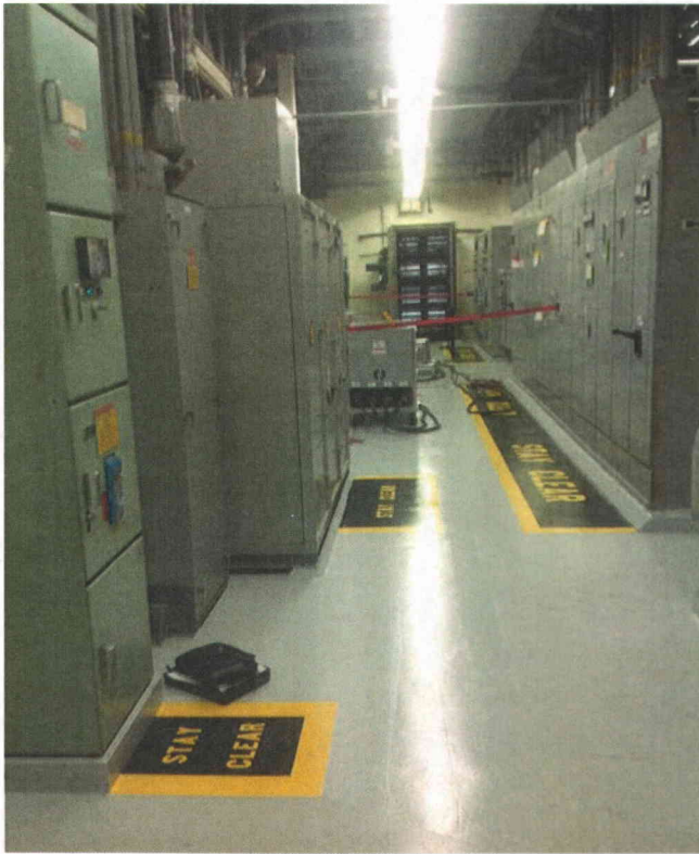
Photo 1 General View of Room 428
