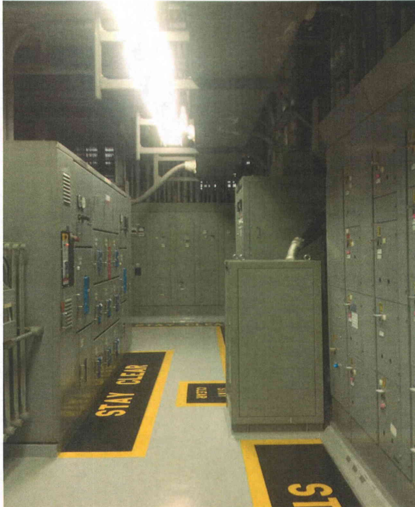
General View of Room 429
