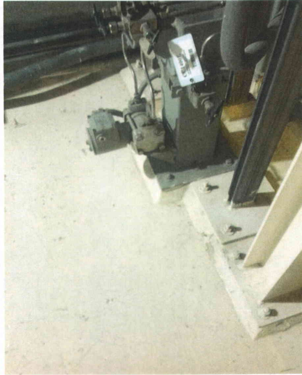
Photo 1 Damaged Grout
