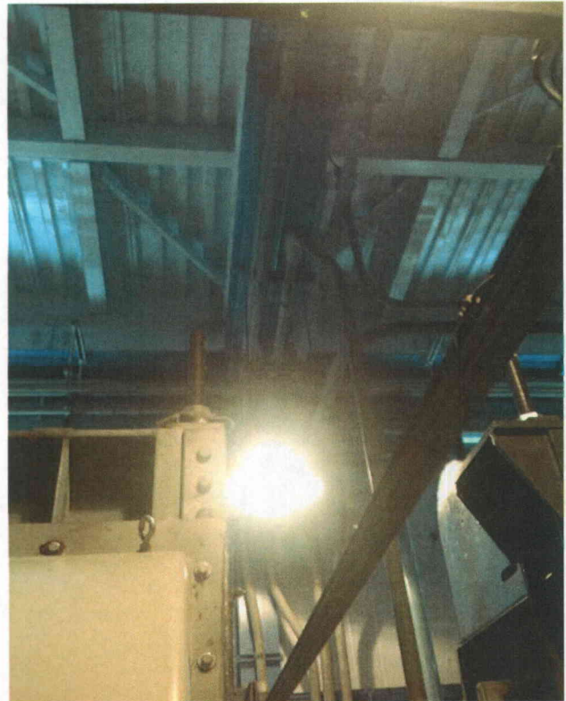
Photo 2 Rod Hung Pipes
