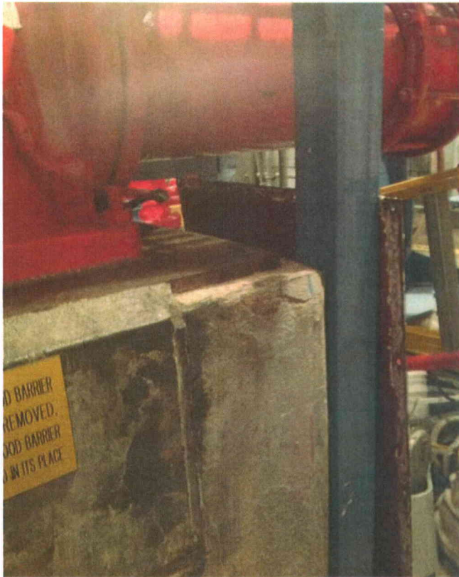
Photo 1 Damaged Grout
