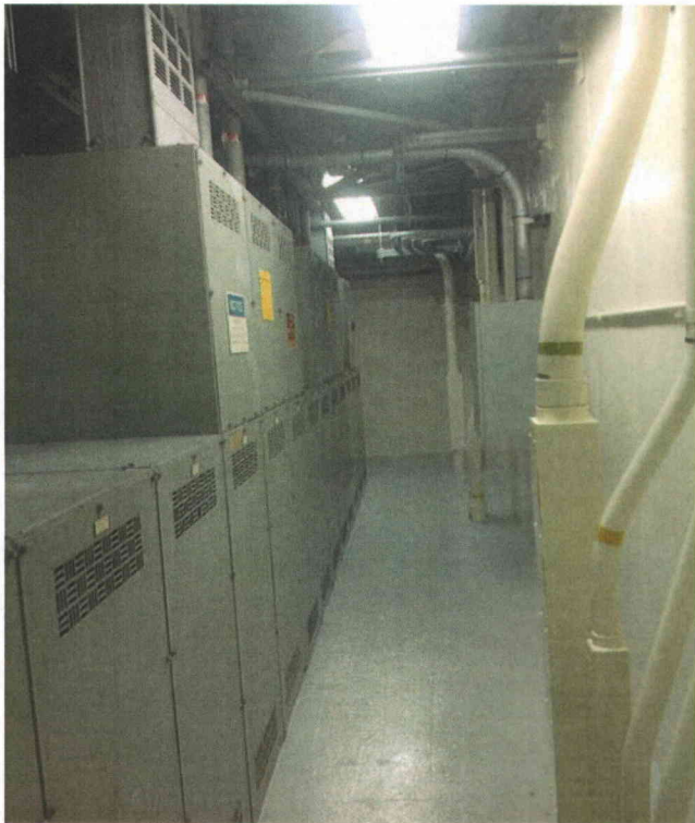
Photo 1 General View of Room 323
