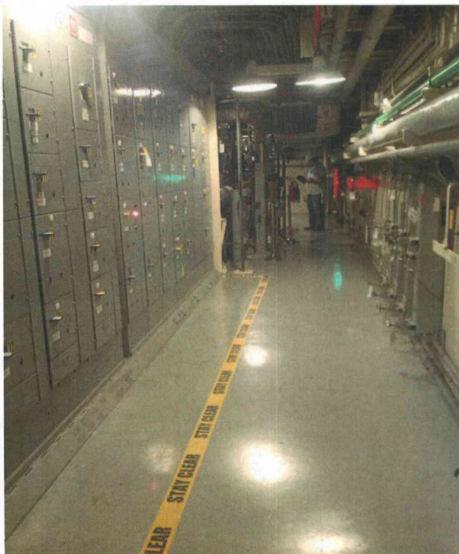
Photo 1 General View of Room 209
