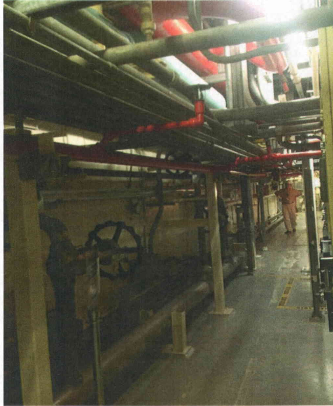
General View of Room 304
