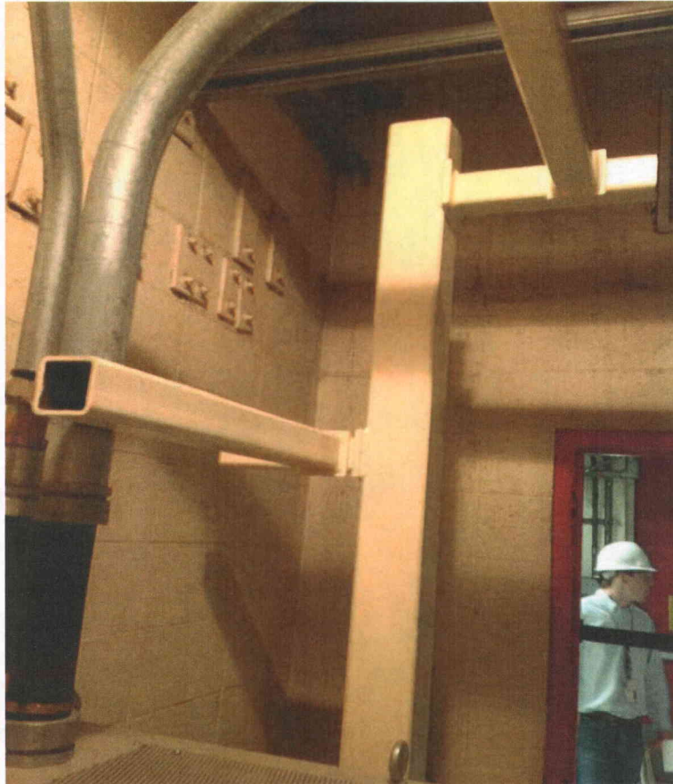
General View of Room 428B
