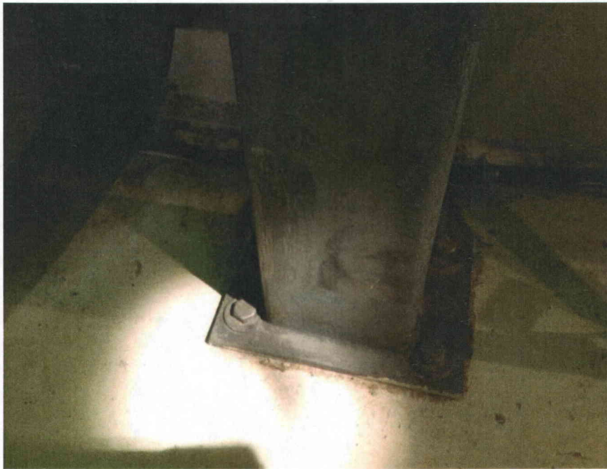
HV5314 anchorage View of anchorage
