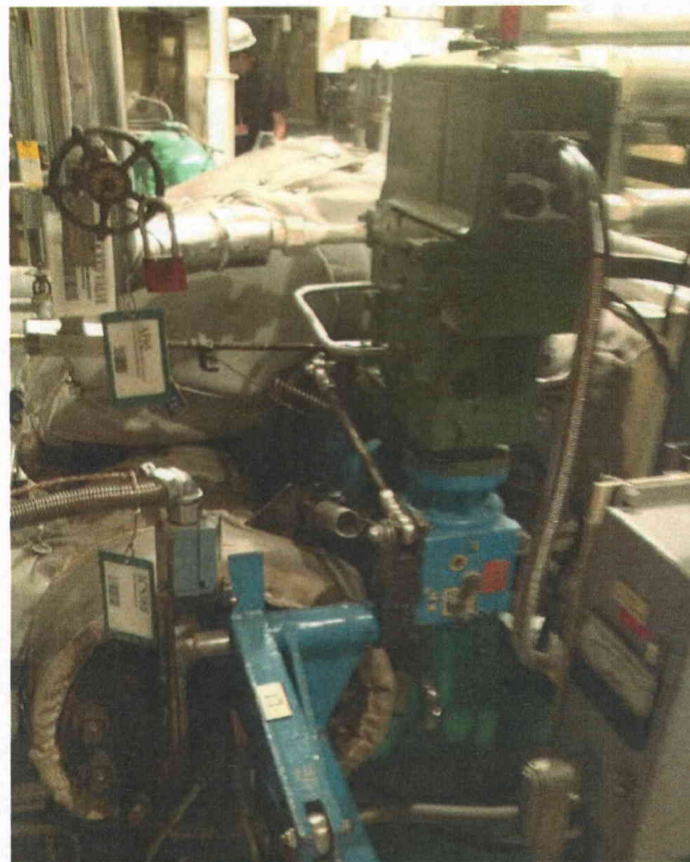
P14-1 general General view of component
