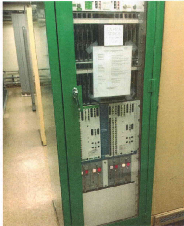
SP9B9-073 General view of component
