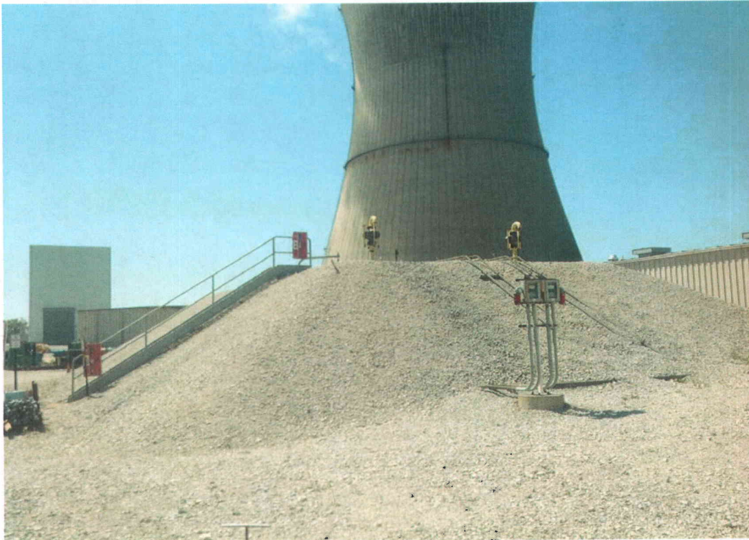
T153-1 General General View of Component
