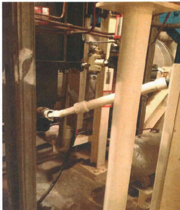
ICS11A brace Brace support for component
