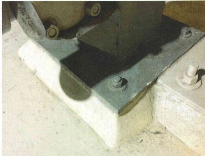
LT1402 anchorage View of anchorage
