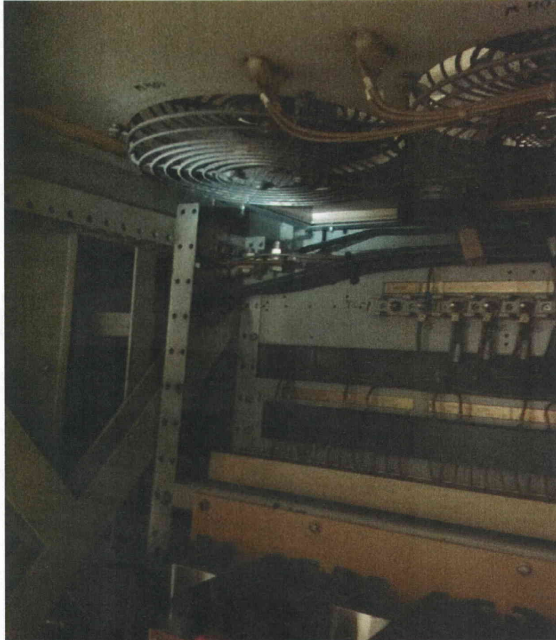
YRF1 open connected to D1P Corresponding train 1 component opened to view internal bolting
