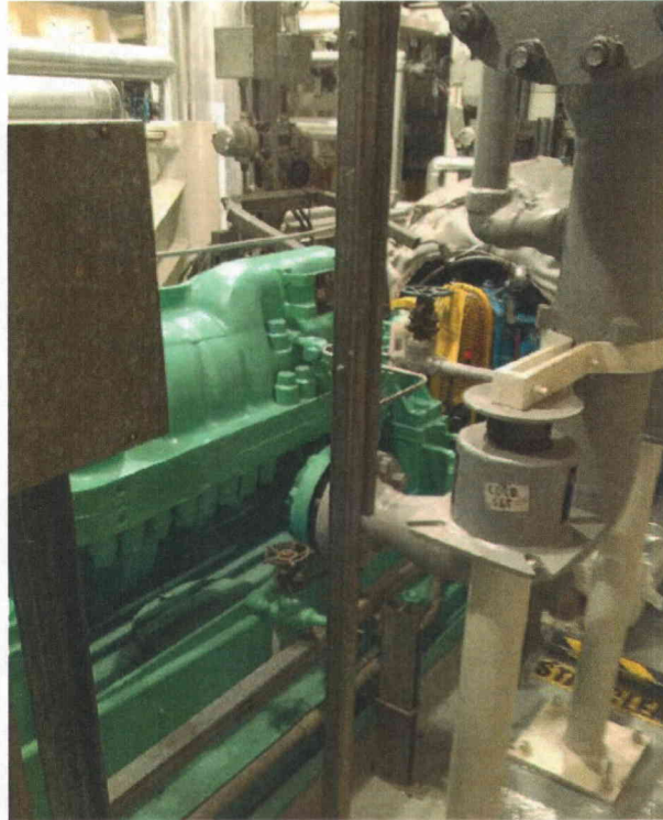
P14-1 general4 General view of component
