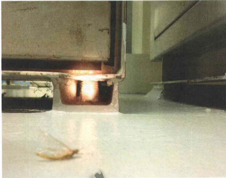
Y2 anchorage Partial view of anchorage, view is typical of all anchors
