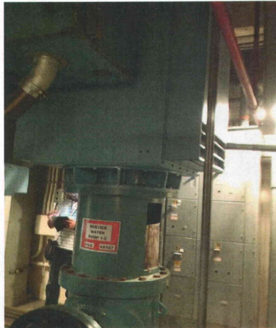
P3-2 general General view of component
