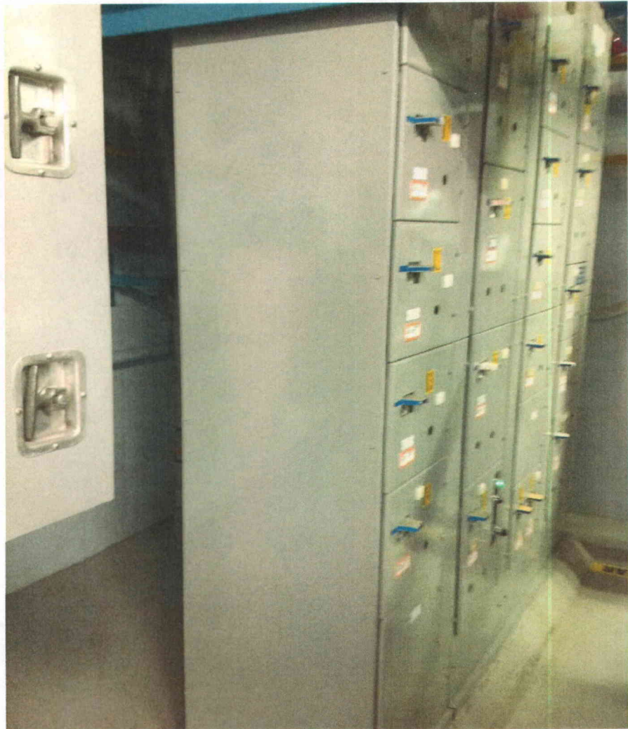
YF1 General General view of component
