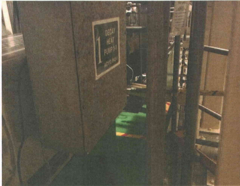
P42-1 general2 General view of component
