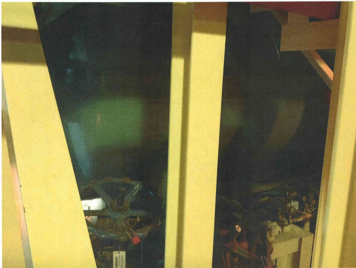
T12 general General view of component
