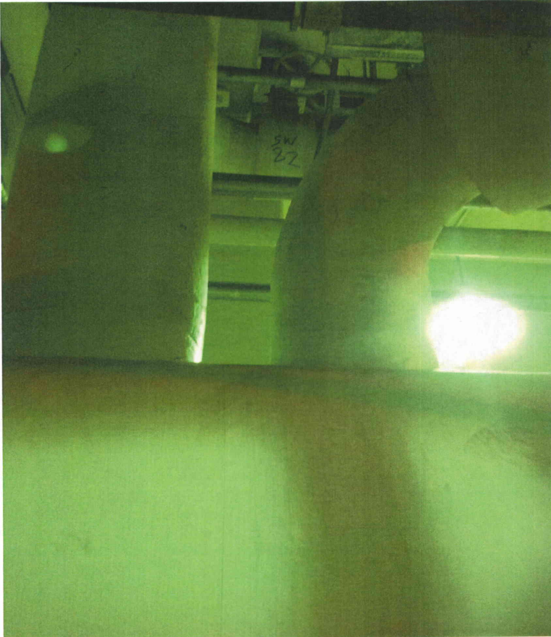
SW82 Plate and General Overall view of component
