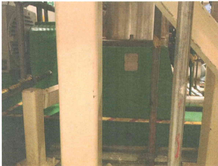
P42-1 general General view of component
