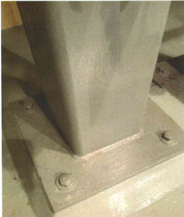
PSL 4928A anchorage View of anchorage
