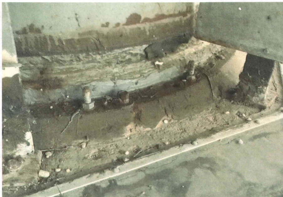
F108-1 Encasing Anchorage View of Intake encasing anchorage condition.
