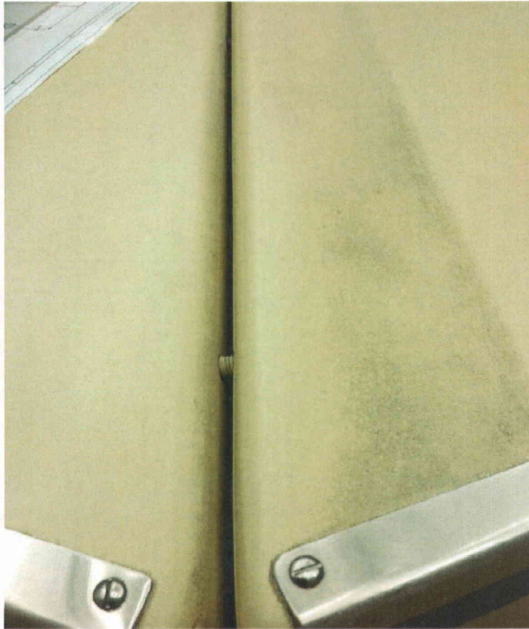
C5706 bolted to left and right sides Cabinets are bolted together on both sides
