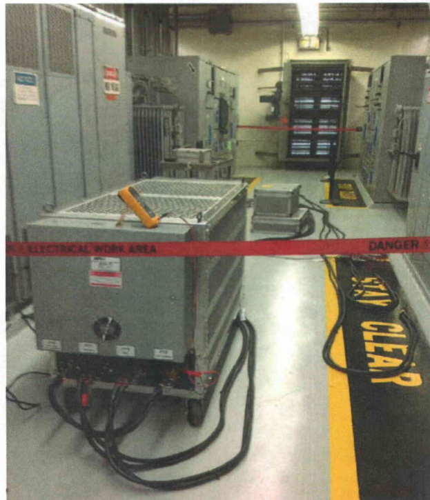
D2 ED carts int Unsecured carts near unit can cause relay chatter on impact
