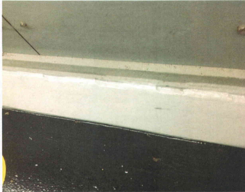
D2 ED stitch weld Partial view of anchorage, view is typical of all anchors
