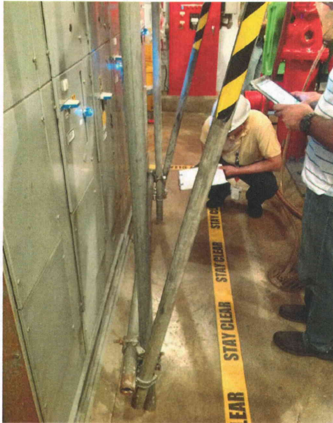
E12C Scaffold View of scaffolding near component
