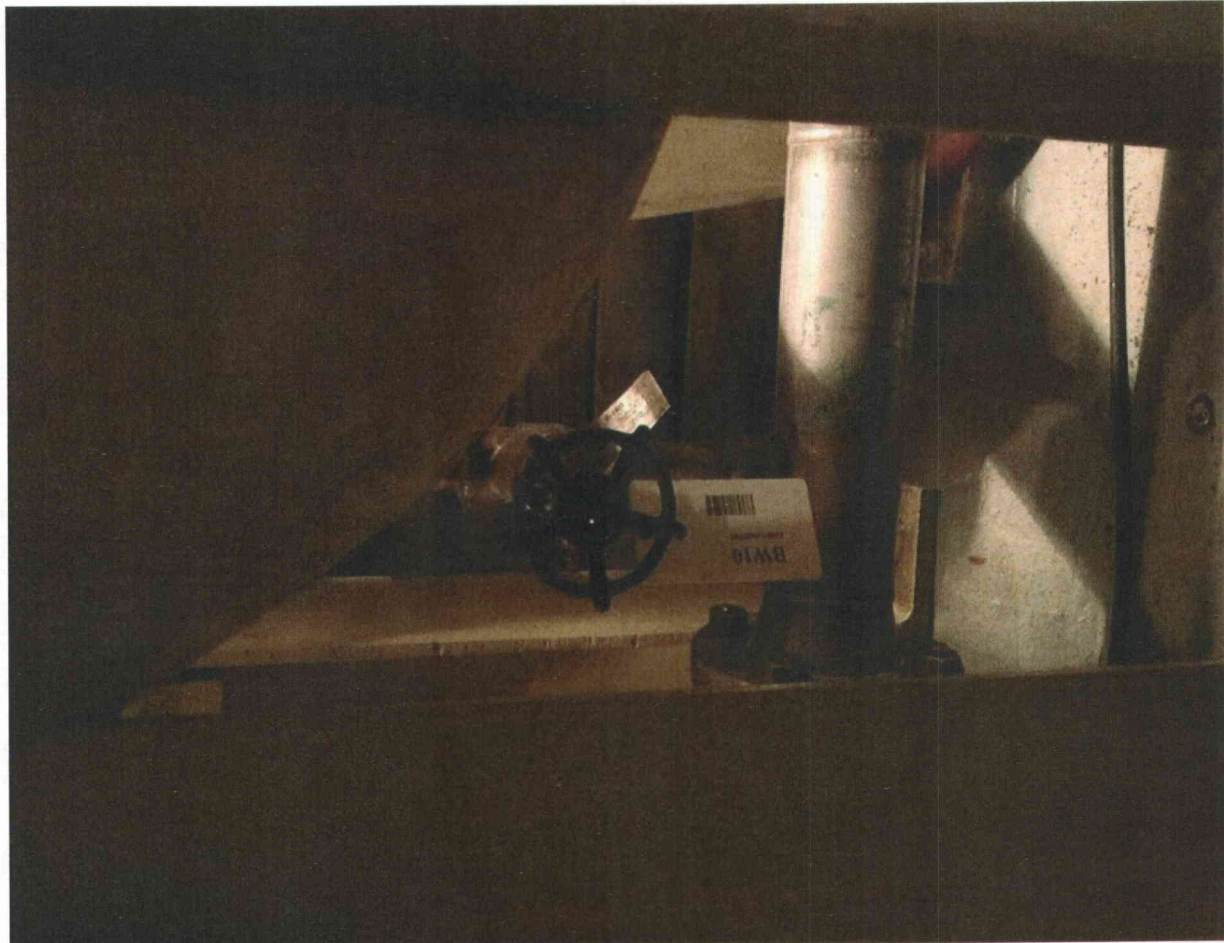
BW10 Plate and General ID plate and general view of component
