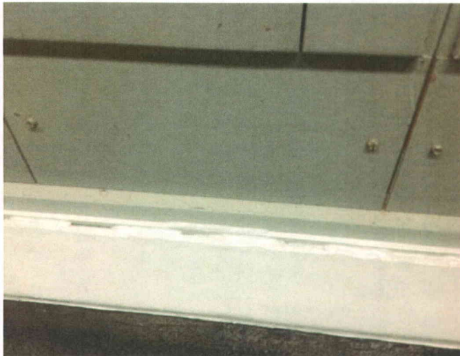
D1_ED stitch weld Partial view of welded base detail.
