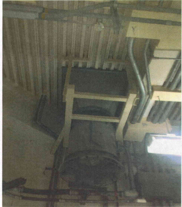
FD1062 anchorage View of anchorage
