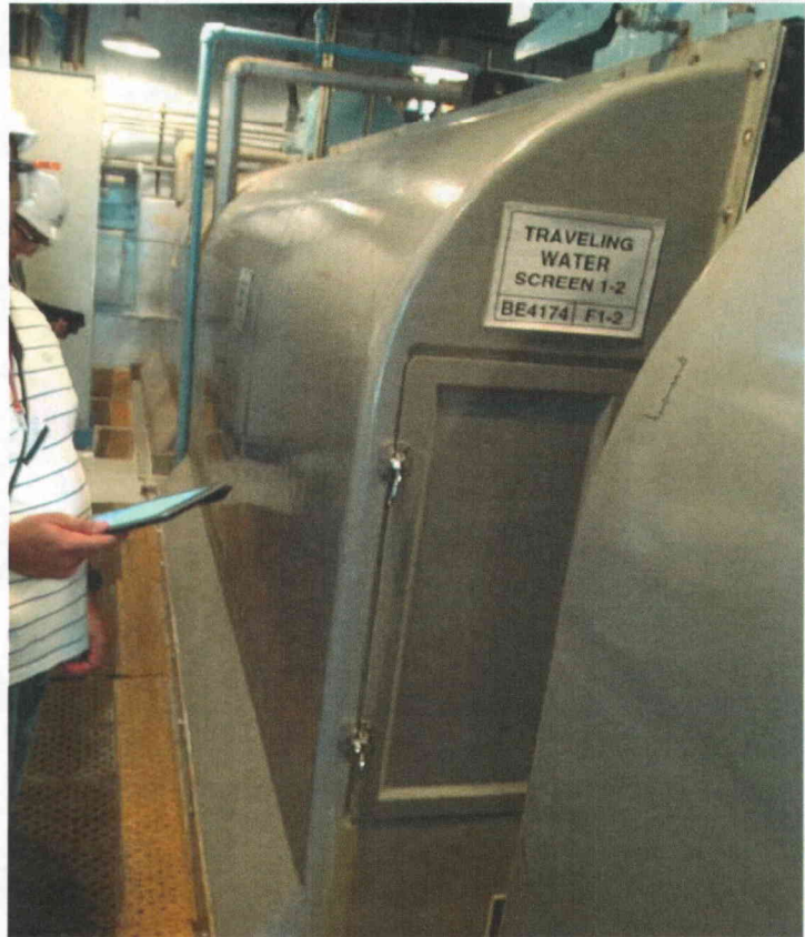
F1-2 general General view of component
