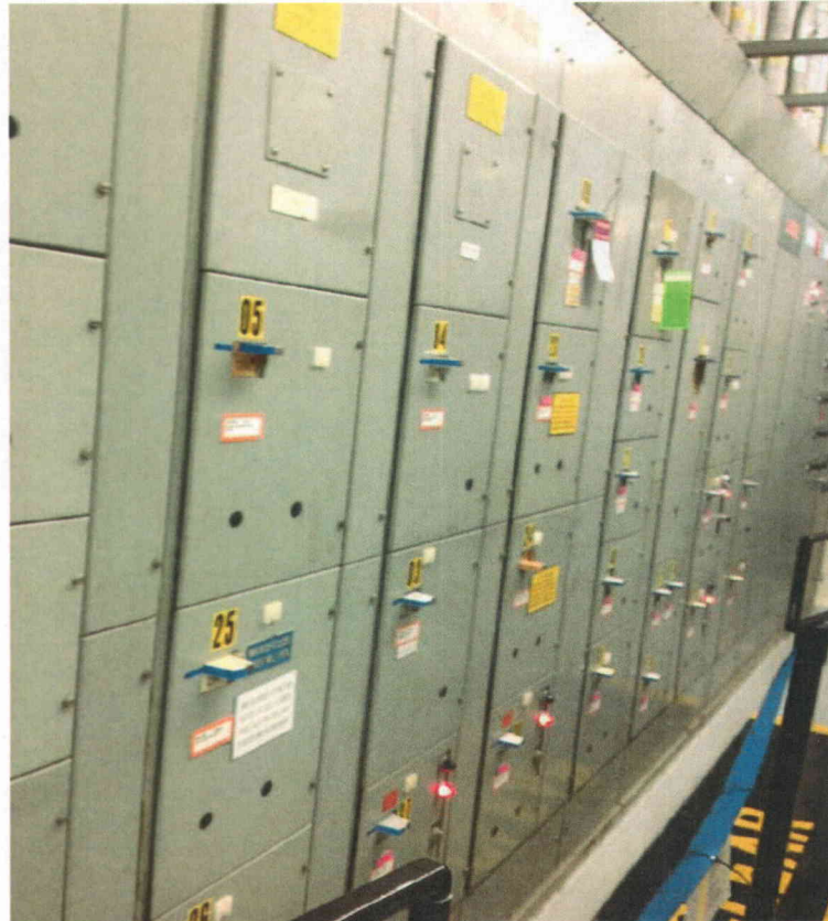
F12A general General view of component
