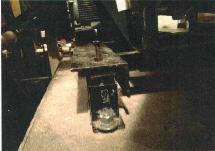
C21-1 anchorage typical View of anchorage
