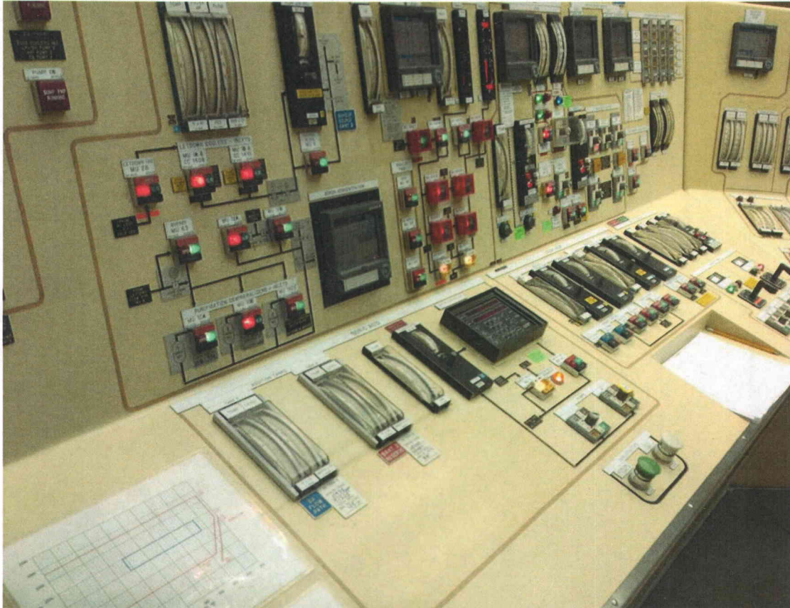
C5702 General view of component
