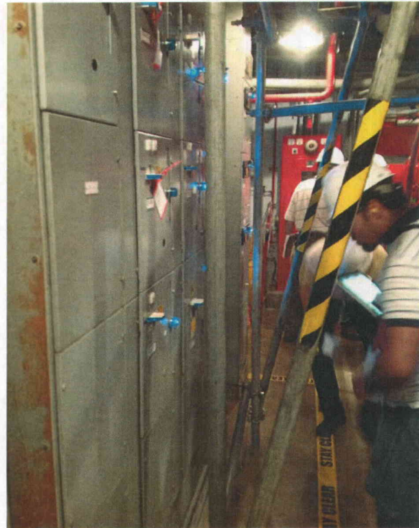
E12C general General view of component
