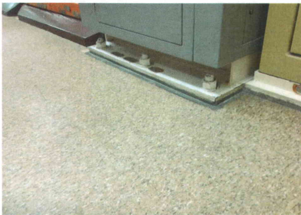
C5755 anchorage General view of anchorage detail
