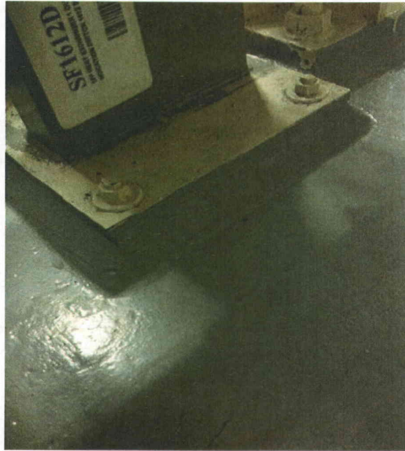
FIS1612 anchorage View of anchorage
