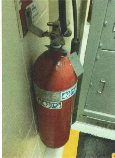
Figure 6-5: Typical Wall Mounting for Fire Extinguishers
