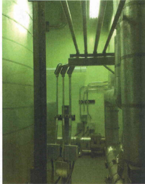
File Name: 1-59-4-3-04.jpeg Description: General view of Boric Acid Tank Room
