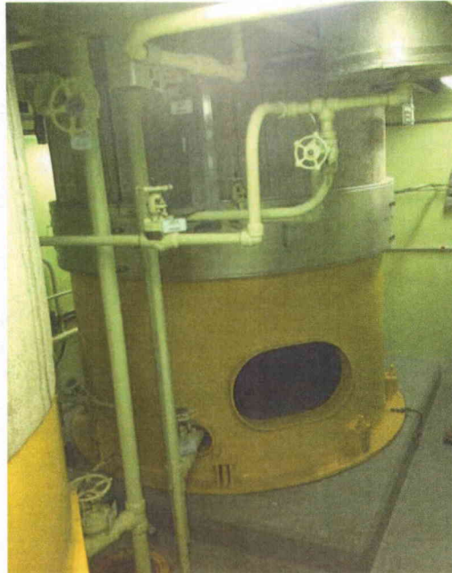
File Name: 1-65-2-3-05.jpeg Description: General view of Surge Tank
