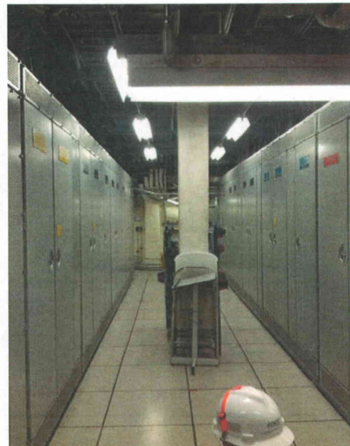
File Name: 1-60-4-3-06.jpeg Description: View of maintenance equipment properly tight to center column
