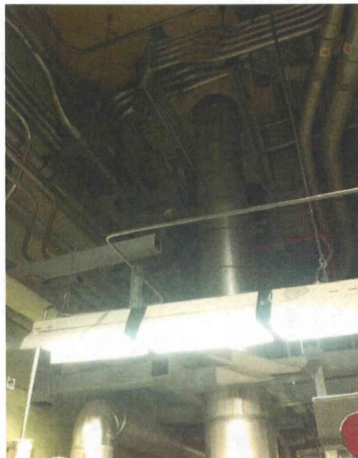
File Name: 1-60-5-3-23.jpeg Description: General view of room's ceiling
