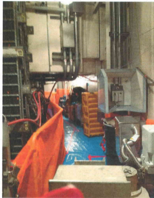
File Name: 1-60-2-3-19.jpeg Description: View of maintenance equipment in the area
