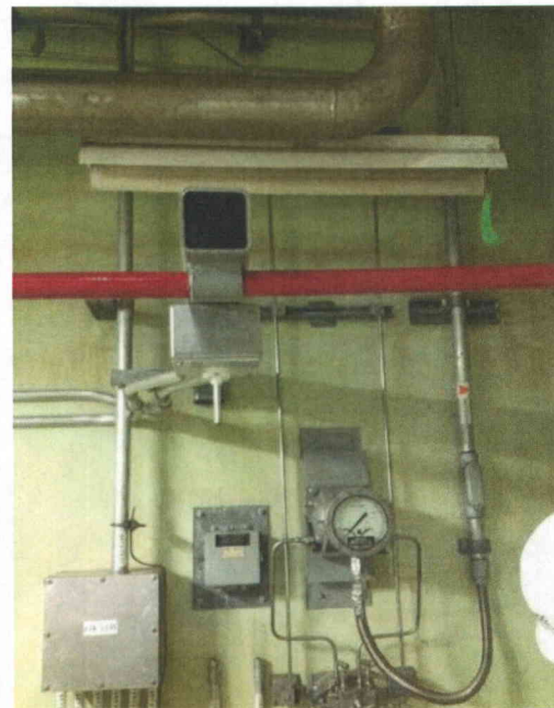
File Name: 1-70-5-3-23.jpeg Description: Potential falling of light bulb could impact instrument below. Judged not a significant interaction.
