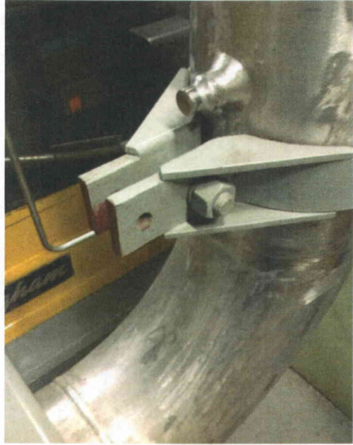
File Name: 1-68-5-4-23.jpeg Description: View of deleted support rod for 2QSS-P21A discharge nozzle.
