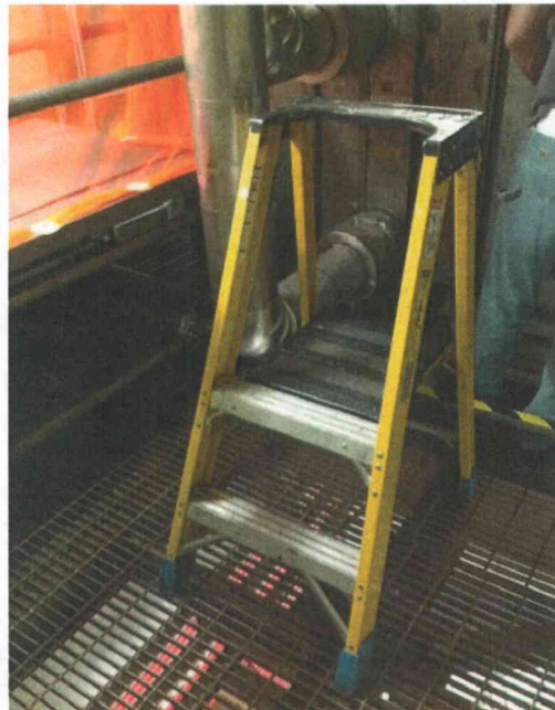
File Name: 1-60-2-3-25.jpeg Description: Unrestrained ladder identified in the area. Judged not a seismic concern for nearby equipment.
