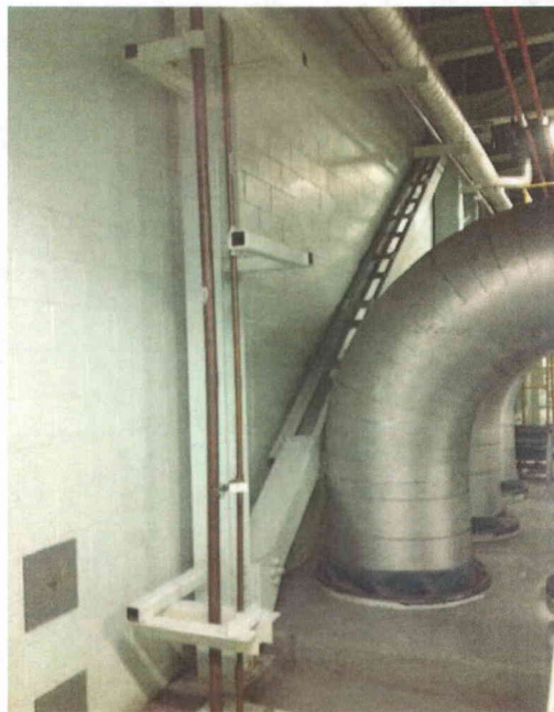
File Name: 1-68-2-3-27.jpeg Description: Block wall identified in the area
