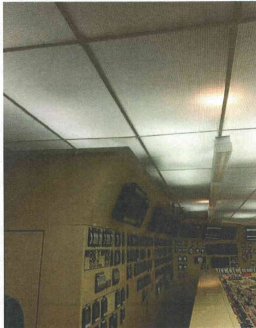
File Name: Control_Rm(6).jpg Description: General view of ceiling grates.
