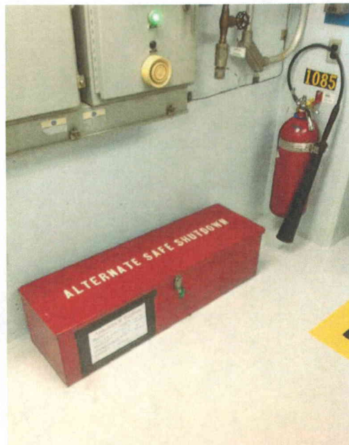
File Name: SWGR AE(4).jpg Description: Storage box located in the area.
