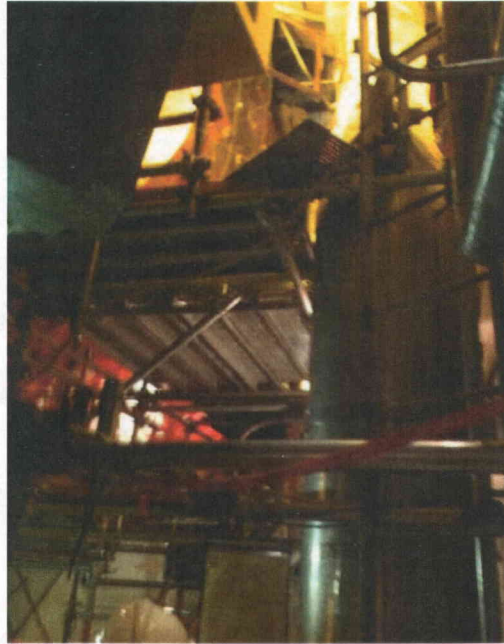
File Name: 1-65-6-3-19.jpeg Description: View of scaffold in the area
