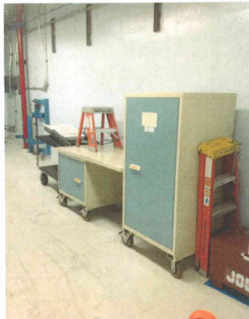
File Name: SWGR_DF(4).jpg Description: Storage carts and ladders located in the area identified to be properly secured.
