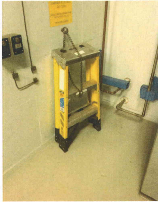
File Name: EDG2-1(7).jpg Description: View of restrained ladder in the area
