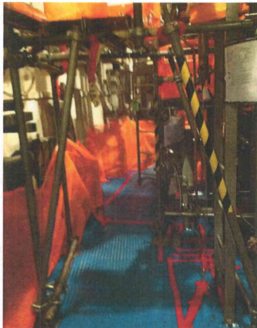
File Name: 1-67-7-3-19.jpeg Description: View of scaffold in the area
