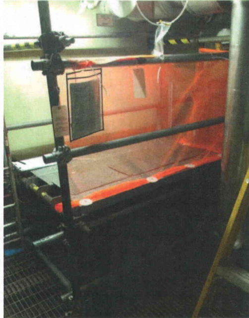
File Name: 1-59-2-3-25.jpeg Description: Scaffold located in the area
