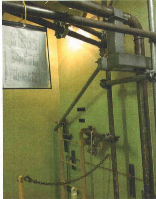
File Name: 1-65-3-3-02.jpeg Description: View of scaffold in the area
