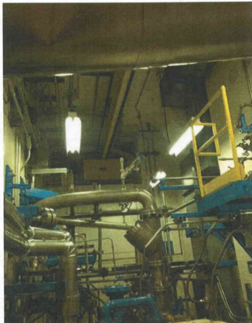
File Name: 1-60-4-3-03.jpeg Description: View of ceiling and lighting fixtures
