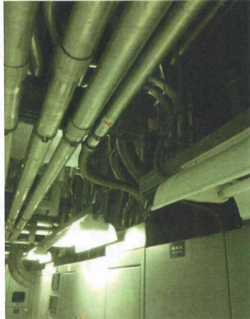
File Name: SWGR AE(7).jpg Description: Hanging light located close to cabinet. Interaction addressed in CR-2012-14463
