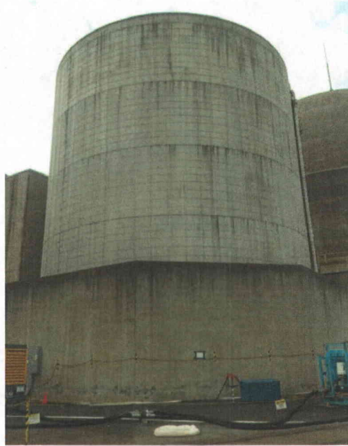
File Name: 1-65-4-3-29.jpeg Description: View of Tank 2QSS-TK21.
