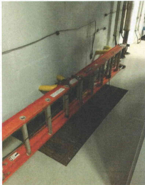
File Name: EDG2-1(8).jpg Description: View of restrained ladder in the area
