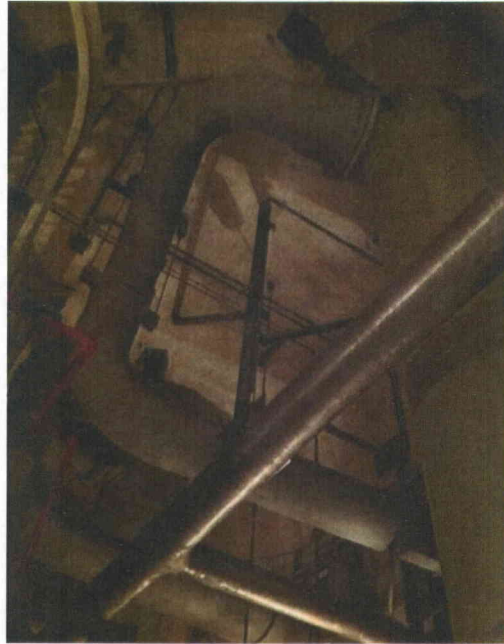
File Name: 2-64-3-2-18.jpeg Description: General view of ceiling rod hung supports
