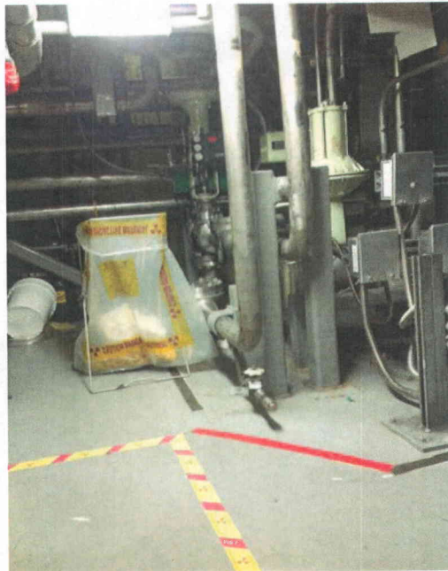
File Name: 1-60-6-3-01.jpeg Description: Area general view
