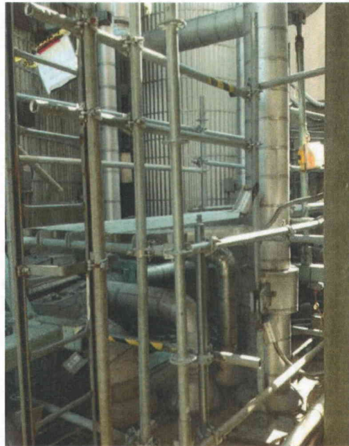
File Name: 1-67-4-3-29.jpeg Description: Scaffold located in the area.
