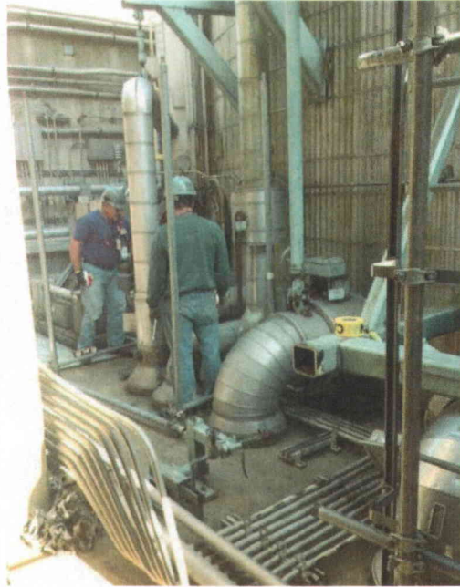
File Name: 1-66-4-3-29.jpeg Description: General view of area
