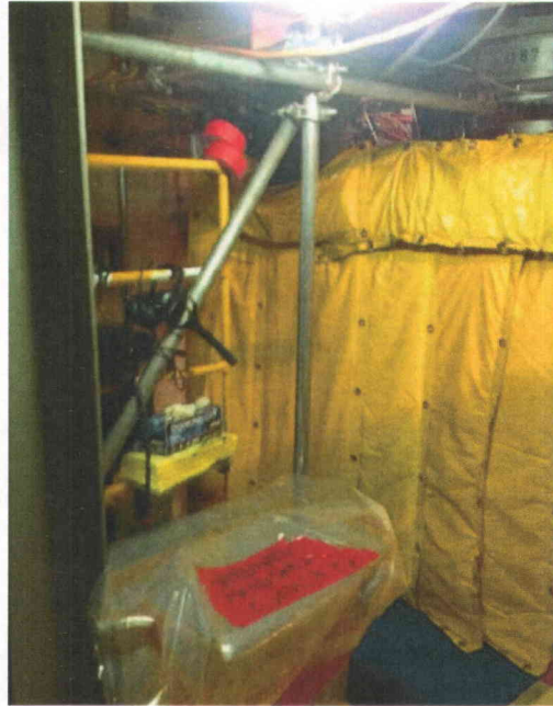
File Name: 1-59-6-3-19.jpeg Description: View of scaffold in the area
