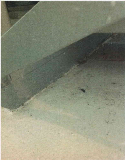
File Name: BAT-2-1(2).jpg Description: View of Anchor Welds
