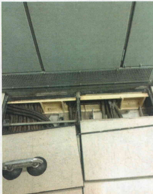
File Name: 2-96-3-2-06.jpeg Description: View of Anchor Welds
