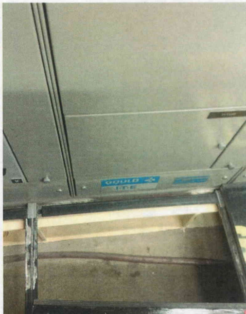
File Name: 2-95-1-2-06.jpeg Description: View of Welds at Component Base
