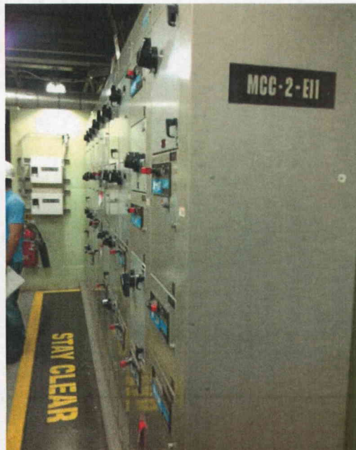
File Name: 2-62-1-2-24.jpeg Description: General View of Component
