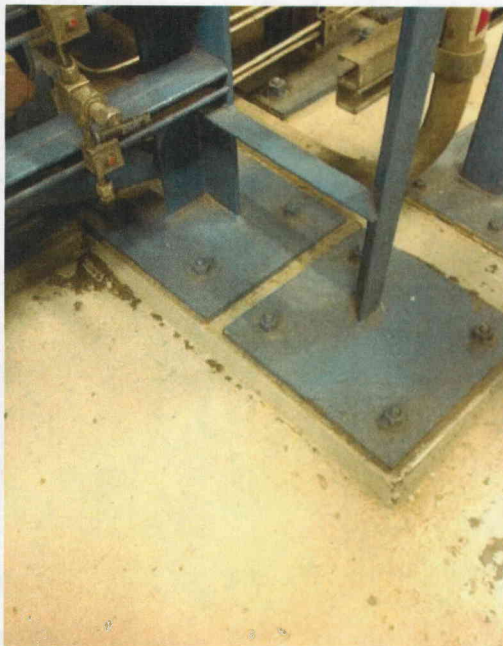
File Name: 2SWS-PT-117A(4).jpg Description: View of Rack Anchorage
