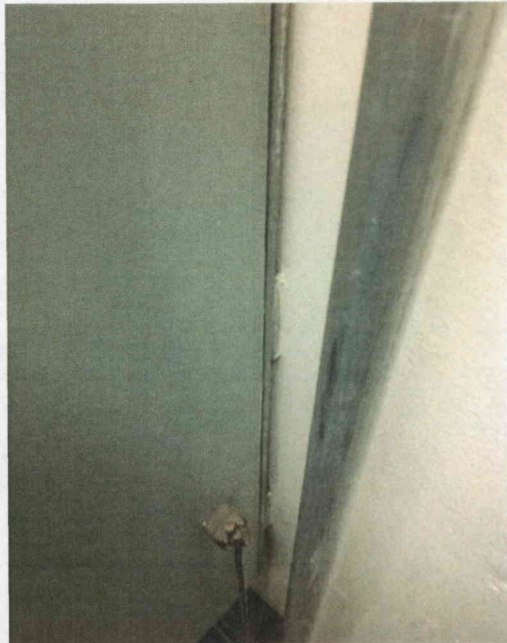
File Name: PNL-VITBS2-2C(4).jpg Description: View of Anchorage to Wall
