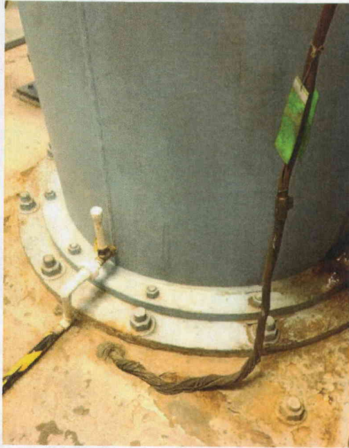
File Name: 2SWS-P21A(3).jpg Description: View of Anchor Bolts
