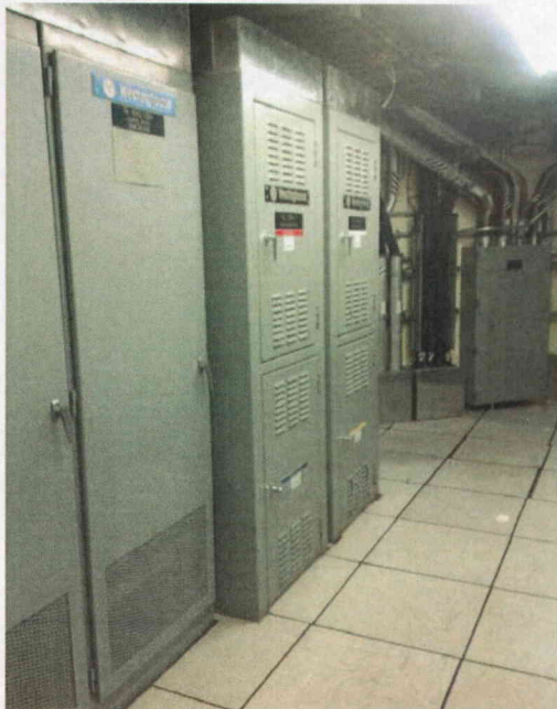
File Name: 2-62-6-2-06.jpeg Description: General View of Component
