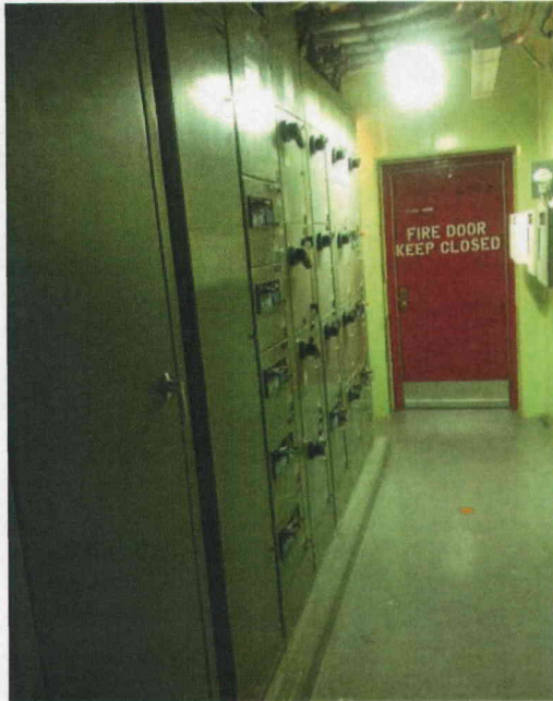
File Name: 2-63-3-2-04.jpeg Description: General View of Component
