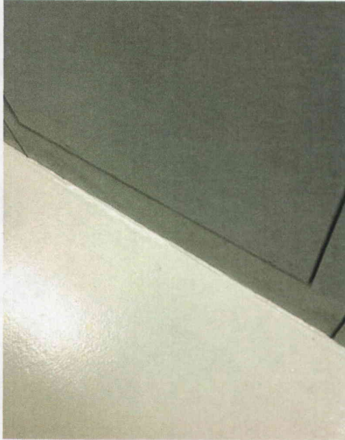
File Name: PNL-SEQ-244(3).jpg Description: View of Anchor Weld
