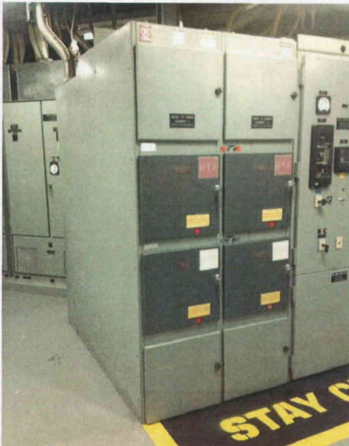
File Name: 2-62-1-2-15.jpeg Description: General View of Component
