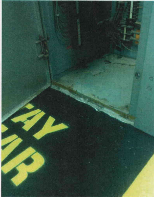
File Name: 2-95-9-2-26.jpeg Description: View of Welds at Component Base
