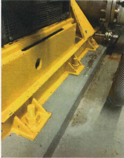
File Name: 2-63-5-2-23.jpeg Description: Close Up View of Anchorage
