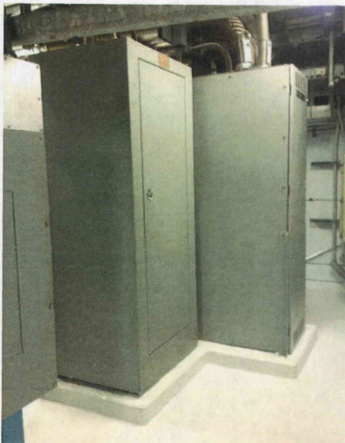
File Name: 2-62-17-2-26.jpeg Description: General View of Component
