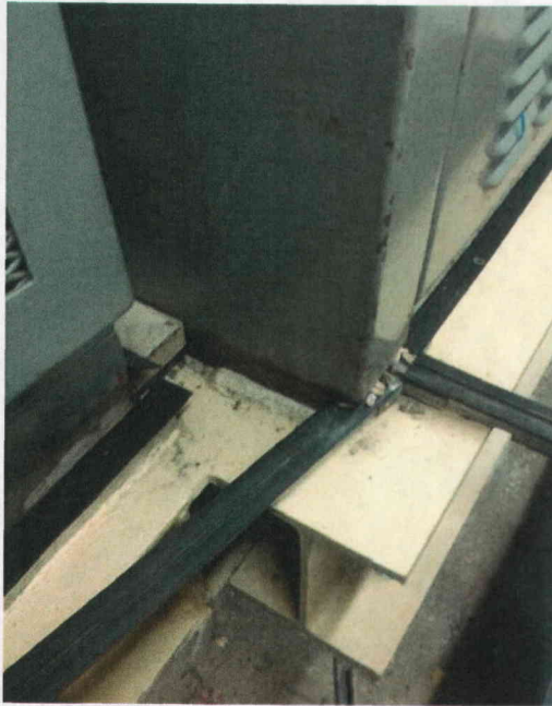
File Name: 2-63-6-2-06.jpeg Description: View of Anchor Welds
