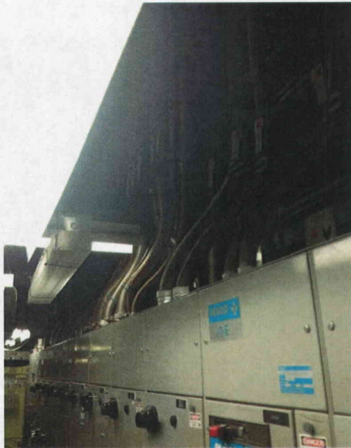
File Name: 2-73-1-2-13.jpeg Description: View of Flexible Top Conduit
