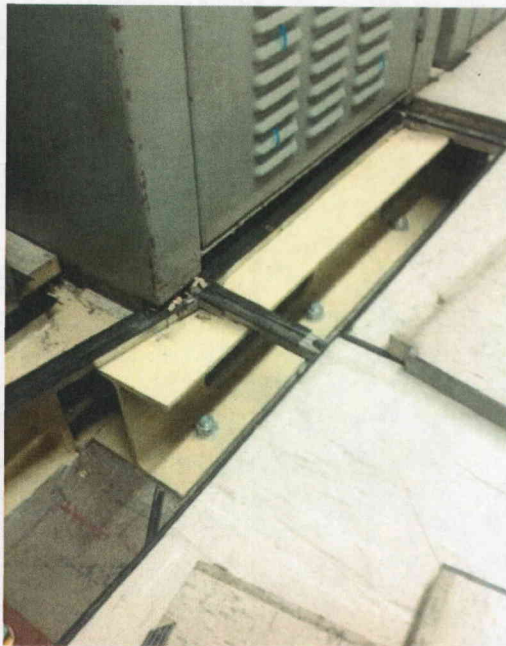
File Name: 2-64-6-2-06.jpeg Description: View of Anchor Welds
