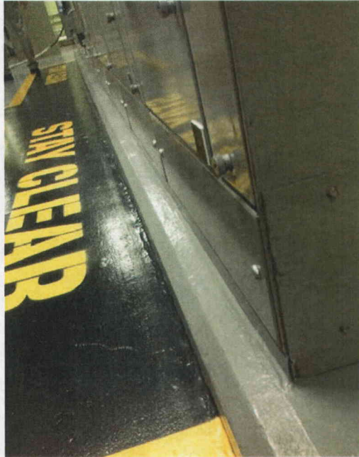
File Name: 2-63-1-2-13.jpeg Description: View of Front Anchorage
