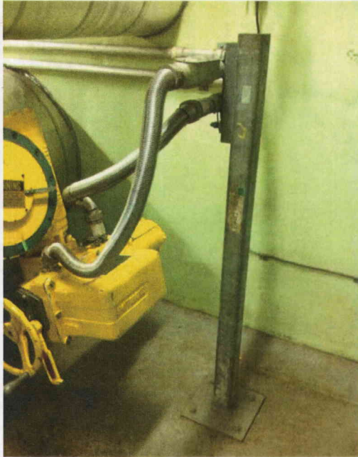
File Name: 2SWS-MOV106A(3).jpg Description: View of Attached Lines
