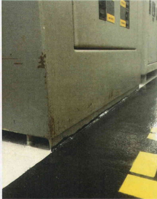
File Name: 2-63-18-2-26.jpeg Description: View of Anchor Weld
