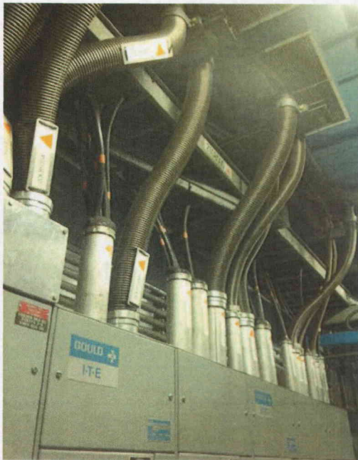
File Name: MCC-2-E07(4).jpg Description: View of Flexible Top Lines
