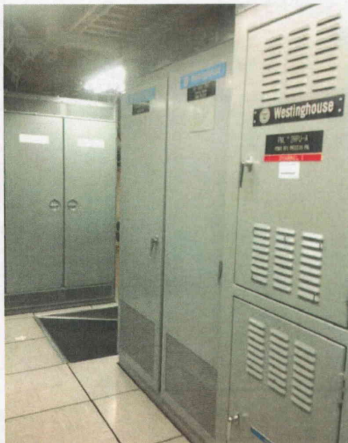
File Name: 2-62-7-2-06.jpeg Description: General View of Component
