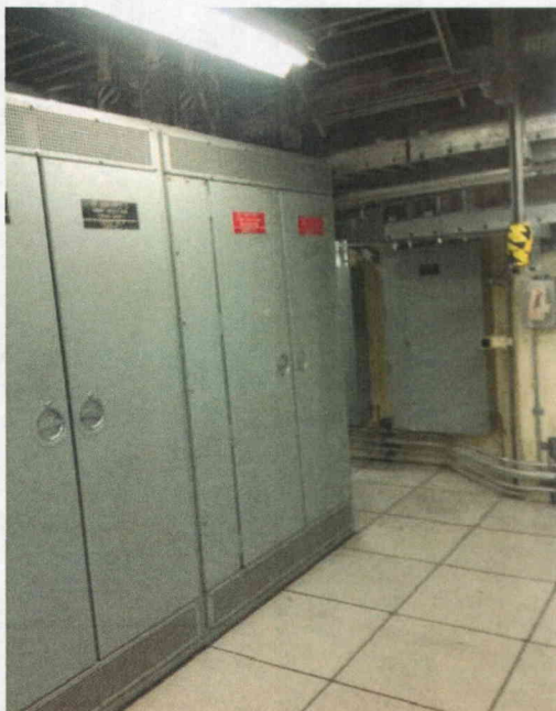
File Name: 2-73-3-2-06.jpeg Description: General View of Component
