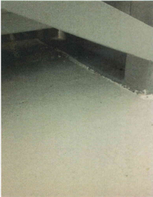
File Name: BAT-2-1(3).jpg Description: View of Anchor Welds
