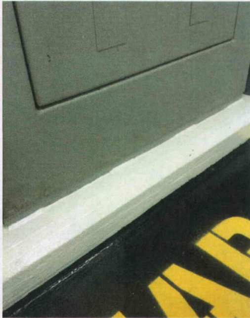
File Name: 2-63-17-2-26.jpeg Description: View of Anchor Welds
