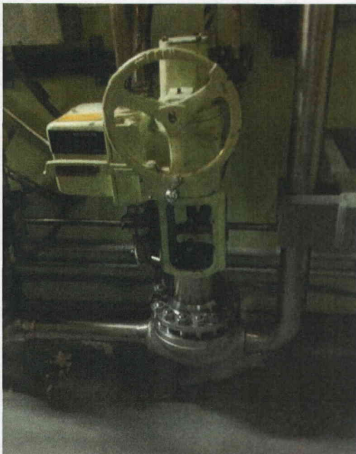
File Name: 2-62-1-2-01.jpeg Description: General View of Component
