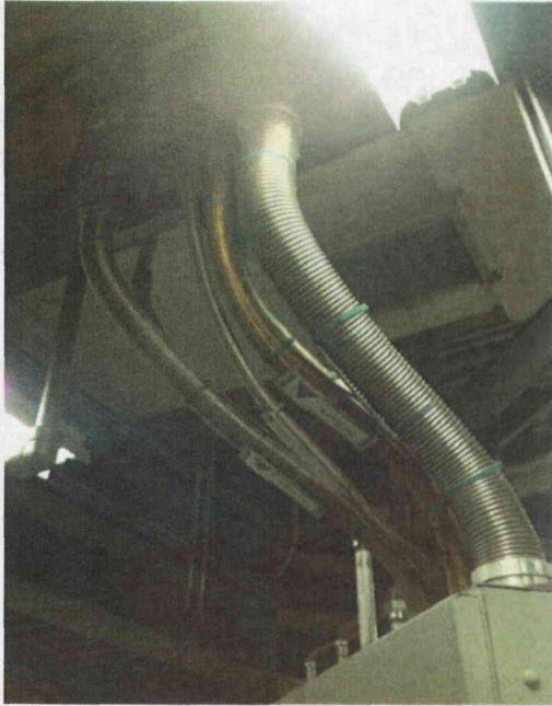
File Name: 2-63-2-2-15.jpeg Description: View of Flexible Top Lines
