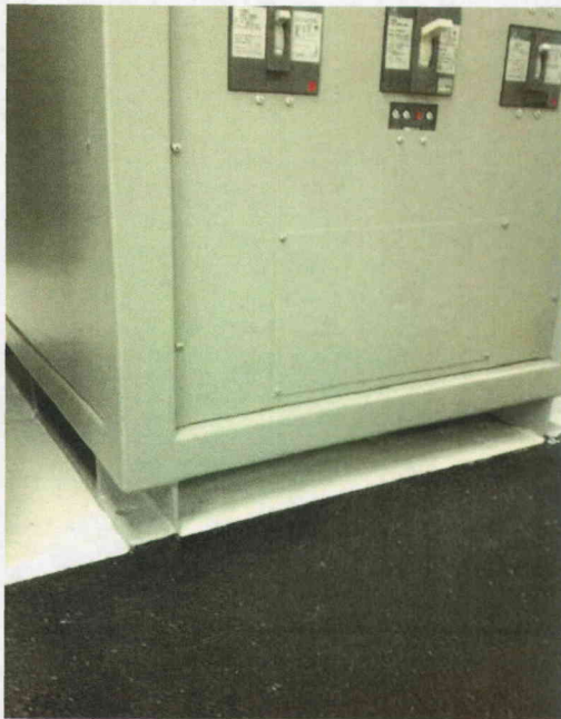
File Name: BAT-CHG2-1(4).jpg Description: View of Welded Channel at Front of Component
