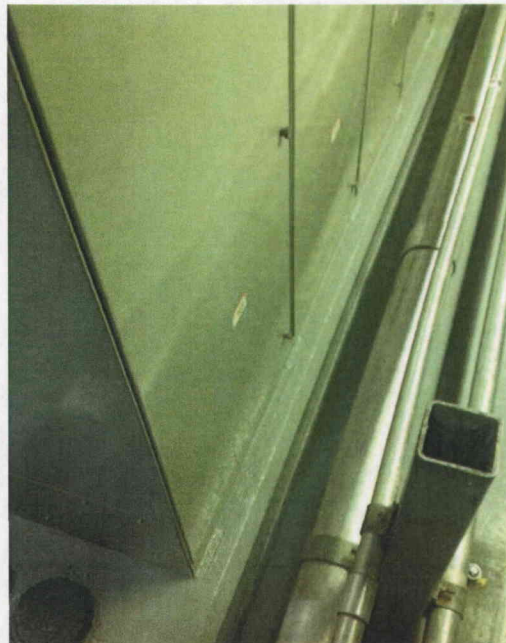
File Name: 2-64-1-2-13.jpeg Description: View of Back Anchorage
