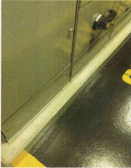
File Name: MCC-2-E07(3).jpg Description: View of Anchor Welds
