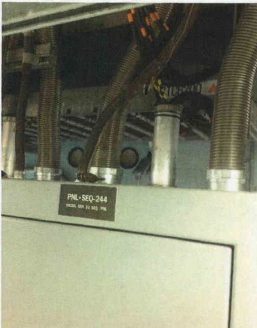
File Name: PNL-SEQ-244(4).jpg Description: View of Flexible Top Lines
