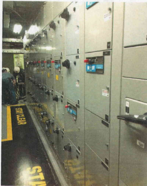
File Name: 2-62-1-2-13.jpeg Description: General View of Component
