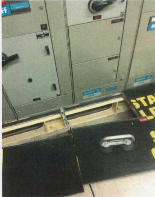
File Name: 2-94-1-2-06.jpeg Description: View of Welds at Component Base
