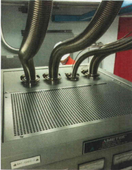
File Name: BAT-CHG2-1(5).jpg Description: View of Flexible Top Lines
