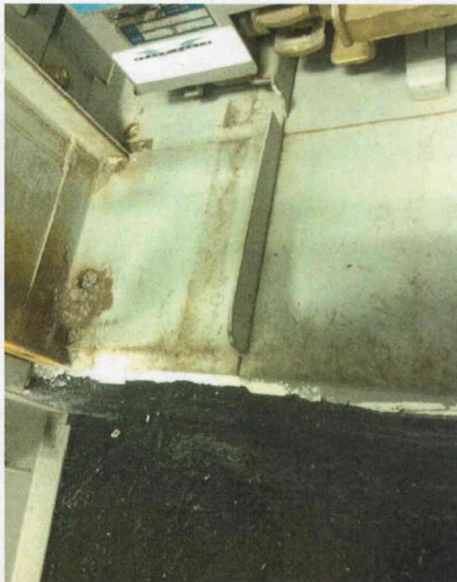
File Name: 2-63-11-2-26.jpeg Description: View of Interior Base
