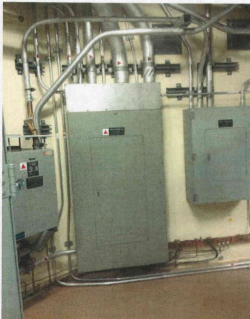
File Name: 2-62-2-2-06.jpeg Description: General View of Component
