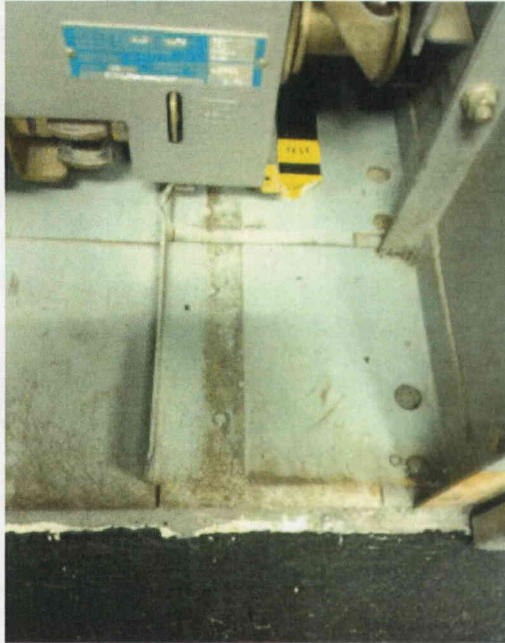
File Name: 2-62-11-2-26.jpeg Description: View of Interior Base
