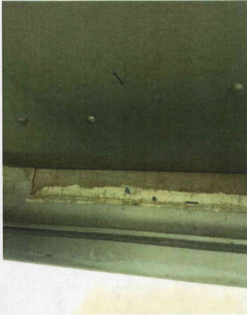
File Name: 2-63-14-2-26.jpeg Description: View of Internal of Back of Cabinet
