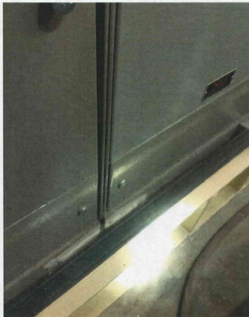
File Name: 2-73-1-2-06.jpeg Description: View of Welds at Component Base
