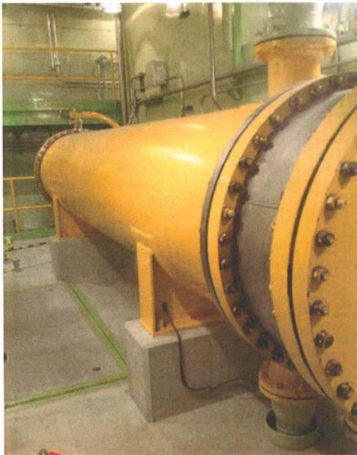
File Name: 2-62-2-2-29.jpeg Description: General View of Component
