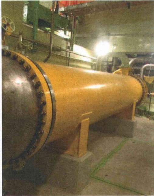
File Name: 2-73-2-2-29.jpeg Description: General View of Component
