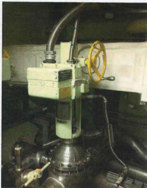
File Name: 2-62-7-2-23.jpeg Description: General View of Component
