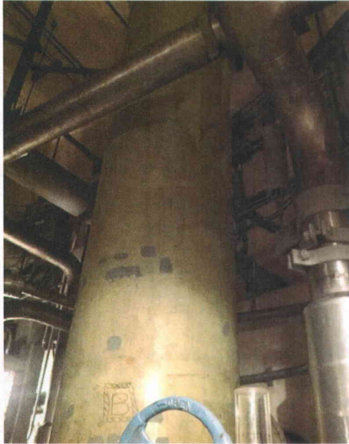
File Name: 2-63-3-2-18.jpeg Description: General View of Component
