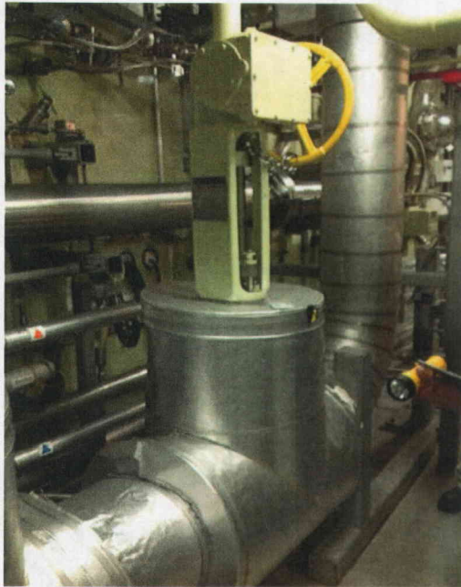
File Name: 2-63-9-2-23.jpeg Description: General View of Main Line and Component
