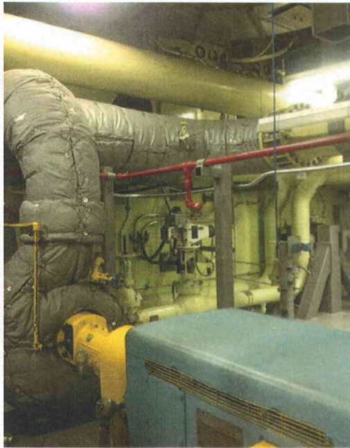
File Name: 2-63-4-2-03.jpeg Description: General View of Main Line and Component
