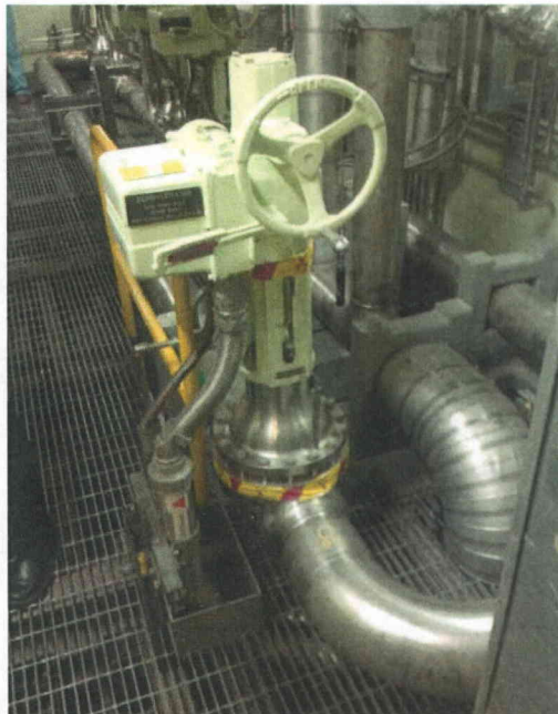
File Name: 2-62-1-2-02.jpeg Description: General View of Component
