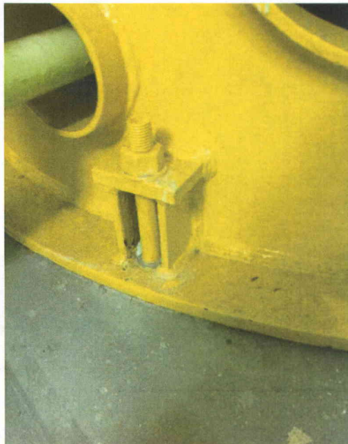
File Name: 2-62-1-2-05.jpeg Description: Close Up View of Anchorage
