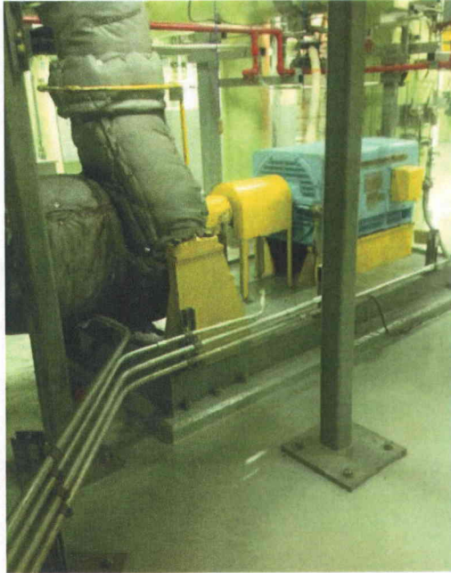
File Name: 2-73-2-2-03.jpeg Description: General View of Component Area
