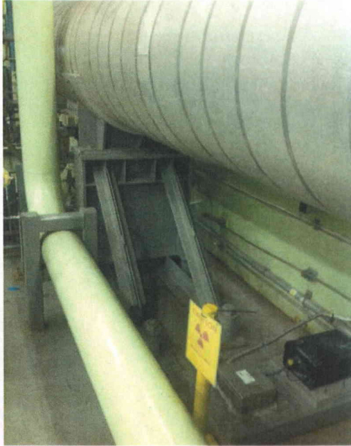
File Name: 2-62-4-2-01.jpeg Description: View of Fixed Support
