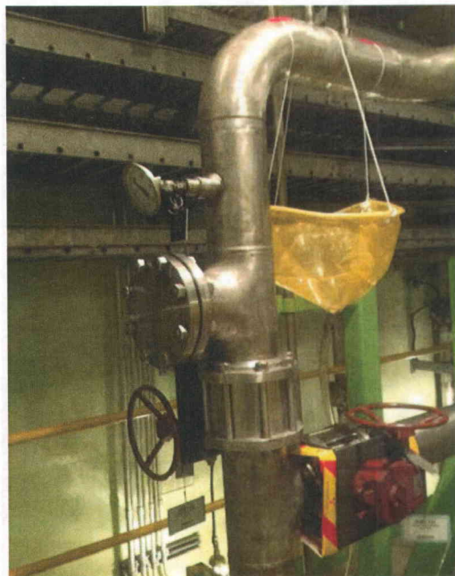
File Name: 2-63-4-2-29.jpeg Description: View of Component Area
