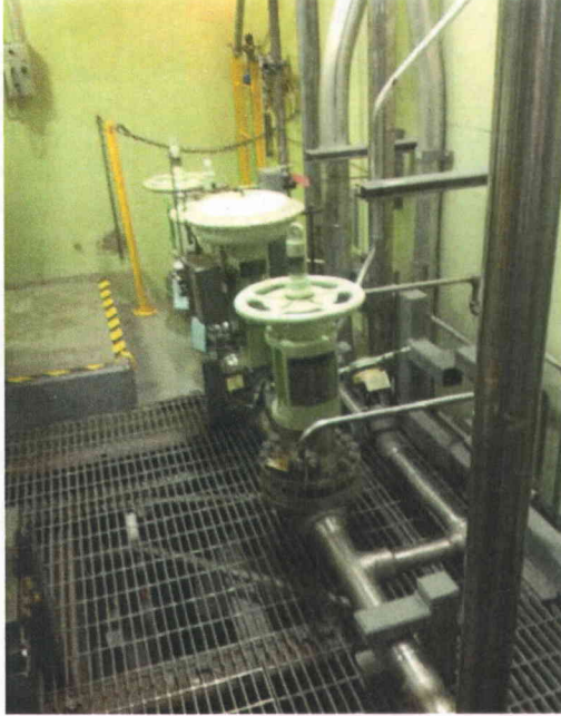
File Name: 2-63-3-2-02.jpeg Description: General View of Component
