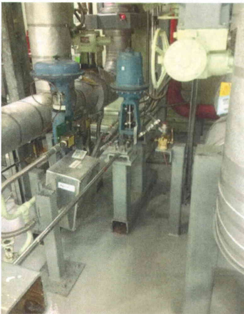
File Name: 2-64-3-2-11.jpeg Description: General View of Component
