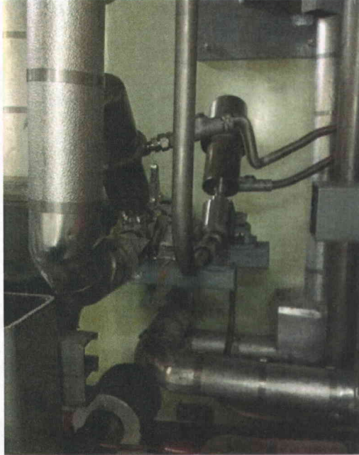
File Name: 2-61-1-2-11.jpeg Description: General View of Component
