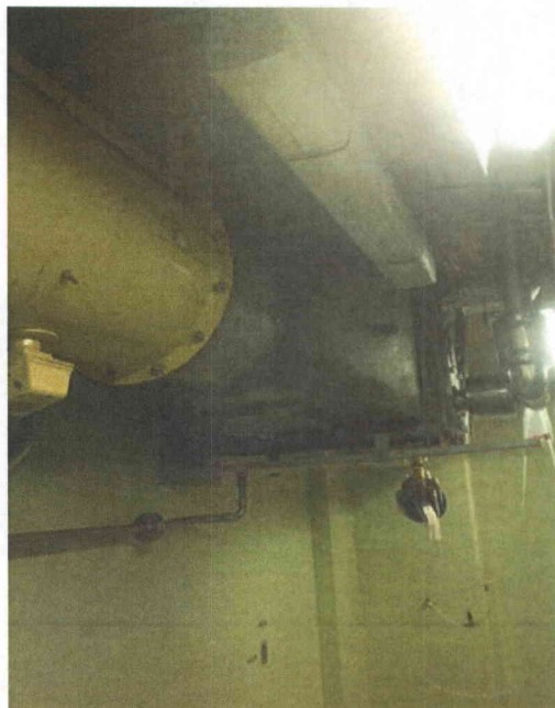
File Name: 2-73-2-2-04.jpeg Description: General View of Component
