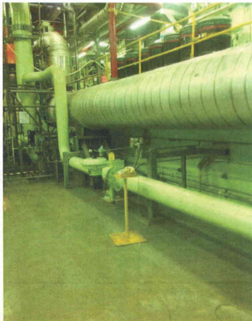
File Name: 2-73-4-2-01.jpeg Description: General View of Component
