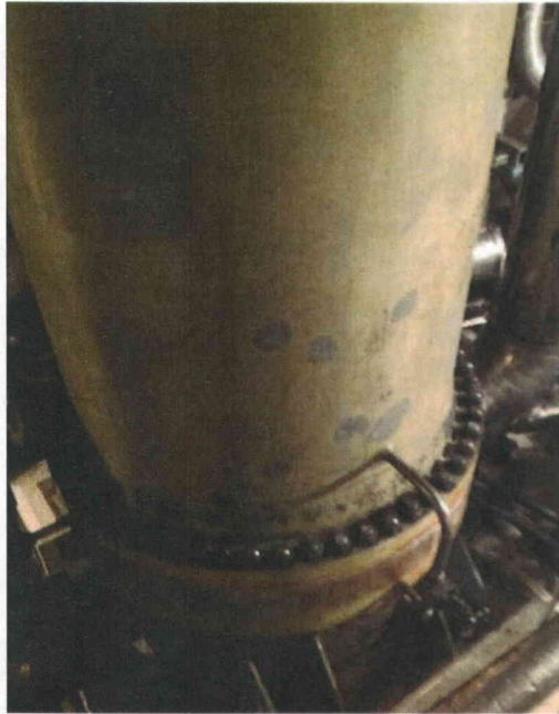
File Name: 2-61-3-2-18.jpeg Description: General View of Anchorage
