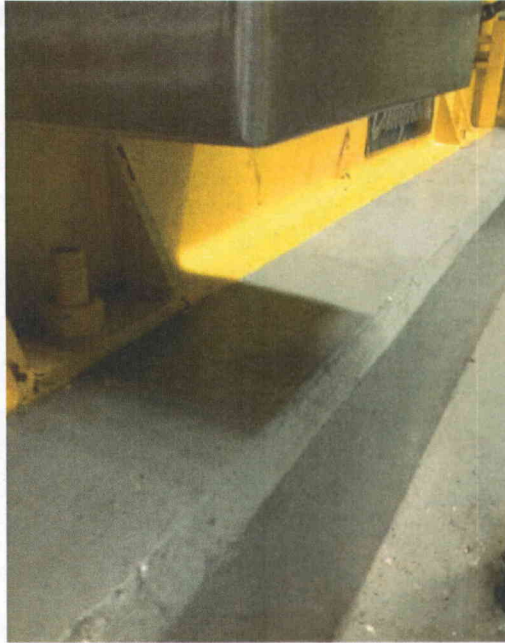
File Name: 2-63-4-2-23.jpeg Description: Close Up View of Anchorage
