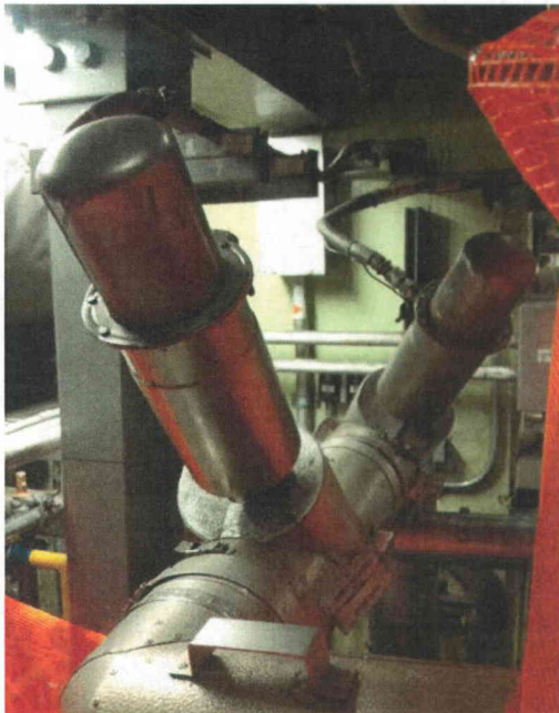
File Name: 2-62-7-2-16.jpeg Description: General View of Component
