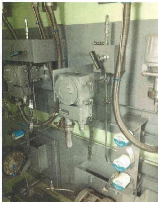
File Name: 2-62-1-2-14.jpeg Description: General View of Component
