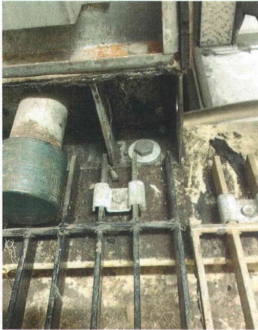
File Name: 2-62-2-2-07.jpeg Description: Close Up View of Anchorage
