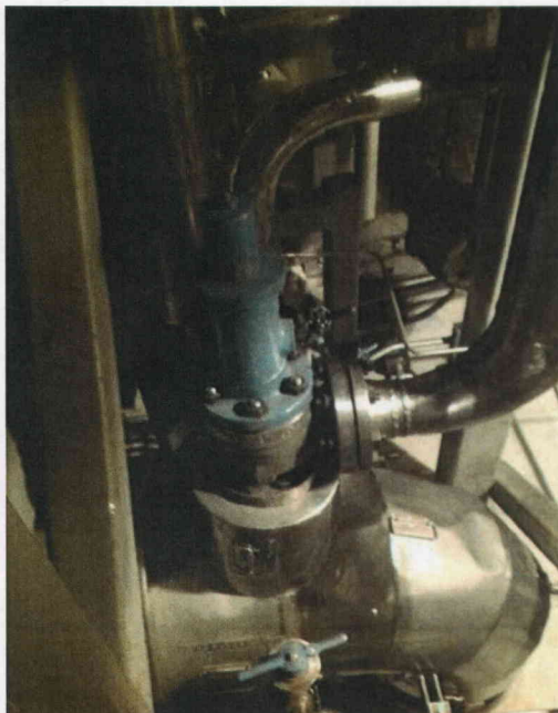
File Name: 2-62-1-2-17.jpeg Description: General View of Component
