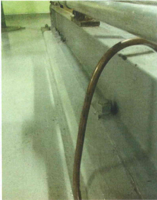
File Name: 2-63-2-2-03.jpeg Description: Close Up View of Anchorage
