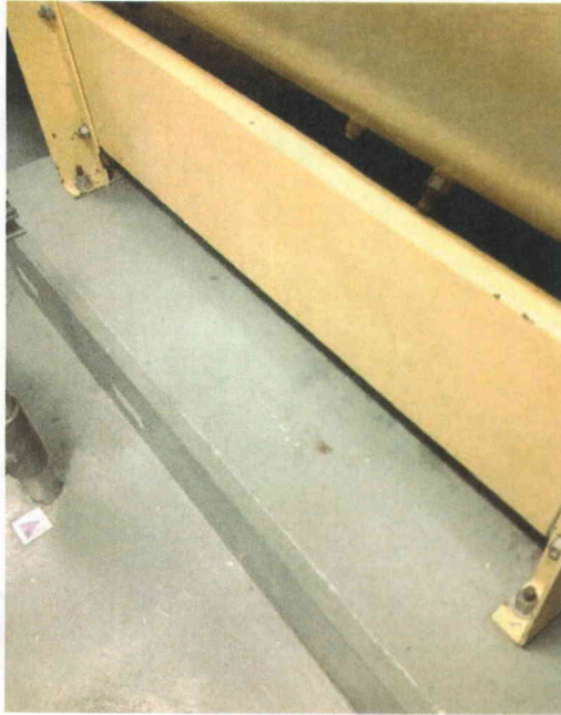
File Name: 2-73-10-2-16.jpeg Description: View of Fan Anchorage
