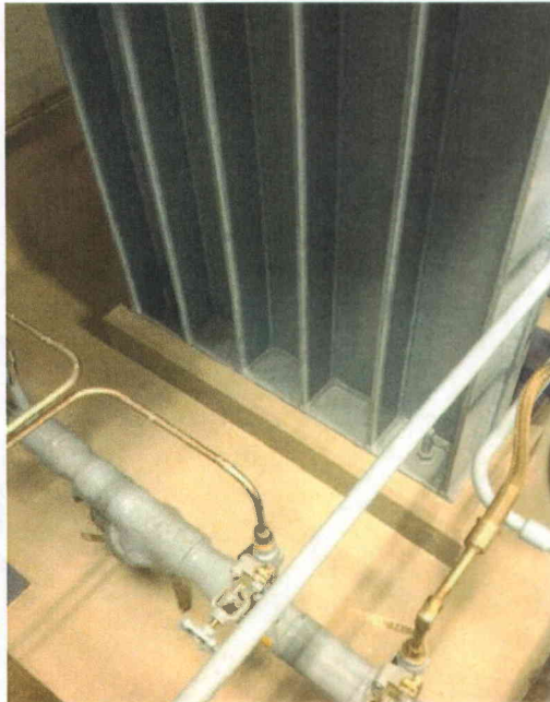
File Name: 2EGF-TK22A(3).jpg Description: View of Anchor Bolts
