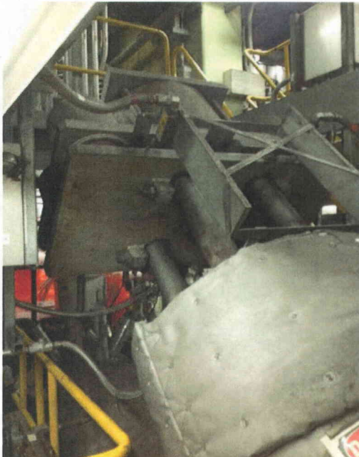
File Name: 2-62-8-2-16.jpeg Description: General View of Component
