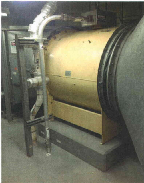
File Name: 2-62-10-2-16.jpeg Description: General View of Component
