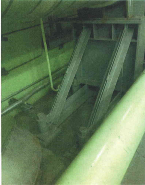
File Name: 2-64-4-2-01.jpeg Description: View of Sliding Support
