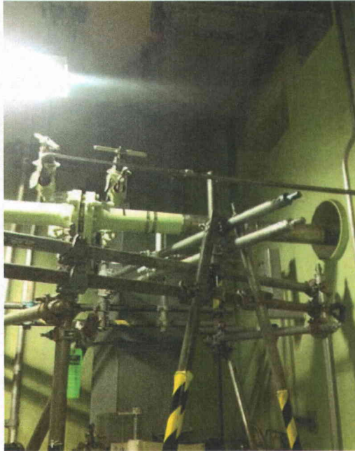
File Name: 2-63-3-2-25.jpeg Description: View of Component Area
