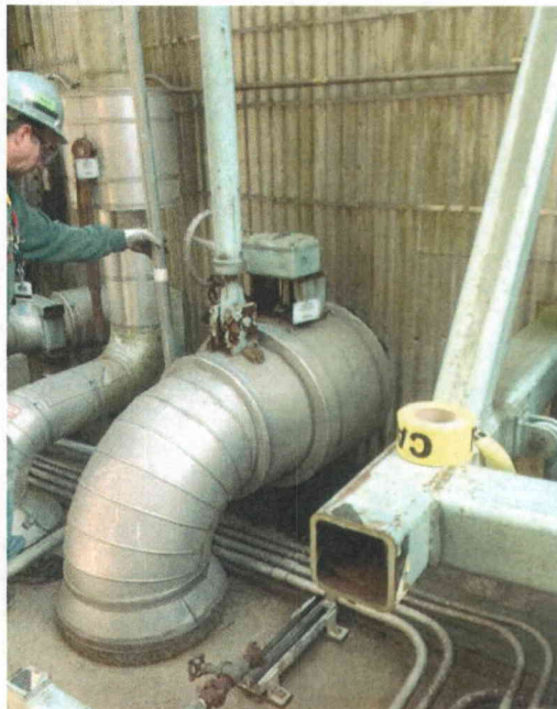
File Name: 2-62-9-2-29.jpeg Description: General View of Component
