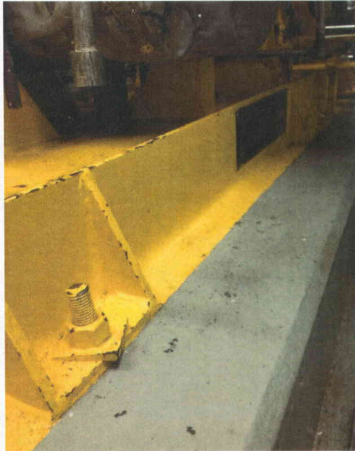
File Name: 2-63-3-2-23.jpeg Description: Close Up View of Anchorage
