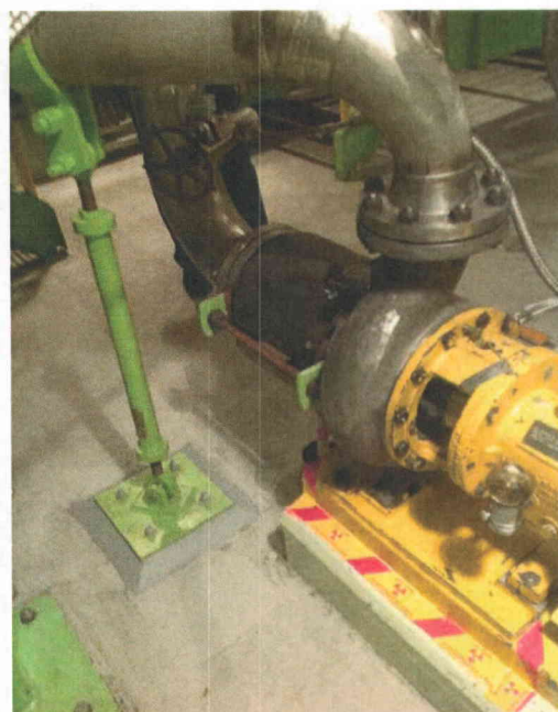
File Name: 2-62-8-2-29.jpeg Description: General View of Component
