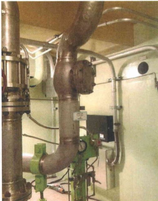
File Name: 2-62-6-2-29.jpeg Description: General View of Component
