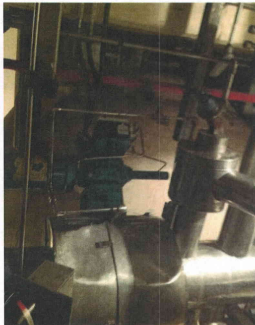
File Name: 2-62-2-2-17.jpeg Description: General View of Component
