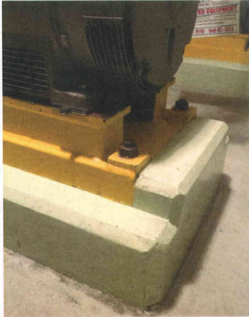
File Name: 2-63-7-2-29.jpeg Description: Close Up View of Anchorage
