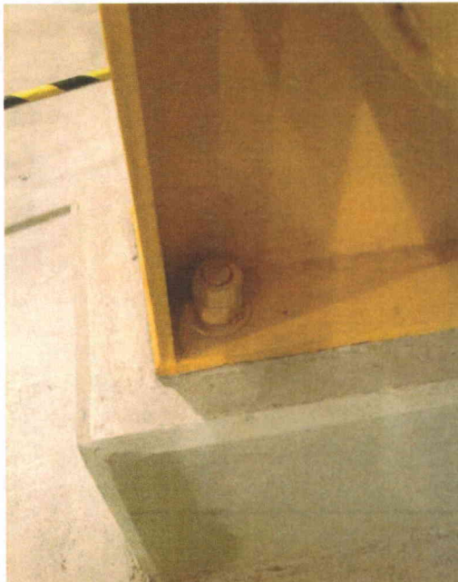
File Name: 2-64-2-2-29.jpeg Description: Close Up View of Anchorage
