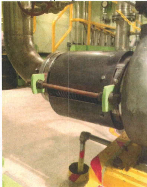
File Name: 2-61-8-2-29.jpeg Description: General View of Component
