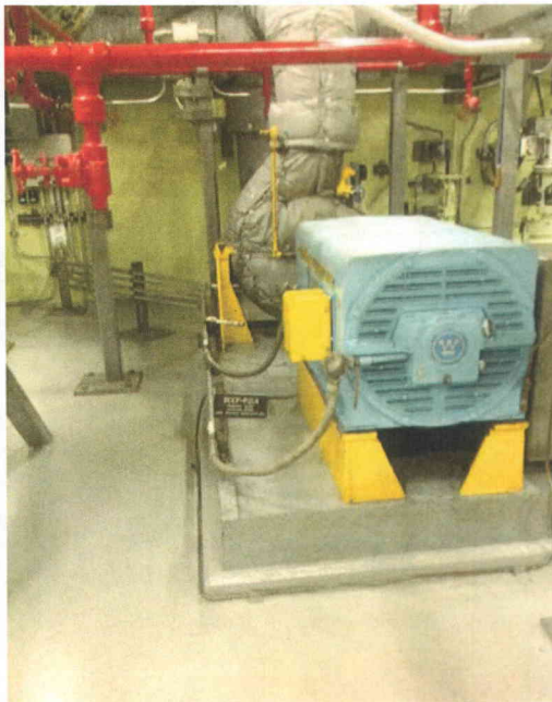
File Name: 2-62-2-2-03.jpeg Description: General View of Component
