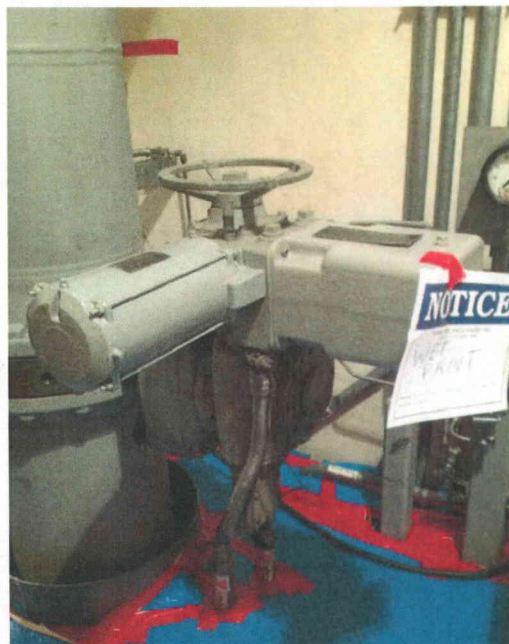
File Name: 2-62-3-2-19.jpeg Description: General View of Component
