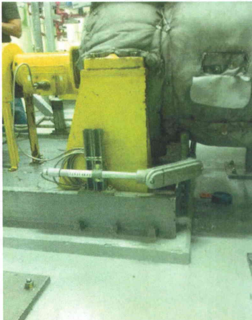
File Name: 2-64-2-2-03.jpeg Description: Close Up View of Anchorage
