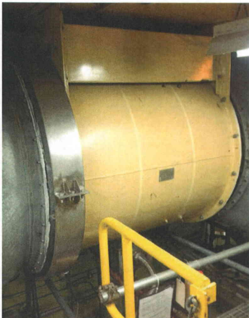
File Name: 2-62-9-2-16.jpeg Description: General View of Component
