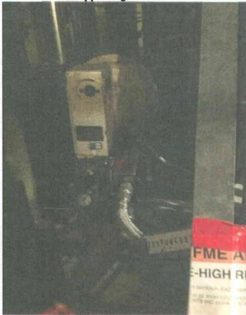
File Name: 2-61-6-2-19.jpeg Description: General View of Component
