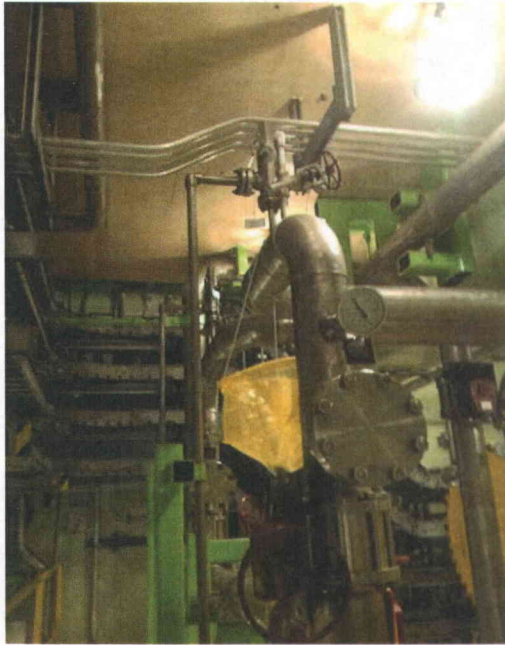
File Name: 2-63-5-2-29.jpeg Description: General View of Component and Main Line
