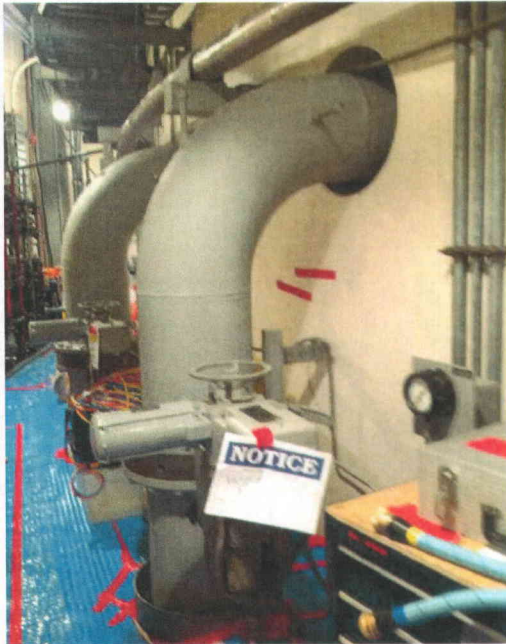
File Name: 2-63-3-2-19.jpeg Description: View of Component Area
