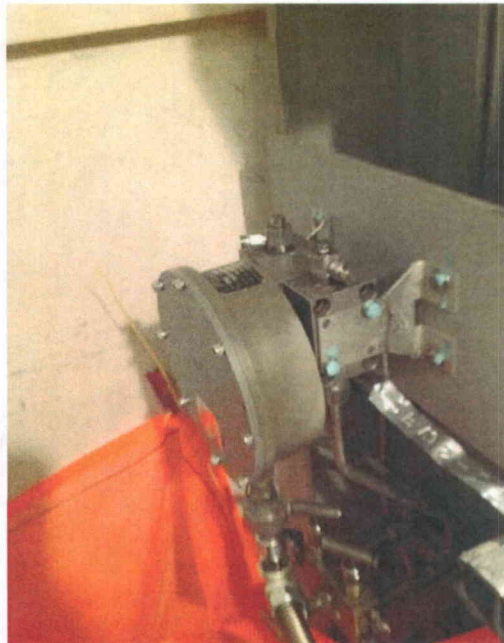
File Name: 2-62-1-2-19.jpeg Description: General View of Component
