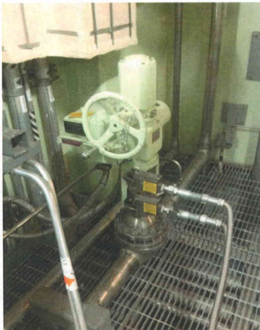
File Name: 2-62-2-2-02.jpeg Description: General View of Component
