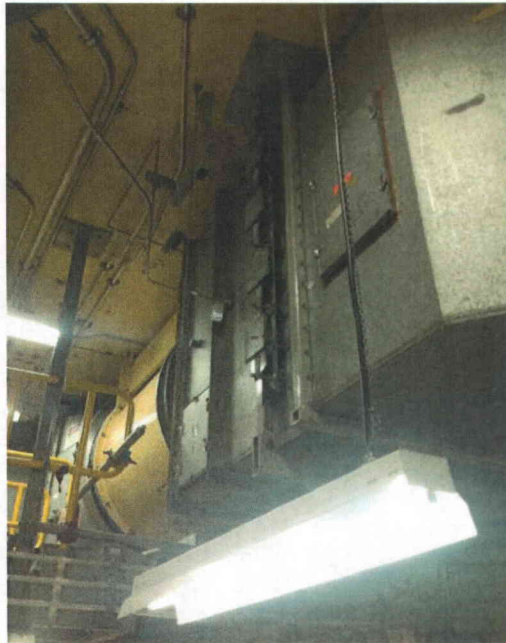
File Name: 2-62-5-2-16.jpeg Description: View of Component Area
