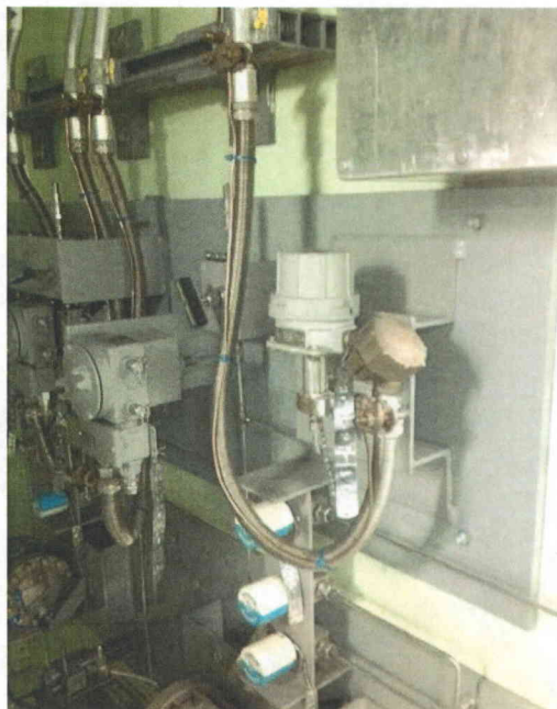
File Name: 2-64-1-2-14.jpeg Description: View of Wall Plate Anchorage
