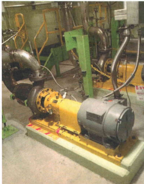
File Name: 2-62-7-2-29.jpeg Description: General View of Component
