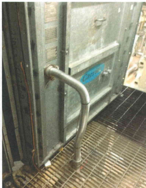
File Name: 2-63-2-2-07.jpeg Description: General View of Component
