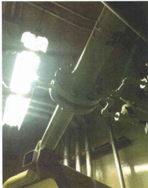
File Name: 2-62-3-2-25.jpeg Description: General View of Component
