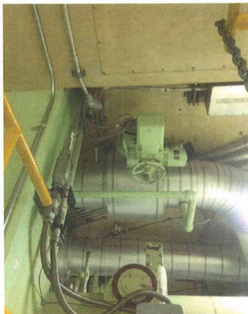
File Name: 2-63-1-2-12.jpeg Description: General View of Main Line and Component
