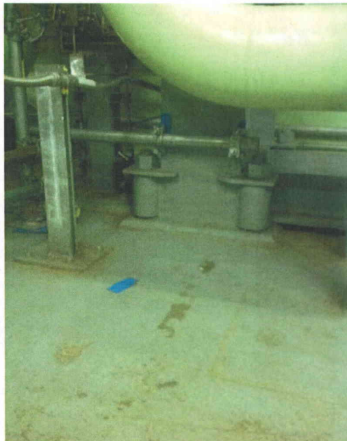
File Name: 2-63-4-2-01.jpeg Description: View of Fixed Support
