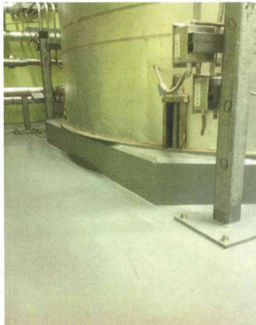
File Name: 2-64-4-2-04.jpeg Description: General View of Pedestal and Anchorage
