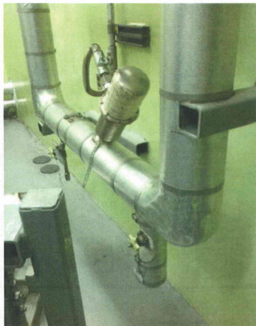
File Name: 2-62-1-2-04.jpeg Description: General View of Component and Main Line
