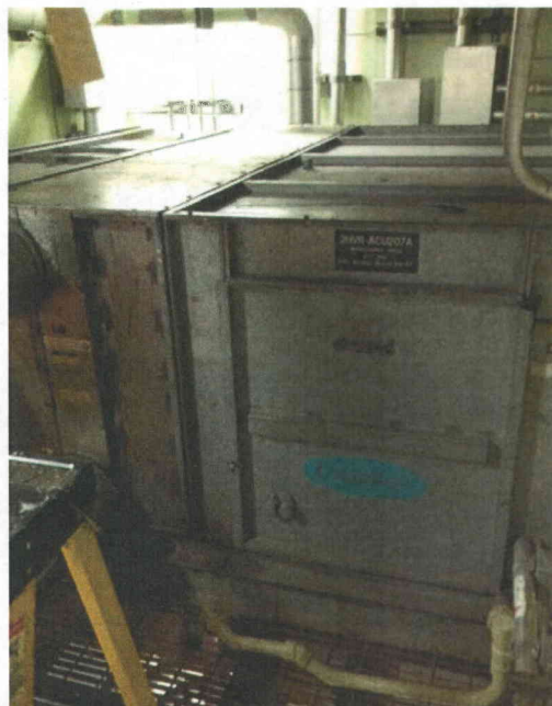
File Name: 2-62-2-2-25.jpeg Description: General View of Component
