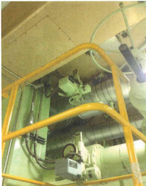
File Name: 2-61-1-2-12.jpeg Description: General View of Component
