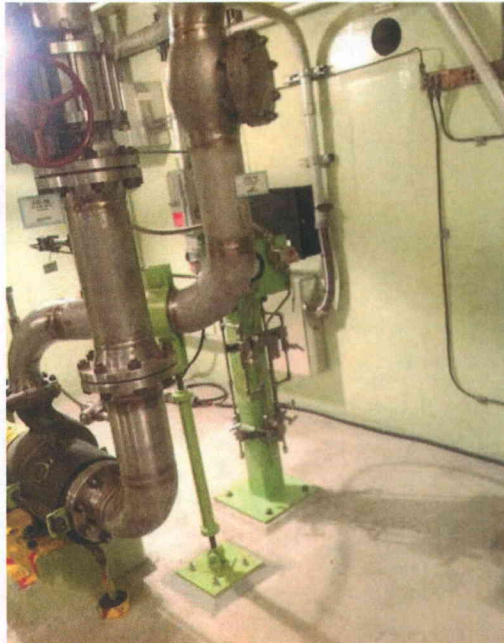
File Name: 2-63-6-2-29.jpeg Description: General View of Component
