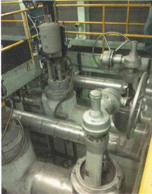
File Name: 2-63-2-2-27.jpeg Description: View of Component Area
