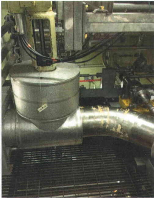
File Name: 2-63-2-2-23.jpeg Description: General View of Main Line and Component
