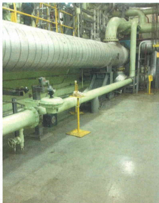
File Name: 2-61-4-2-01.jpeg Description: General View of Component
