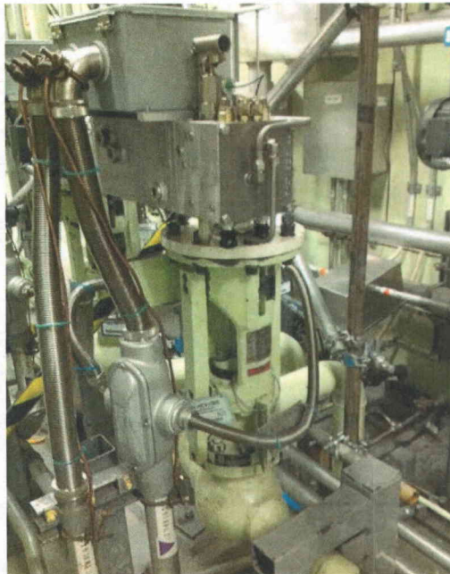
File Name: 2-62-1-2-25.jpeg Description: General View of Component
