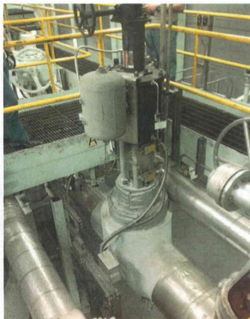
File Name: 2-62-2-2-27.jpeg Description: General View of Component
