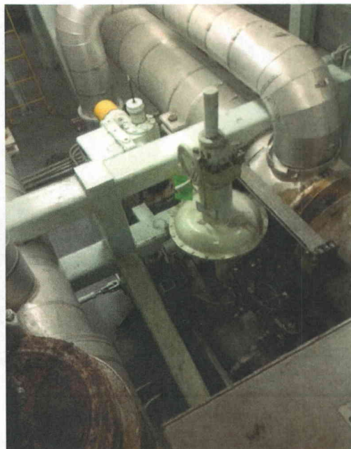
File Name: 2-62-1-2-27.jpeg Description: View of Component Area
