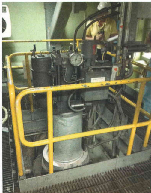
File Name: 2-62-2-2-16.jpeg Description: General View of Component
