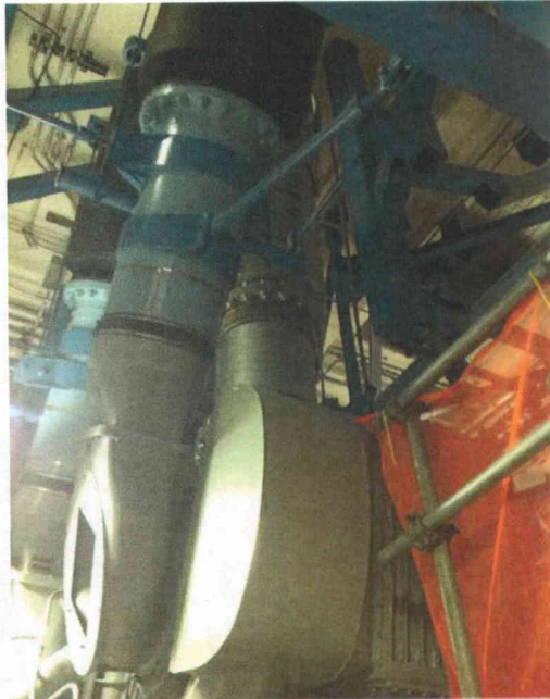
File Name: 2EGS-EG2-1(3).jpg Description: View of Exhaust Pipe Bracing
