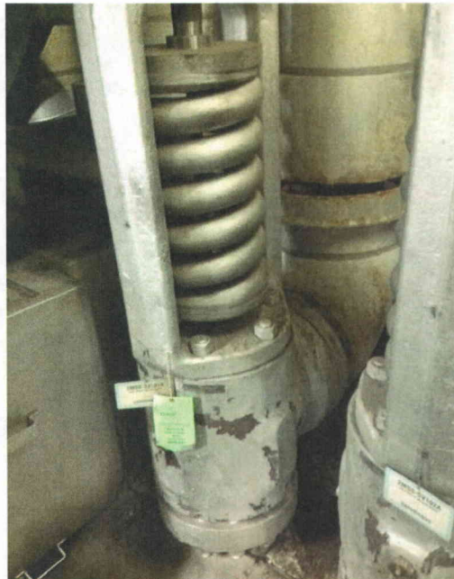
File Name: 2-62-6-2-16.jpeg Description: General View of Component
