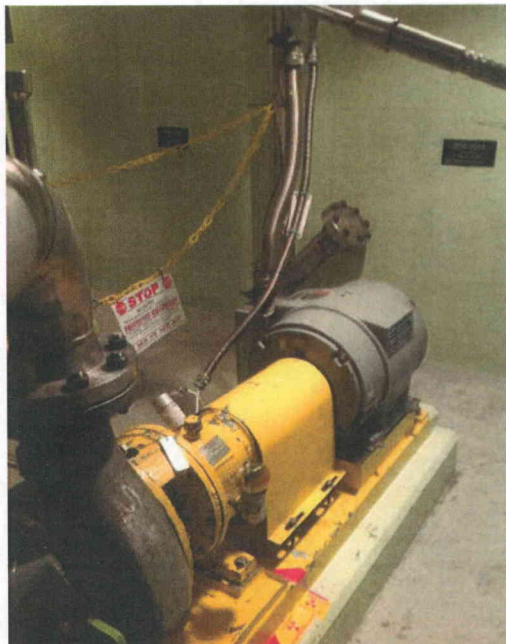
File Name: 2-64-7-2-29.jpeg Description: General View of Component
