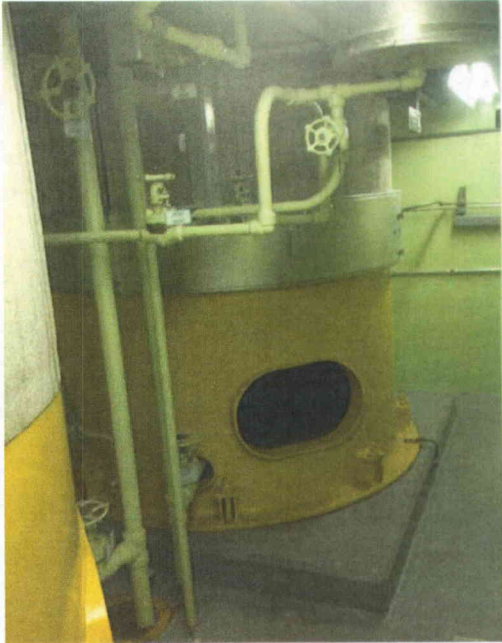
File Name: 2-63-1-2-05.jpeg Description: General View of Component
