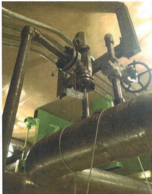
File Name: 2-62-5-2-29.jpeg Description: General View of Component
