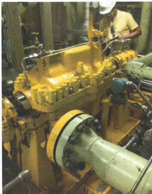
File Name: 2-62-3-2-23.jpeg Description: General View of Component
