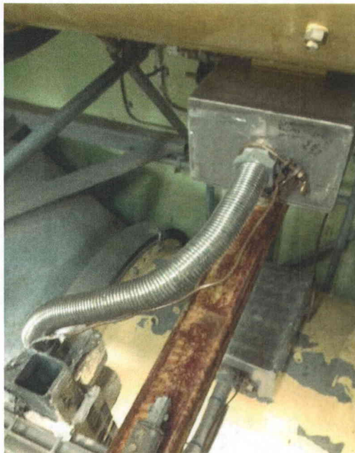
File Name: 2-64-9-2-16.jpeg Description: View of Attached Lines
