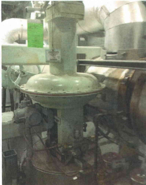
File Name: 2-63-1-2-27.jpeg Description: General View of Component
