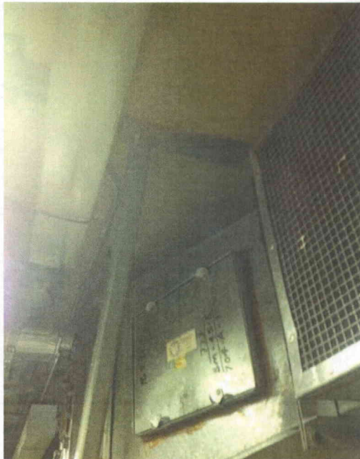
File Name: 2-95-2-2-04.jpeg Description: View of Anchorage to Ceiling
