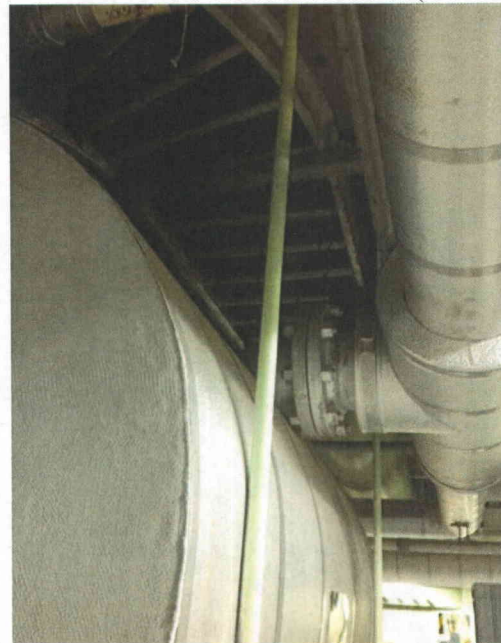
File Name: 1-75-1-4-43.jpeg Description: Unanchored tank, but rod hung. No interaction concern. (The tank is not Cat I)
