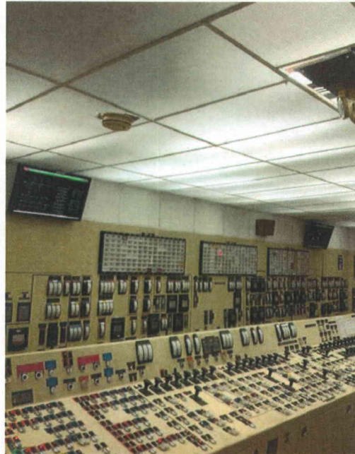
File Name: 1-71-1-4-18.jpeg Description: Several LCD screens are secure and are not a falling concern
