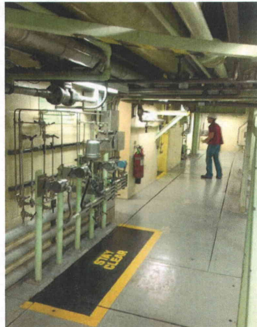
File Name: 1-68-1-4-43.jpeg Description: Block walls, South
