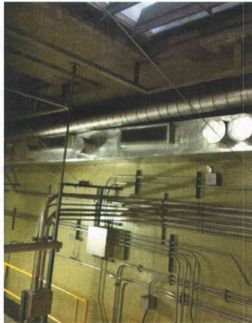
File Name: 1-65-1-4-32.jpeg Description: Ducting in area adequately supported
