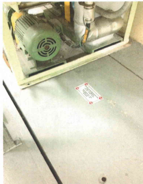
File Name: 1-72-1-4-43.jpeg Description: Unanchored tank, but rod hung. No interaction concern. (The tank is not Cat I)
