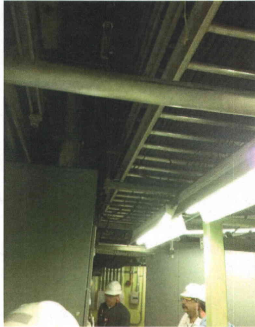
File Name: 1-67-1-4-60.jpeg Description: Cable tray is rod hung with minimal lateral support.
