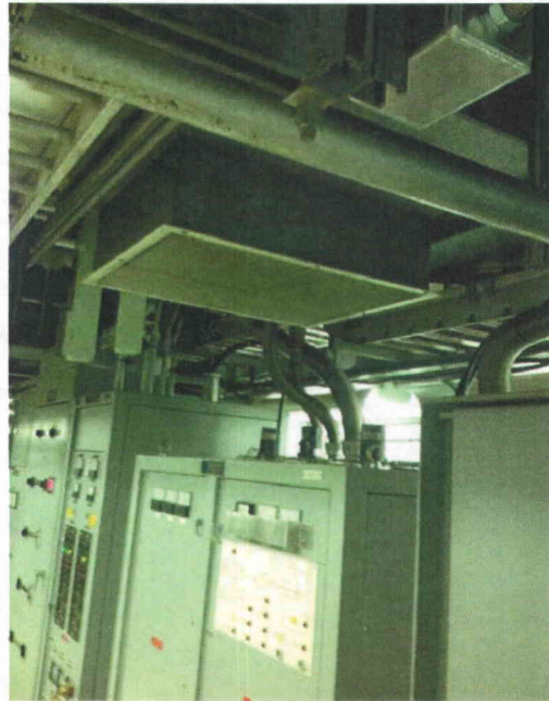
File Name: 1-71-1-4-25.jpeg Description: HVAC grill over INV-VITBUS1-3 judged adequately restrained.
