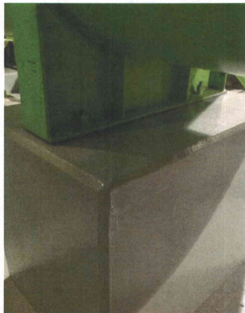
File Name: 1-68-3-4-60.jpeg Description: Small gap under base of FC-E-1B judged not a concern.
