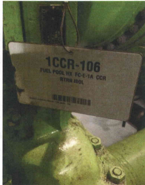
File Name: 1-67-3-4-60.jpeg Description: One nut with one-half thread engagement missing, judged acceptable.
