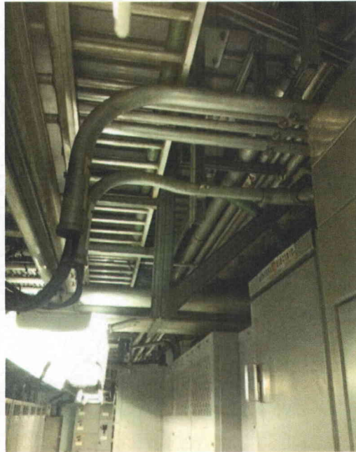
File Name: 1-72-1-4-26.jpeg Description: Cable tray has long rod support, but is laterally braced and judged a non issue
