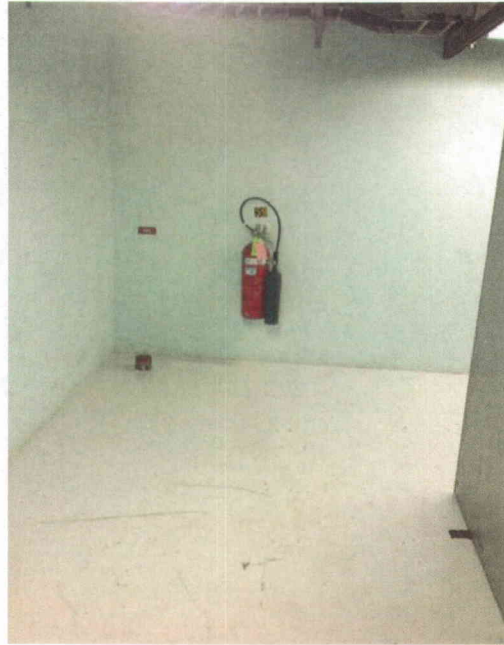
File Name: 1-69-1-4-25.jpeg Description: View of nearby fire extinguisher
