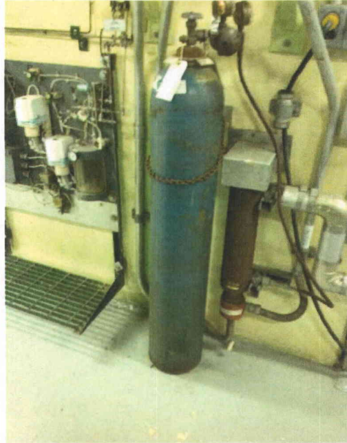
File Name: 1-67-1-4-46.jpeg Description: Gas bottle with only one chain at top near Post Accident Sampling panel PA5C1 judged OK.
