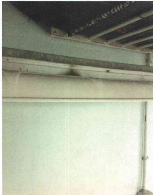
File Name: 1-68-1-4-25.jpeg Description: Light has burn marks on it, appears disused. Considered a non issue.
