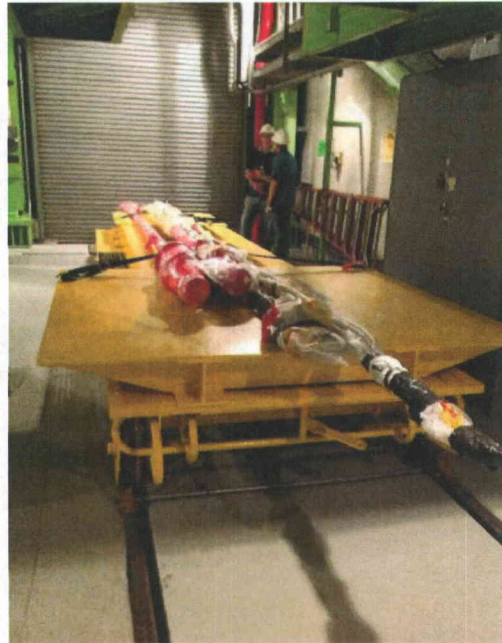
File Name: 1-76-3-4-60.jpeg Description: Cart, ladder, and fire pipe, all secured, judged a non issue.
