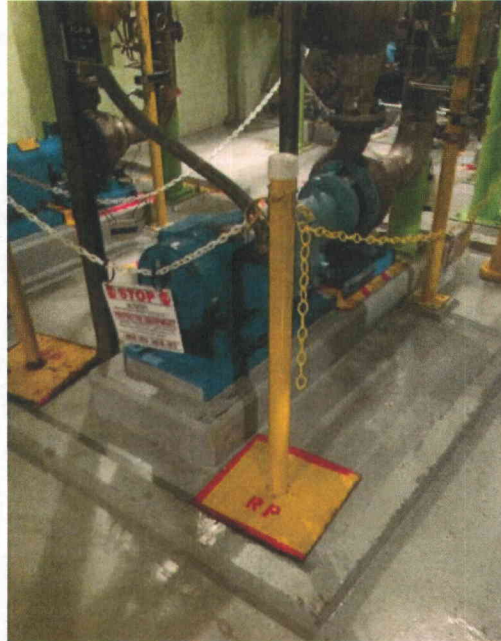
File Name: 1-74-3-4-60.jpeg Description: Posts located near component. Judged not a significant seismic concern.
