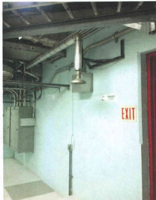
File Name: 1-71-1-4-26.jpeg Description: Emergency shower is rugged, judged not a spray concern
