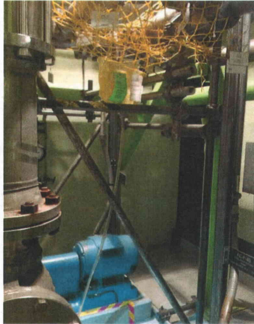
File Name: 1-72-3-4-60.jpeg Description: Scaffold in area is adequately braced.
