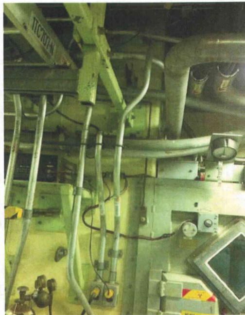
File Name: 1-66-1-4-46.jpeg Description: HSS hung cable tray is axially braced and judged a non issue.
