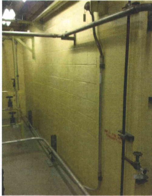
File Name: 1-67-4-4-60.jpeg Description: Block wall in area
