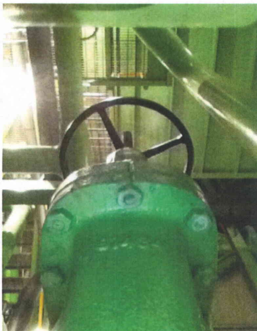
File Name: 1-66-3-4-60.jpeg Description: Underside of not engaged nut. Judged acceptable.
