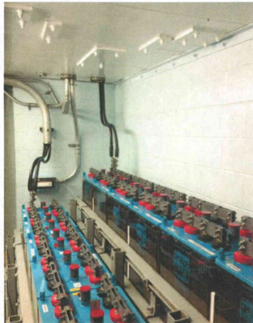
File Name: 1-60-1-4-01.jpeg Description: Block wall in area
