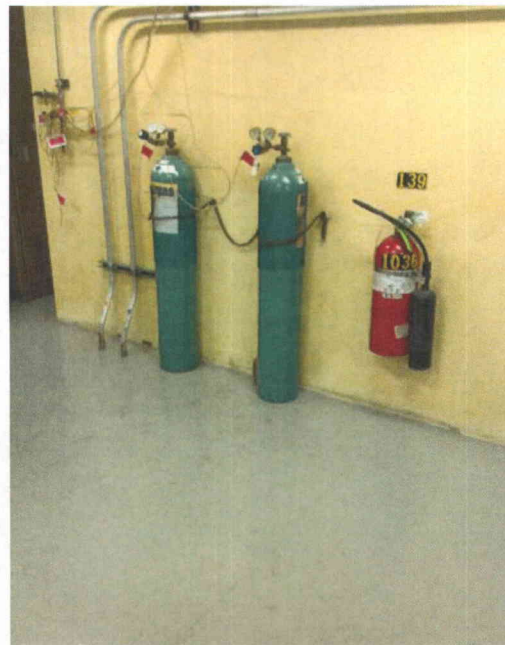
File Name: 1-66-4-4-60.jpeg Description: Fire extinguisher in area and chained gas bottle judged not to be interaction concerns
