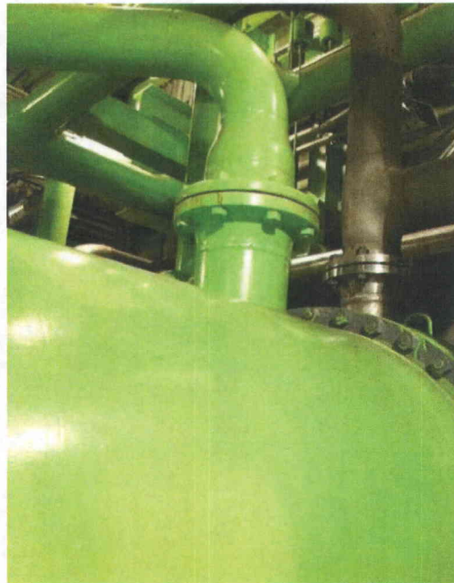
File Name: 1-75-3-4-60.jpeg Description: Thread engagement at heat exchanger FC-E-1B nozzle is judged acceptable.
