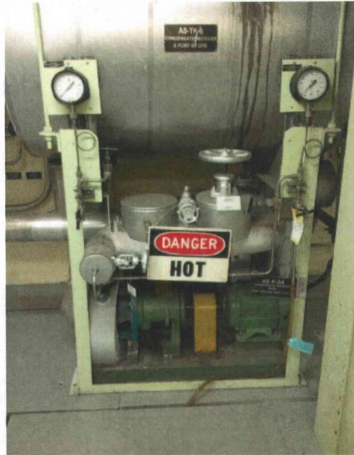
File Name: 1-74-1-4-43.jpeg Description: Unanchored tank, but rod hung. No interaction concern. (The tank is not Cat I)
