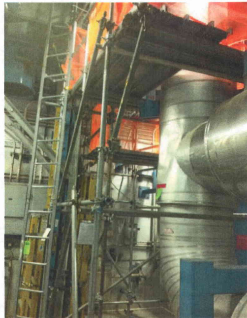
File Name: 1-66-1-4-28.jpeg Description: Temporary scaffold not an issue
