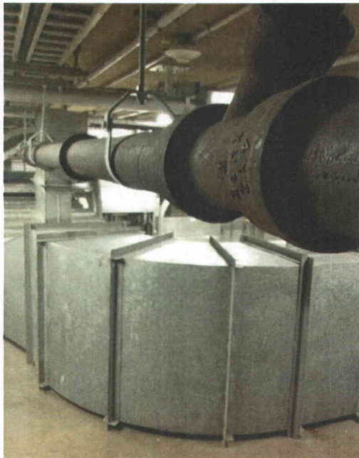
File Name: 1-66-1-4-56.jpeg Description: View of cast iron pipe located in the area.
