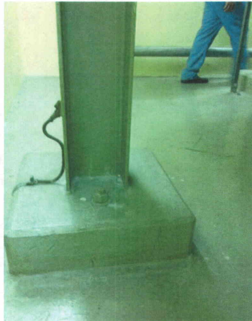
File Name: 1-66-1-4-14.jpeg Description: Gap between nut and base on west post
