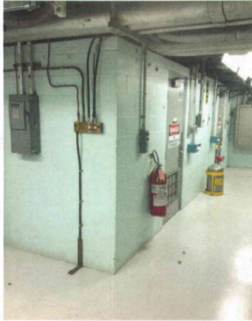
File Name: 1-65-1-4-26.jpeg Description: Block wall, fire ext, fire danger sign
