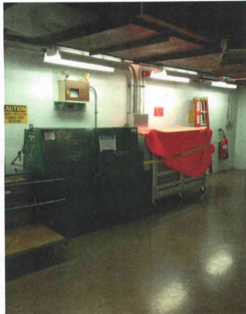
File Name: 1-65-1-4-33.jpeg Description: View of carts, ladders and fire extinguisher in the area
