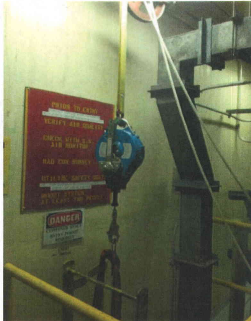
File Name: 1-65-1-4-58.jpeg Description: Lifting hook unsecured. Judged not to cause interaction concerns.
