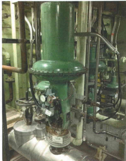
File Name: 2-62-1-1-38.jpeg Description: General view of component
