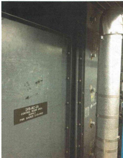
File Name: 2-62-1-1-06.jpeg Description: General view of component
