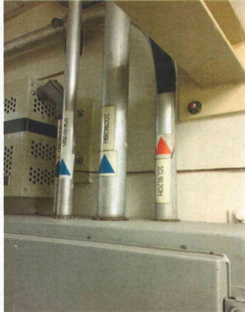
File Name: 2-63-2-1-18.jpeg Description: View of top entry conduits
