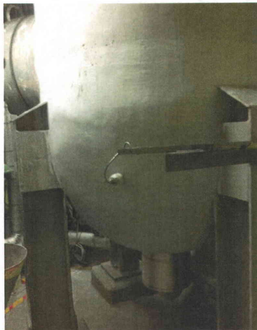
File Name: 2-62-1-1-42.jpeg Description: General view of component
