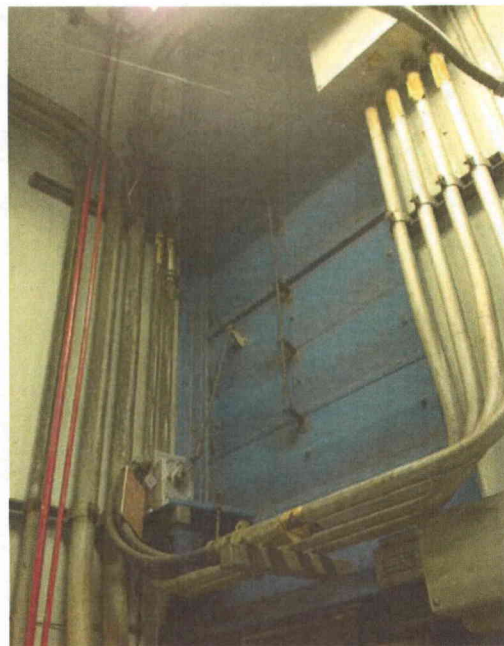
File Name: 2-62-1-1-21.jpeg Description: General view of component
