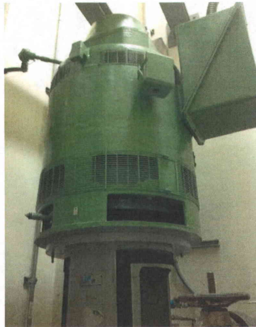
File Name: 2-61-1-1-10.jpeg Description: General view of component
