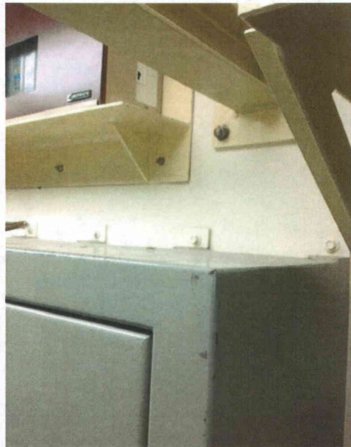
File Name: 2-64-3-1-18.jpeg Description: View of typical wall anchorage configuration
