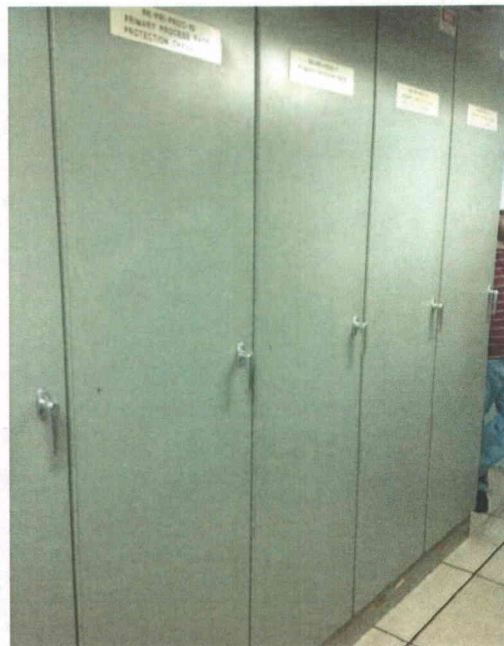
File Name: 2-62-2-1-49.jpeg Description: General view of component
