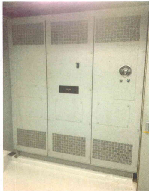
File Name: 2-62-7-1-26.jpeg Description: General view of component
