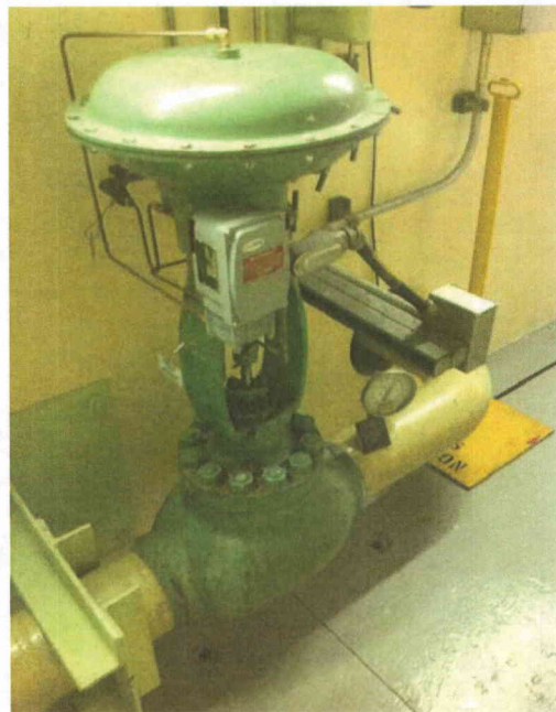
File Name: 2-62-1-1-41.jpeg Description: General view of component
