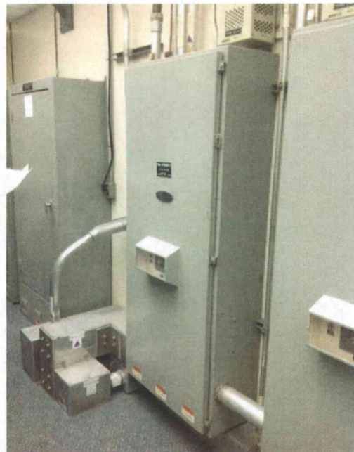
File Name: 2-62-1-1-18.jpeg Description: General view of component
