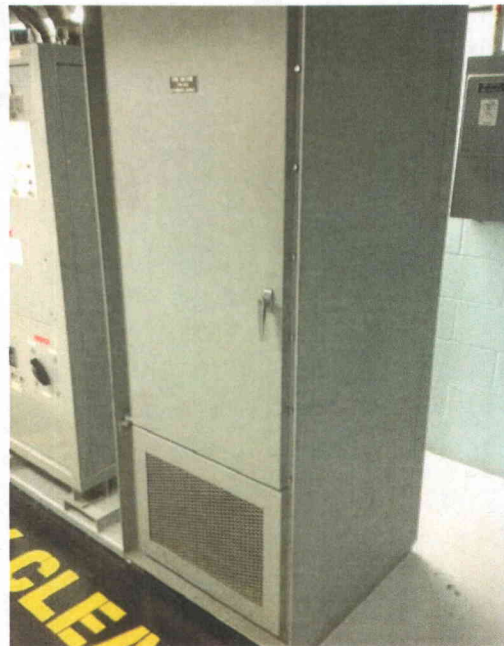
File Name: 2-62-7-1-25.jpeg Description: General view of component
