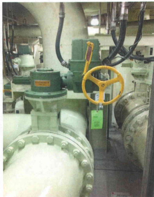
File Name: 2-62-3-1-43.jpeg Description: General view of component
