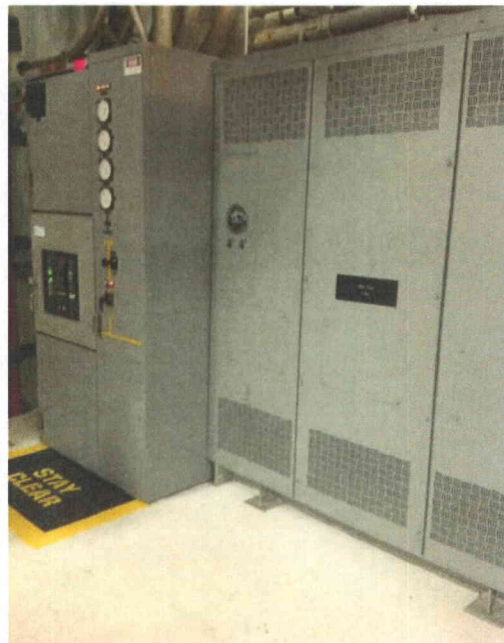
File Name: 2-62-1-1-34.jpeg Description: General view of component
