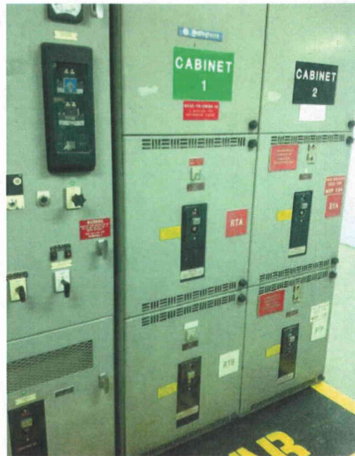
File Name: 2-62-1-1-33.jpeg Description: General view of component
