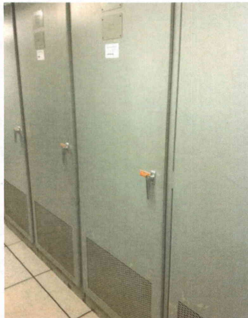
File Name: 2-62-1-1-49.jpeg Description: General view of component
