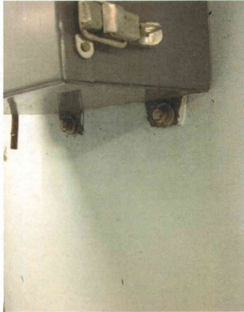
File Name: 2-63-5-1-25.jpeg Description: Bottom wall mounting configuration
