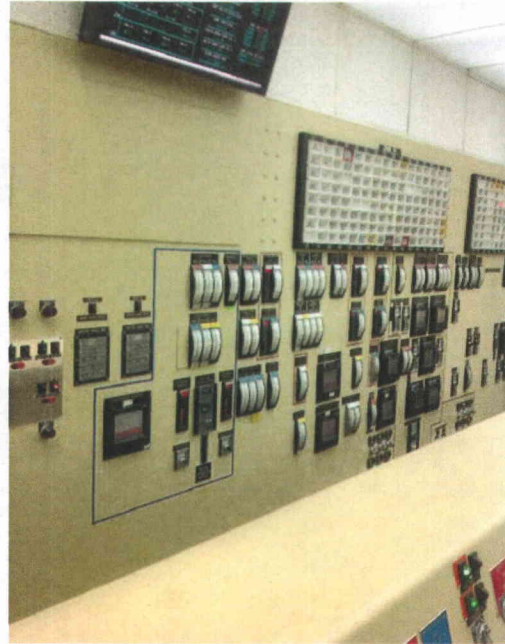
File Name: 2-61-6-1-18.jpeg Description: General view of component
