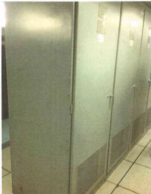
File Name: 2-62-3-1-49.jpeg Description: General view of component
