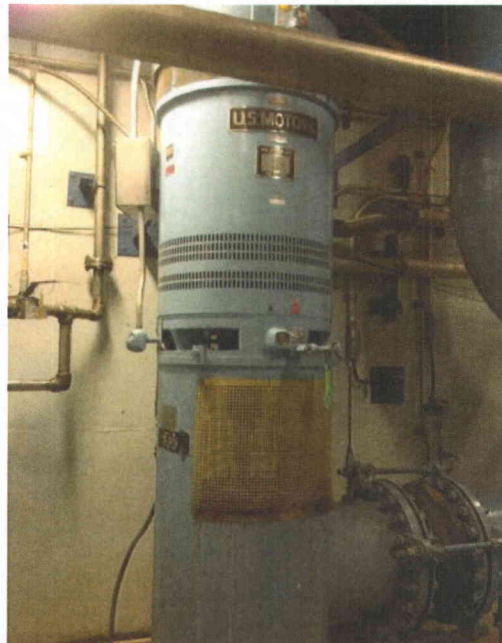
File Name: 2-62-2-1-28.jpeg Description: General view of component
