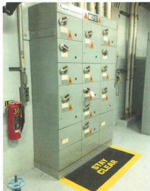
File Name: 2-62-7-1-20.jpeg Description: General view of component
