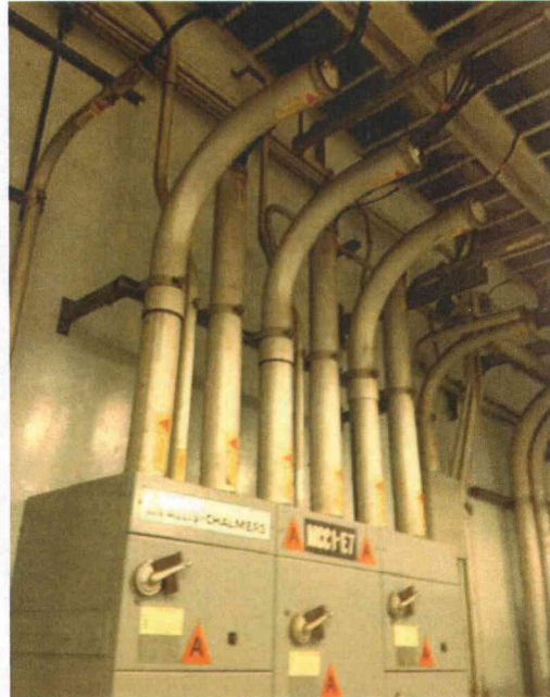
File Name: 2-63-7-1-20.jpeg Description: View of top entry conduits
