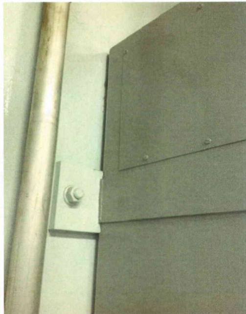
File Name: 2-64-7-1-20.jpeg Description: View of wall mounted lateral support
