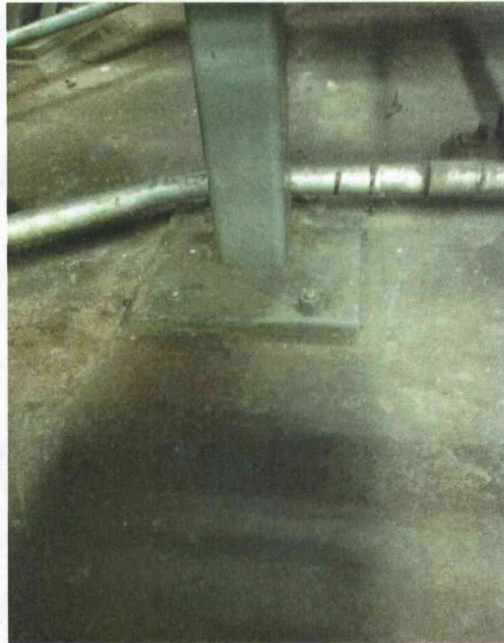
File Name: 2-63-7-1-32.jpeg Description: View of base anchorage configuration
