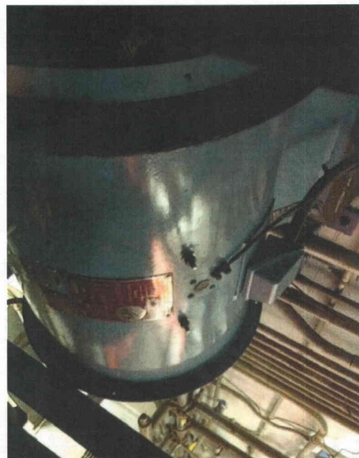
File Name: 2-62-4-1-28.jpeg Description: General view of component
