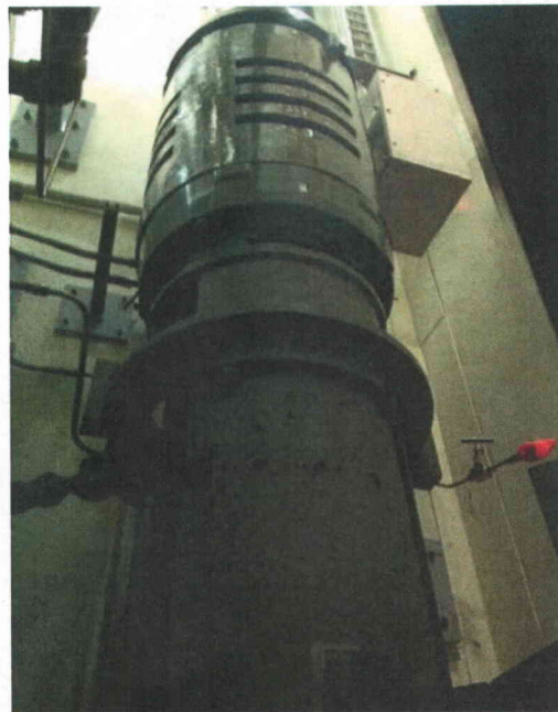
File Name: 2-61-1-1-31.jpeg Description: General view of component
