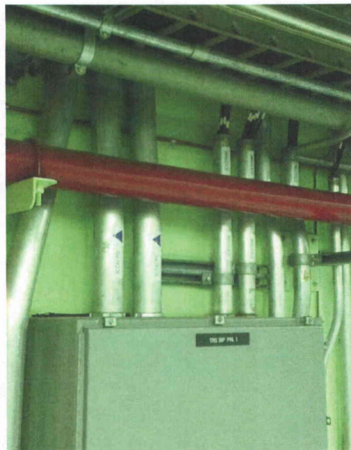
File Name: 2-64-1-1-23.jpeg Description: View of top entry conduits
