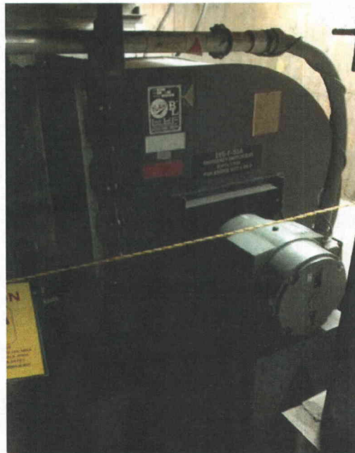
File Name: 2-62-1-1-56.jpeg Description: General view of component
