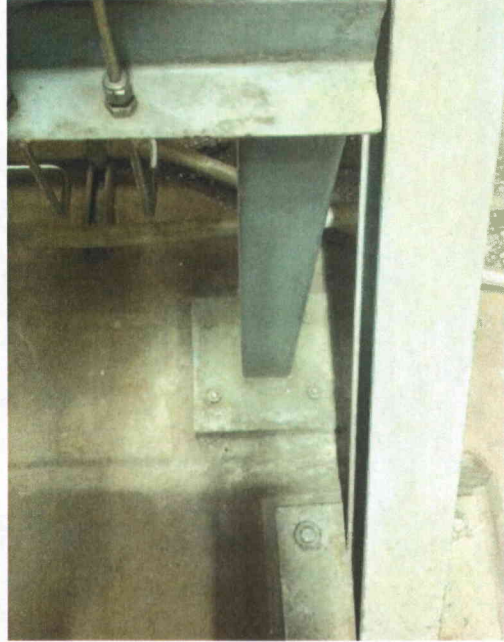
File Name: 2-63-8-1-32.jpeg Description: View of base anchorage configuration
