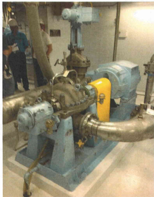
File Name: 2-62-7-1-50.jpeg Description: General view of component
