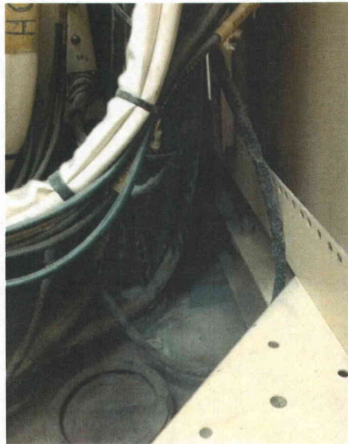
File Name: 2-64-4-1-18.jpeg Description: View of anchorage between cabinet housing and base frame
