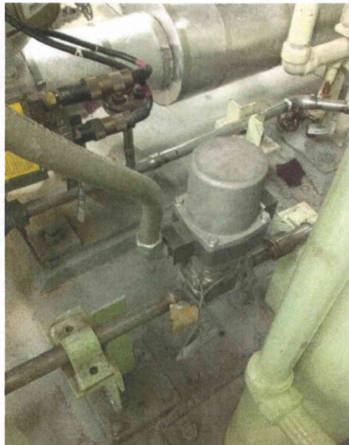
File Name: 2-62-2-1-38.jpeg Description: General view of component
