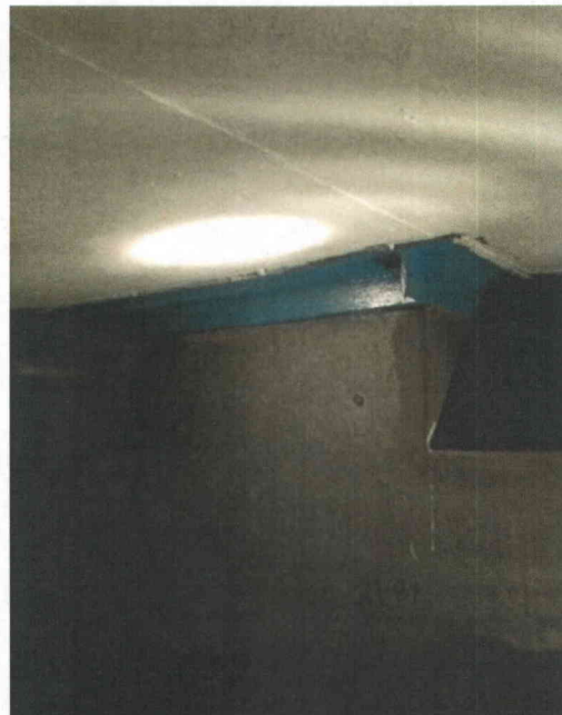
File Name: 2-63-1-1-29.jpeg Description: View of angle framing connected to ceiling
