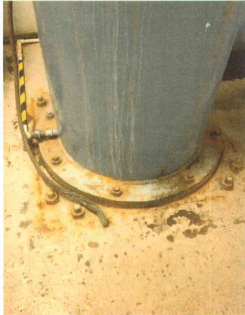
File Name: 2-63-2-1-28.jpeg Description: View of anchorage configuration
