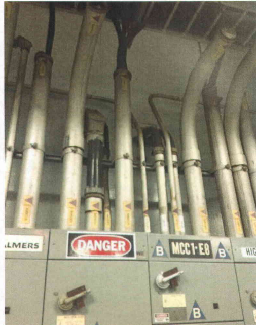
File Name: 2-63-1-1-22.jpeg Description: View of top entry conduits
