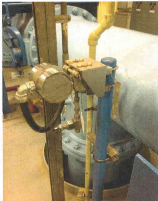
File Name: 2-62-1-1-45.jpeg Description: General view of component
