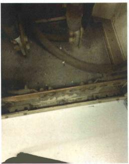
File Name: 2-95-11-1-25.jpeg Description: One 1/2" diam anchor bolt identified at back of breaker.
