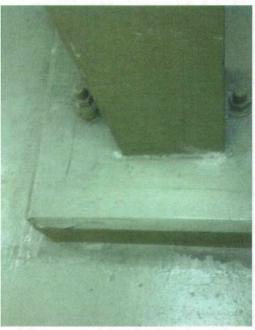
File Name: 2-63-1-1-14.jpeg Description: View of anchorage detail for a typical tank support
