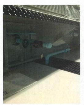
File Name: 2-73-8-1-20.jpeg Description: View of base detail showing no grout below DG's middle section.
