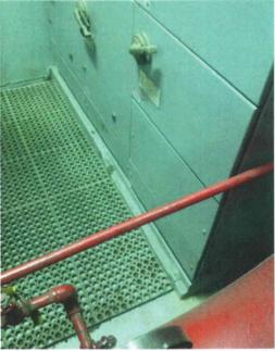
File Name: 2-63-1-1-27.jpeg Description: View of spalled concrete at base of MCC
