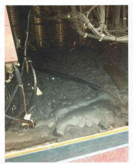
File Name: 2-62-5-1-18.jpeg Description: View of insulating material covering component anchorage
