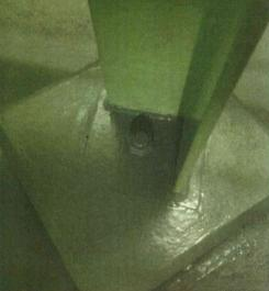
File Name: 2-62-1-1-15.jpeg Description: View of anchorage detail for a typical tank support
