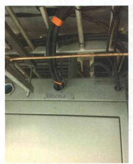
File Name: 2-73-1-1-25.jpeg Description: View of flexible lines going though switch board cabinet
