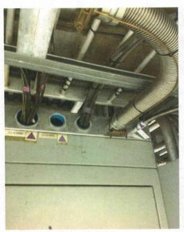
File Name: 2-64-6-1-26.jpeg Description: View of flexible lines going though switch board cabinet
