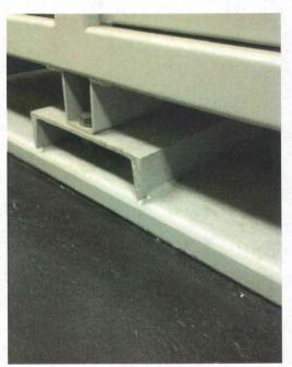
File Name: 2-94-2-1-26.jpeg Description: View of weld detail on channel mounting base
