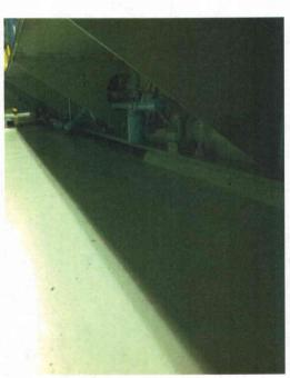
File Name: 2-73-3-1-21.jpeg Description: View of base detail showing no grout below DG's middle section.
