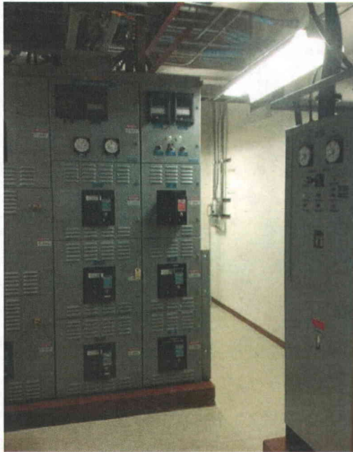
File Name: 1-59-1-1-02.jpeg Description: General view of room
