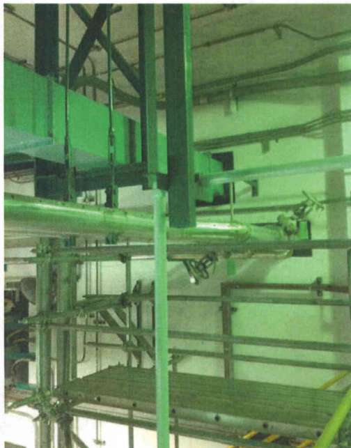
File Name: 1-60-1-1-11.jpeg Description: View of HVAC duct wall penetration
