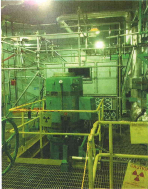
File Name: 1-59-1-1-19.jpeg Description: General View of Room
