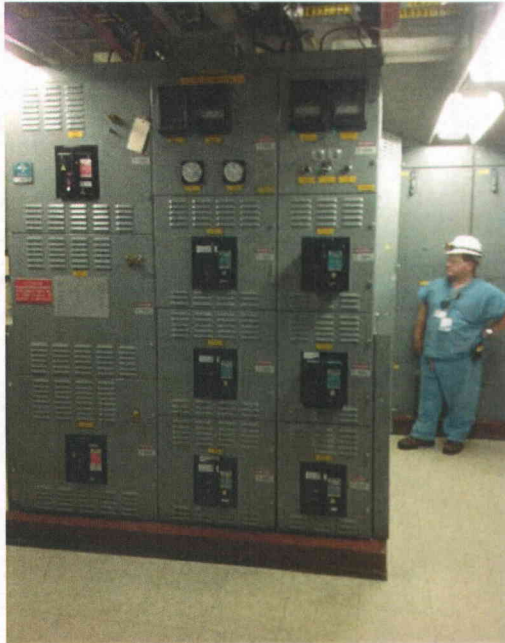
File Name: 1-59-3-1-02.jpeg Description: General view of room
