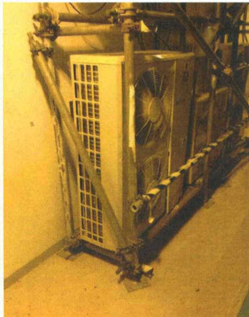
File Name: 1-60-3-1-14.jpeg Description: Scaffold structure for chiller unit
