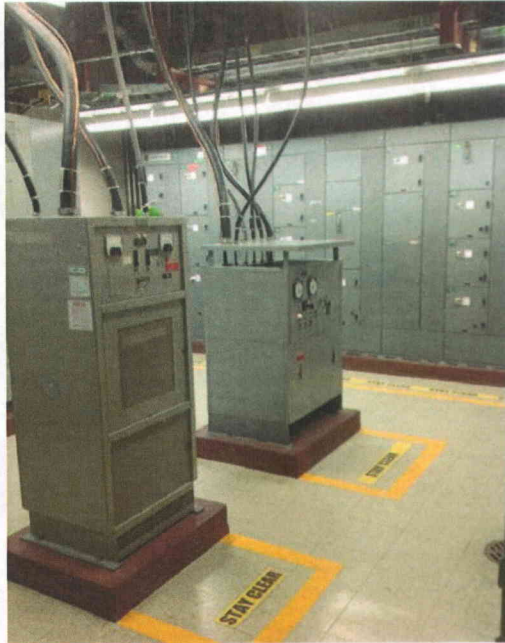
File Name: 1-59-2-1-06.jpeg Description: General view of room
