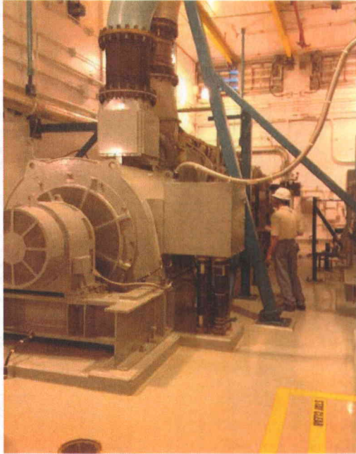
File Name: 1-59-2-1-08.jpeg Description: General view of room
