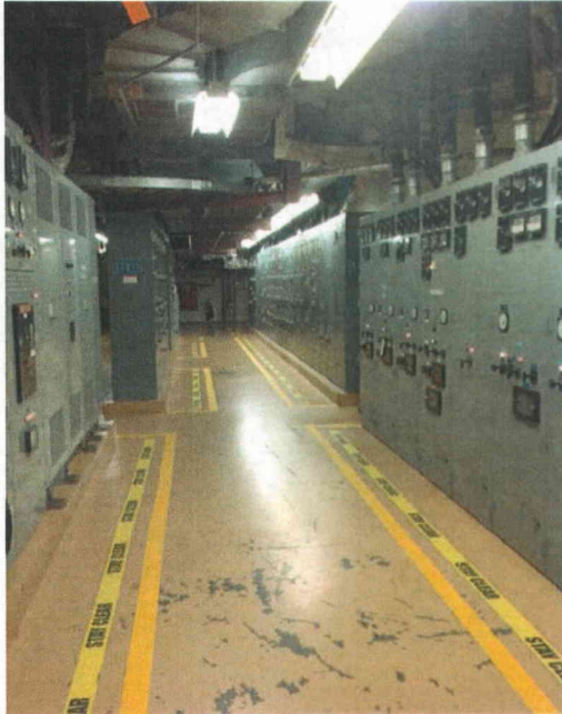
File Name: 1-59-1-1-06.jpeg Description: General view of room
