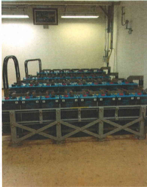
File Name: 1-59-4-1-02.jpeg Description: General view of room
