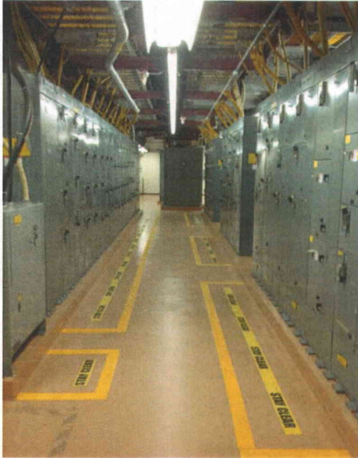
File Name: 1-59-3-1-06.jpeg Description: General view of room
