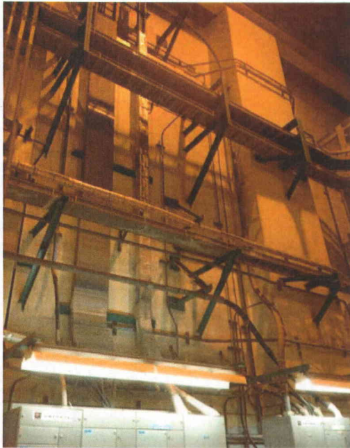
File Name: 1-59-1-1-05.jpeg Description: Raceways rigidly supported
