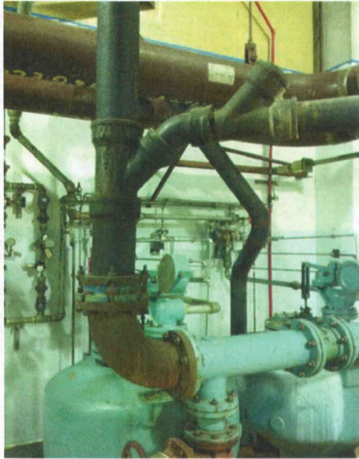
File Name: 1-71-1-1-01.jpeg Description: Cast iron pipe
