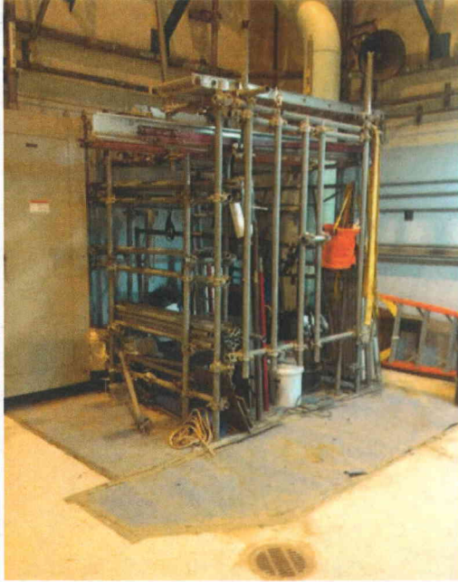
File Name: 1-67-1-1-05.jpeg Description: Scaffolding staging area
