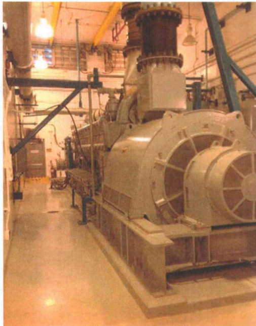
File Name: 1-60-2-1-08.jpeg Description: General view of room
