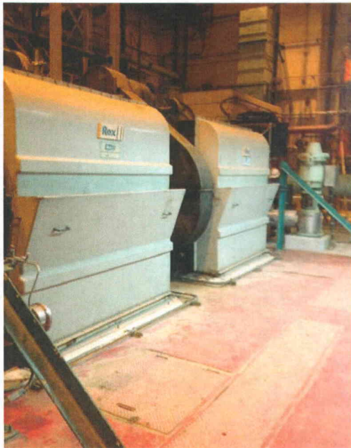
File Name: 1-69-1-1-05.jpeg Description: General view of room
