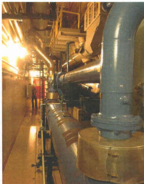
File Name: 1-60-1-1-08.jpeg Description: General view of room
