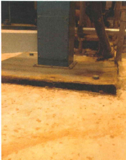
File Name: 1-66-1-1-05.jpeg Description: Close up of anchorage condition
