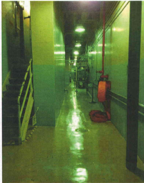
File Name: 1-59-3-1-18.jpeg Description: General view north hallway
