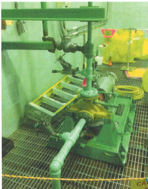
File Name: 1-60-5-1-18.jpeg Description: View of ladder in the area
