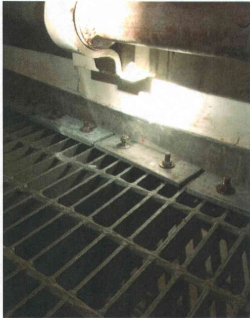
File Name: 1-66-1-1-13.jpeg Description: Loose nut for securing grating.
