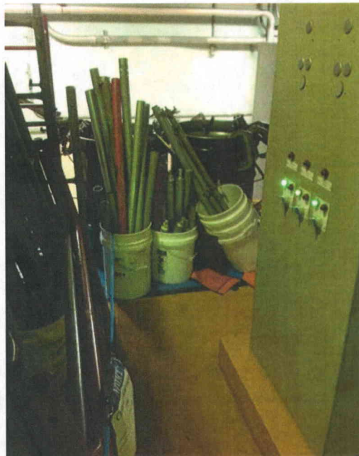
File Name: 1-66-3-1-20.jpeg Description: View of scaffold staging area
