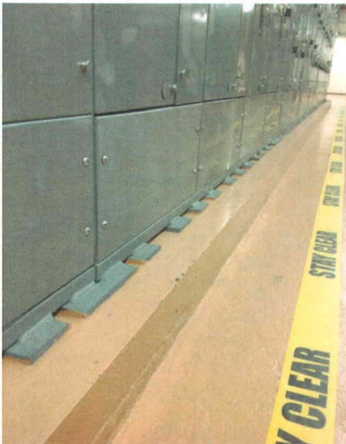
File Name: 1-60-3-1-06.jpeg Description: View of 1R24-S0021 welded to shims
