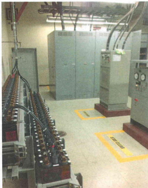
File Name: 1-60-2-1-06.jpeg Description: General view of room
