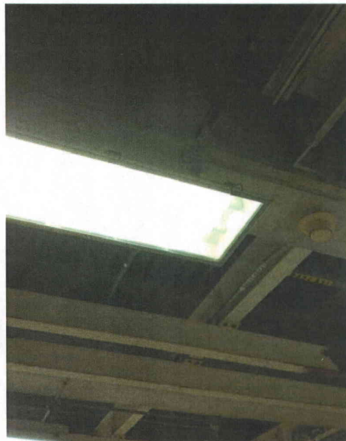
File Name: 1-60-4-1-02.jpeg Description: Protective light cover
