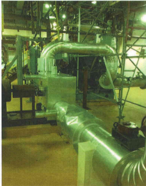
File Name: 1-59-1-1-01.jpeg Description: General view of room
