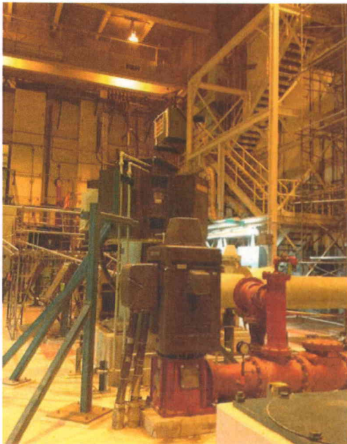
File Name: 1-60-1-1-05.jpeg Description: General view of room
