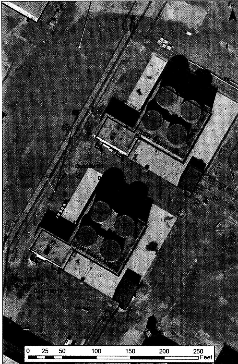
Figure 2.2-2: PMP Sealed Doors Near SSW Pump Houses
