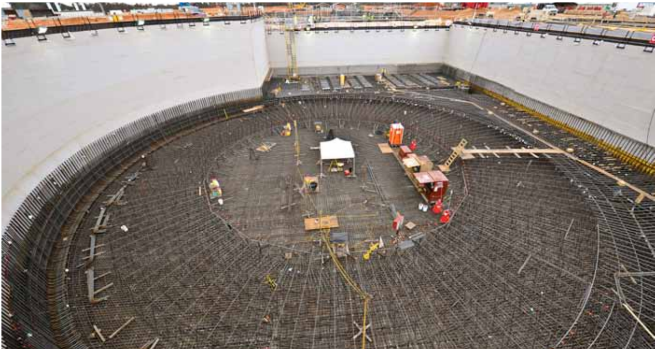
Vogtle Unit 3 nuclear island; rebar placement in preparation for six-foot thick concrete basemat pour.
