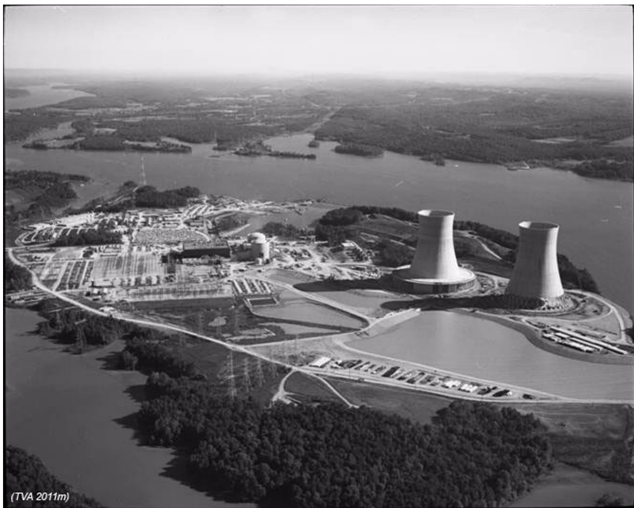
Figure 2.12-4 Oblique Aerial Photograph Taken During SQN Plant Construction
