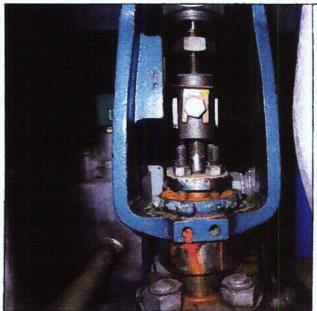
Note: North bank (CV-3-126-10-27) valve showing surface corrosion.
