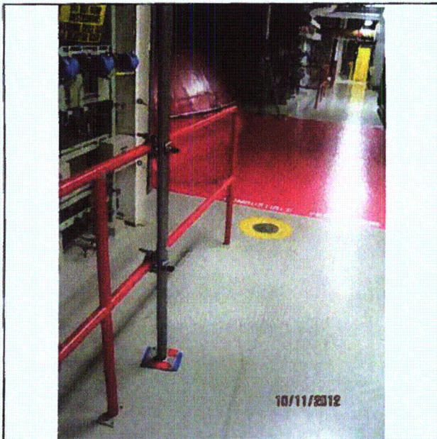
Note: Railing near RK25-6A/B
