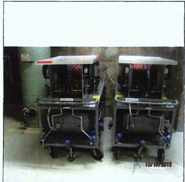
Note: Two wheeled leak test equipment secured.
