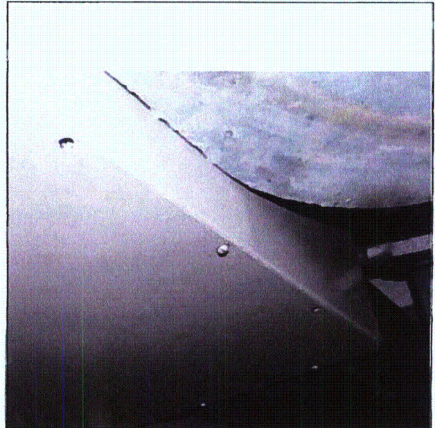
Note: Detail view showing 2 missing screws on access panel.
