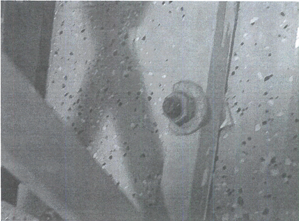
Figure 4 Additional Anchor with Cut Washer
