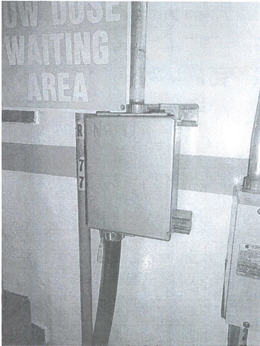
Figure 3: Companion Junction Box for 2T41-N021A Note: Fading ink with component number.
