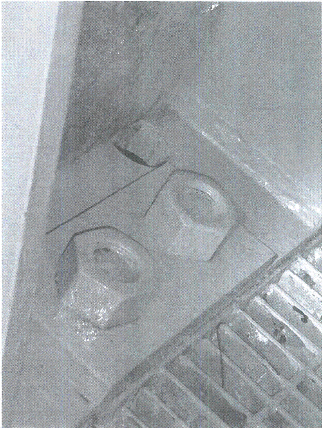
Figure 3 – Bolt Threads below Nut (2E11-B001A)
