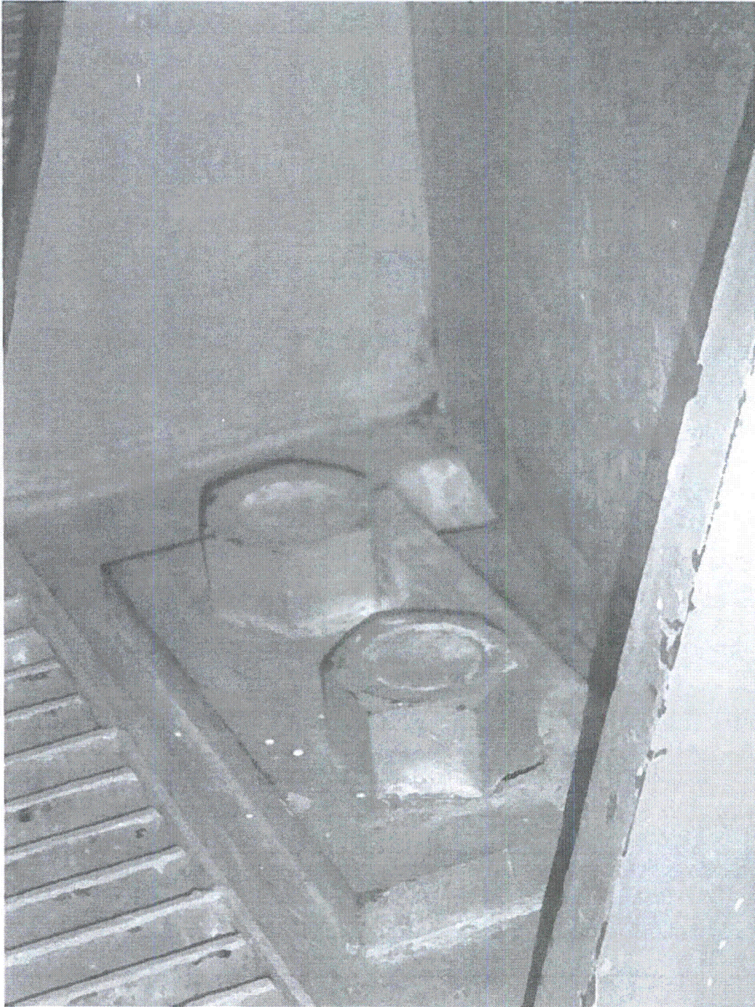
Figure 3 – Bolt Threads Flush with Nut (2E11-B001B)
