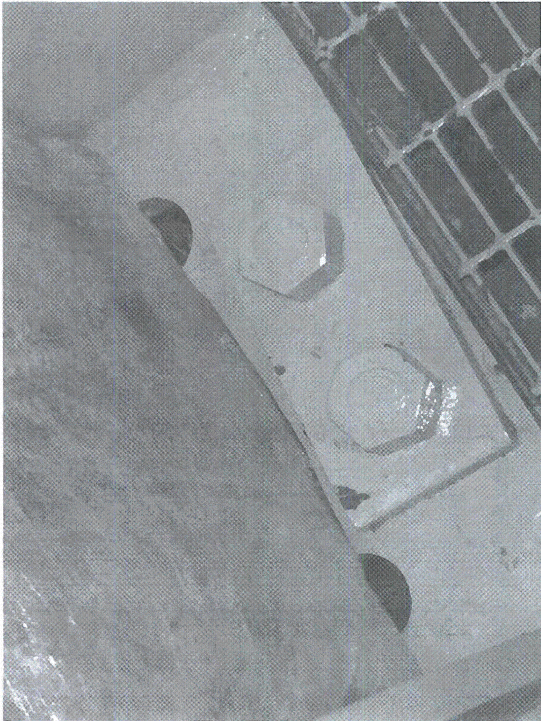
Figure 4 – Bolt Threads Flush with Nuts (2E11-B001A)
