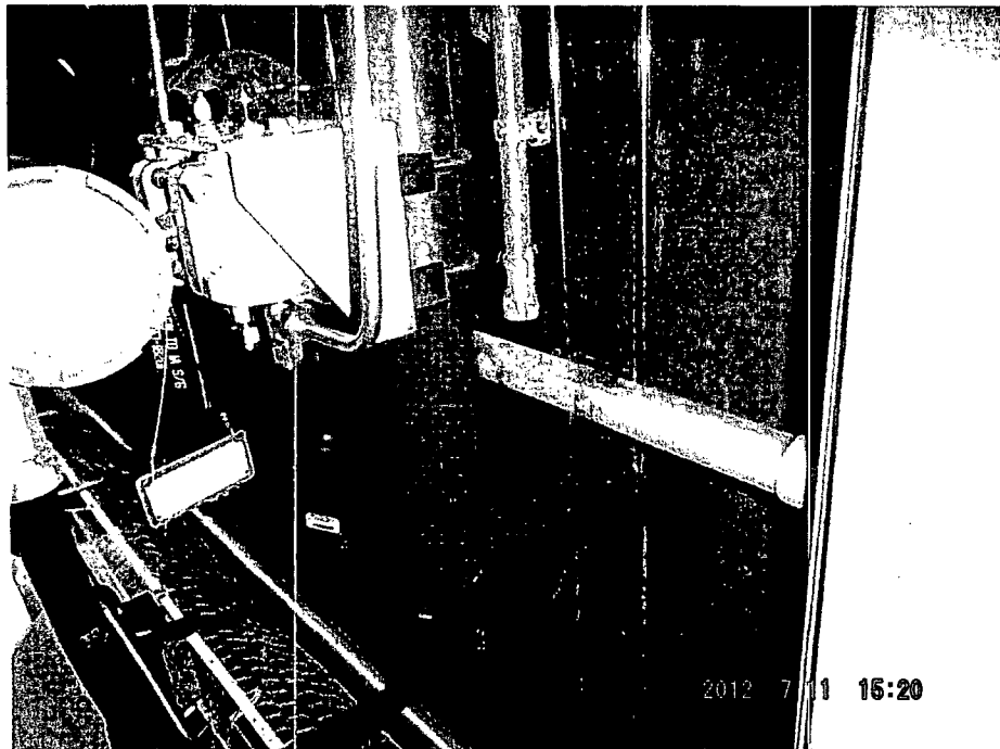
Conduit is in contact with support, but does not seismically challenge the support.
