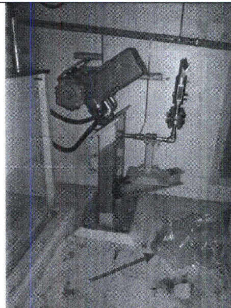
Note: General view of valve area
