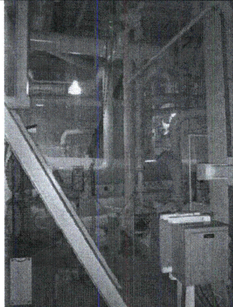
Note: General view of the area
