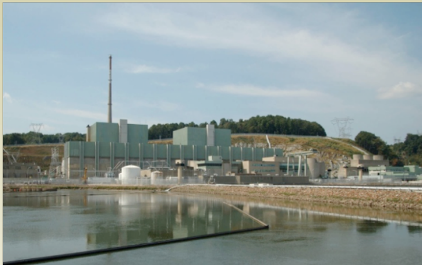
Figure 2.1 Peach Bottom Atomic Power Station (top) and Surry Power Station (bottom).
