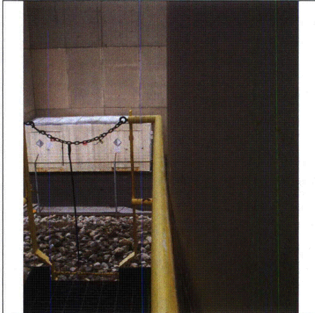
Note: Very small gap between platform and RWST.
