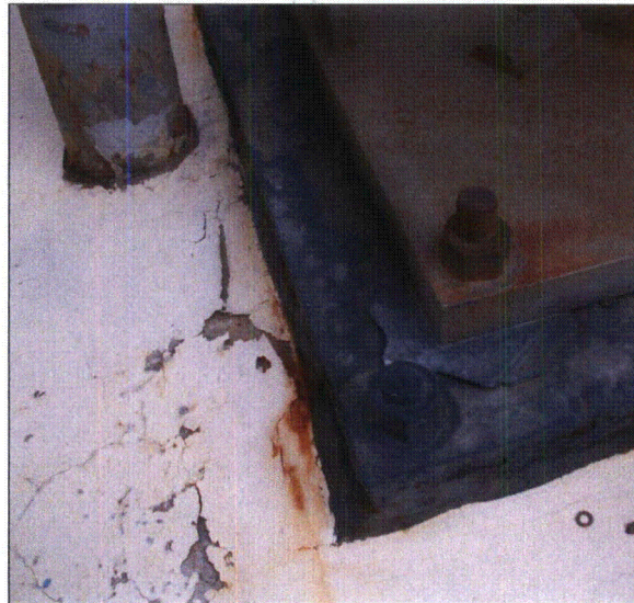
Note: Typical anchor bolt.
