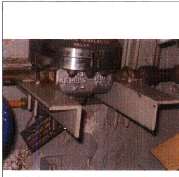
Note: Close up view of its support.
