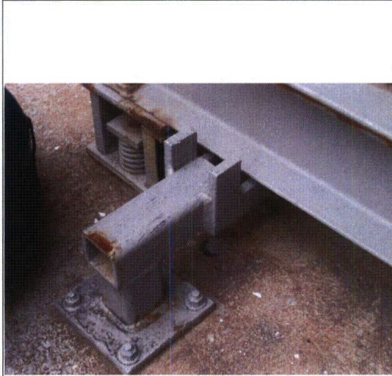
Note: View of the base plate and anchors
