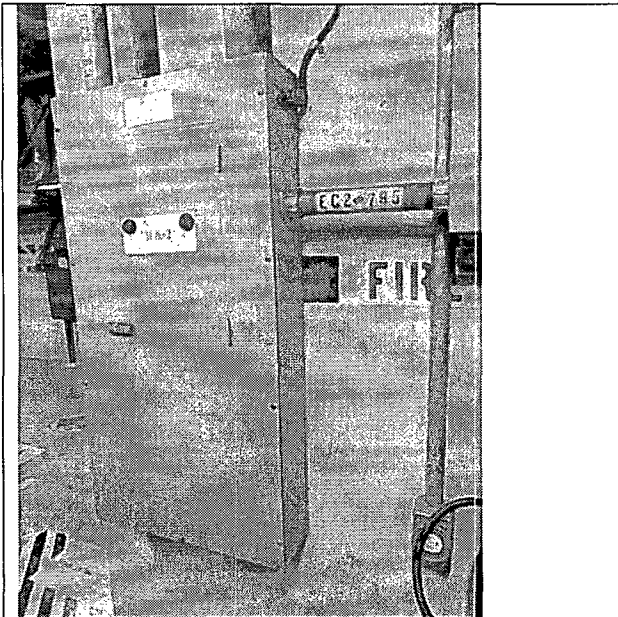
Note: View of panel RA-2 in Room 95.
