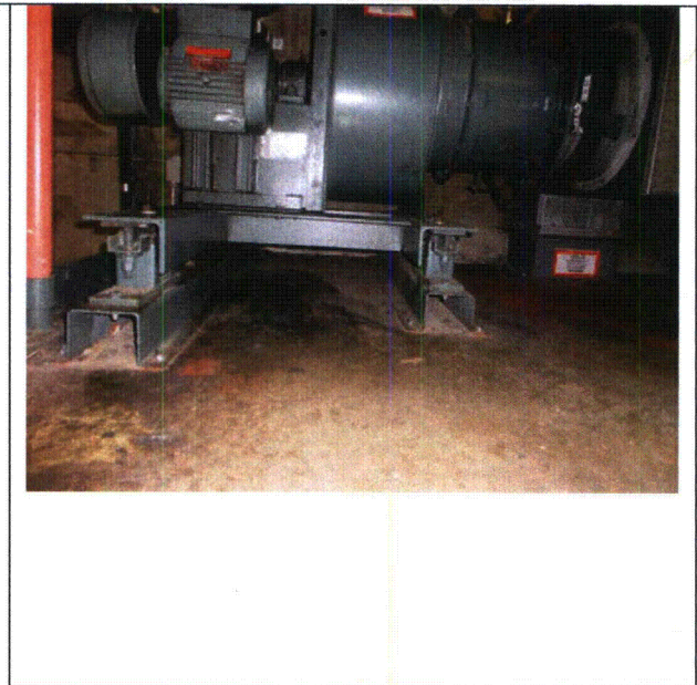
Note: 72FN-46A anchorage
