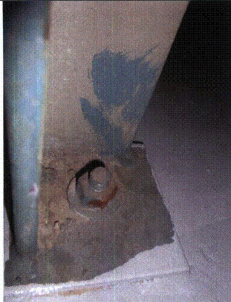
Note: 93AR-A1 anchorage to floor
