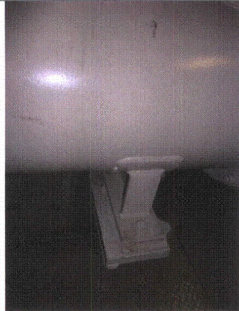
Note: 93WE-1C Anchorage – Fixed Foot
