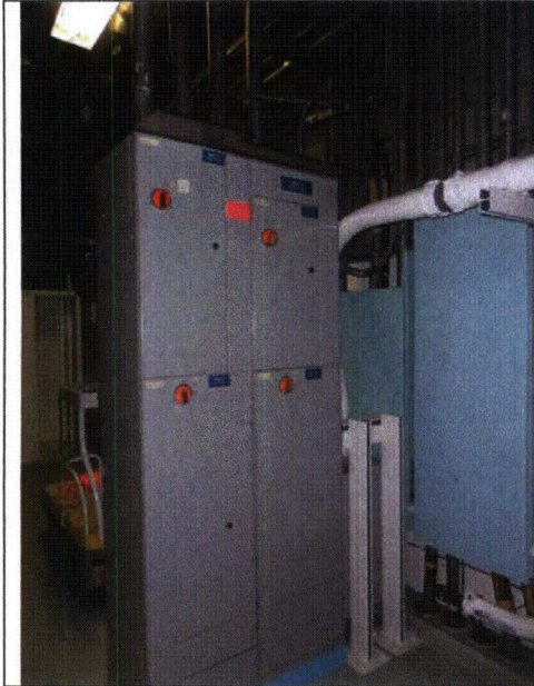
Note: 71BMCC-6 Front View
