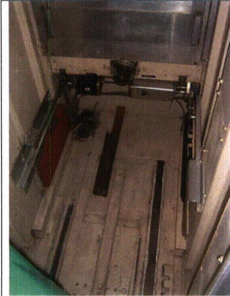
Note: 71-10614 anchorage configuration.
