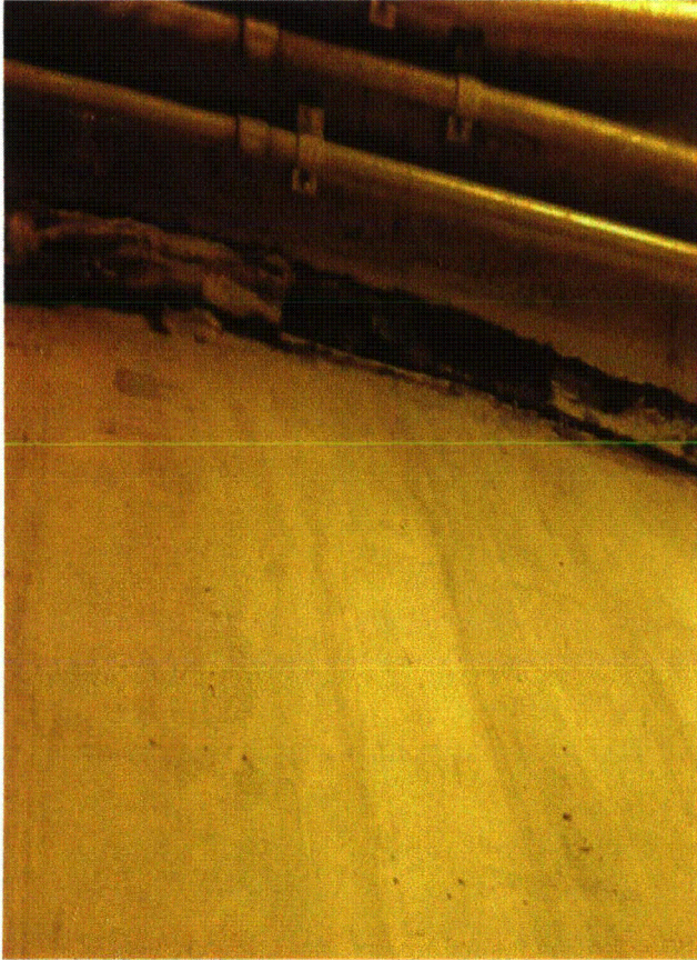
2MS018C (DEGRADED ISO JOINT) Byron 1 & 2 143
