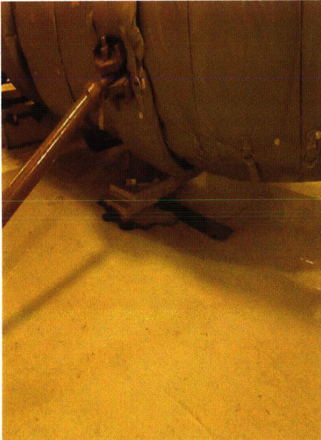
1SX01PB (6695 - concrete cracks) 7-18-12 043
