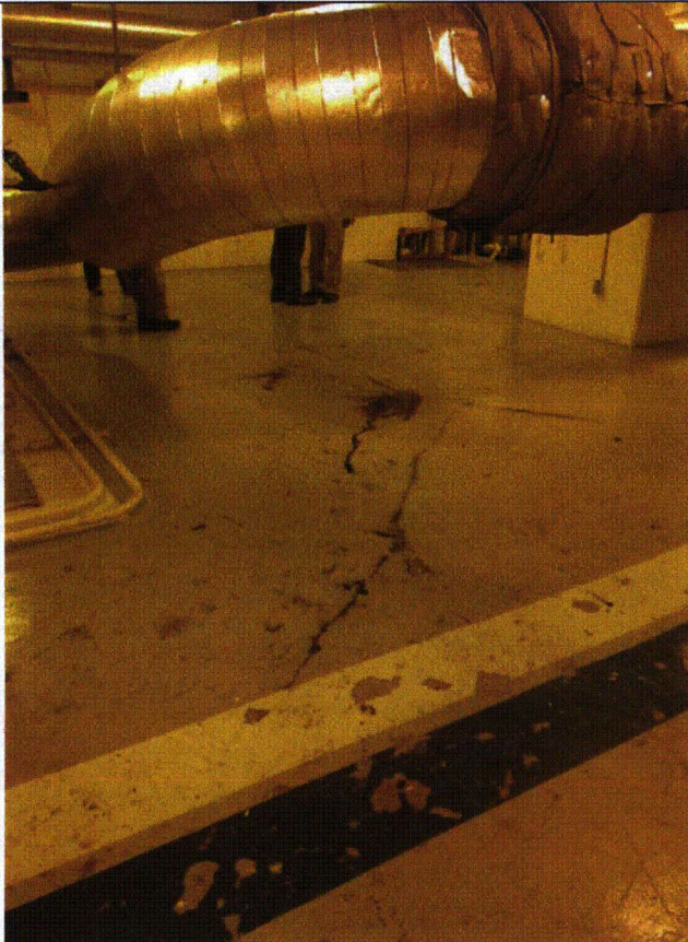
1SX01PB (6695 - concrete cracks) 7-18-12 045
