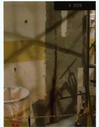
0TI-FC007 (AWB - Water leakage) 7-19-12 033
