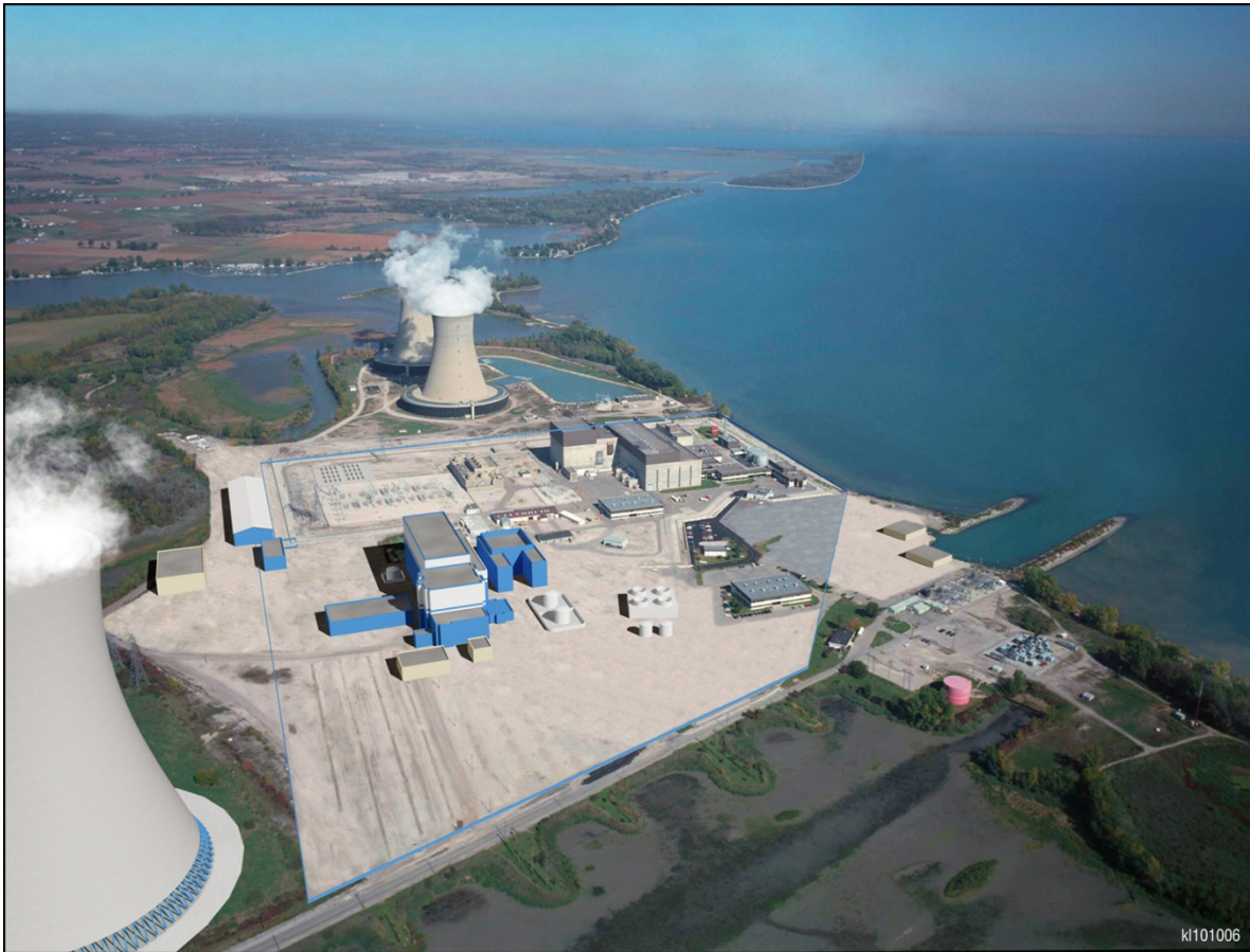
Figure 3-4. Aerial View of the Fermi Site Looking North with Proposed Fermi 3 Structures Superimposed (Detroit Edison 2011b)
