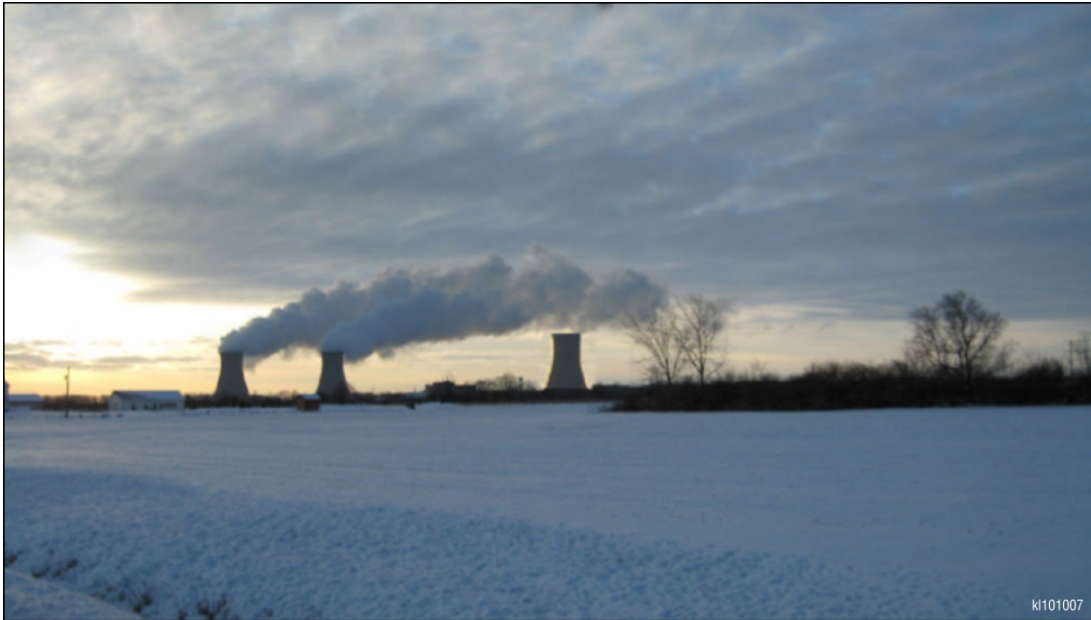
Figure 3-5. View of the Fermi Site from Post Road Looking Southeast: Existing Fermi 2 Cooling Towers Are Shown on the Left; the Proposed Fermi 3 Cooling Tower Is on the Right (Detroit Edison 2011b)
