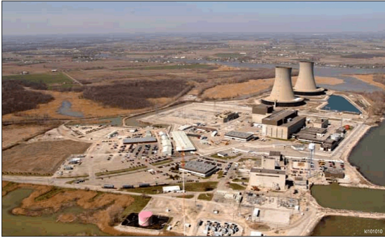
Figure 3-3. Aerial View of the Existing Fermi Site Looking North (Detroit Edison 2011b)
