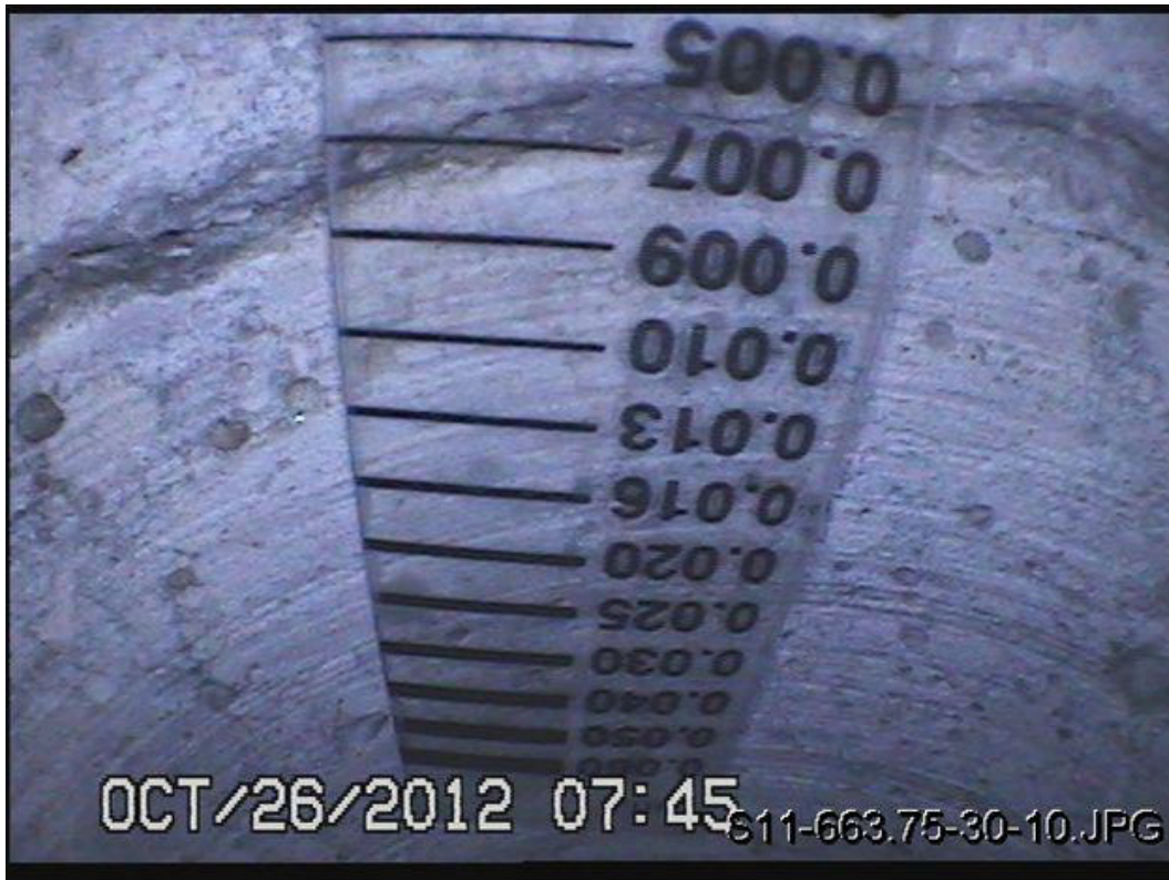
Picture No. 7 – Davis-Besse Shield Building Core Bore Location S11-663.75-30-10
