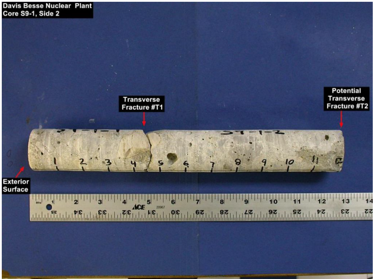
Picture No. 8 – Davis-Besse Shield Building – Core Boring Sample
