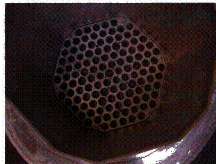
Grid Plate in Core Shroud
