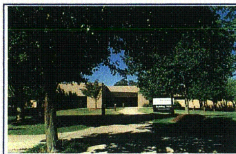
Duke Energy Corporation's Environmental Center
