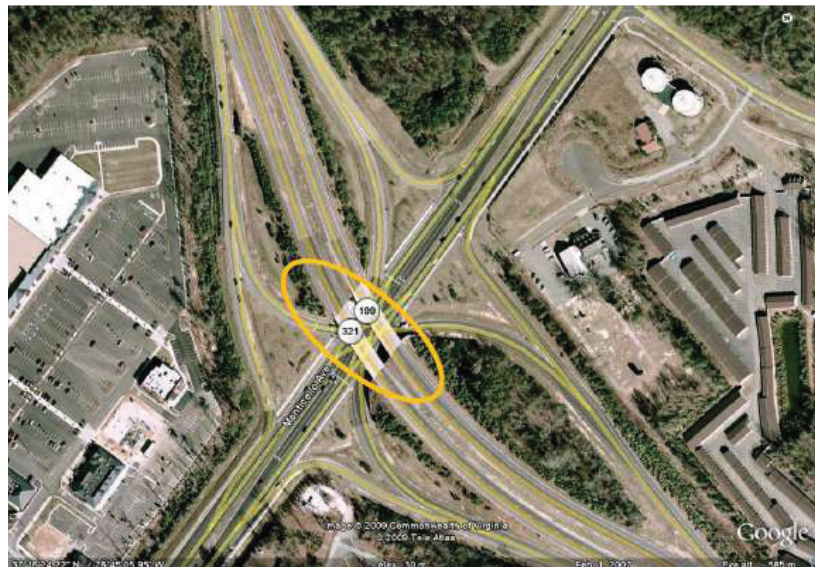
Figure 6-19 Highway 199 Over Highway 321 (Bridge 13 on Figure 6-20)
