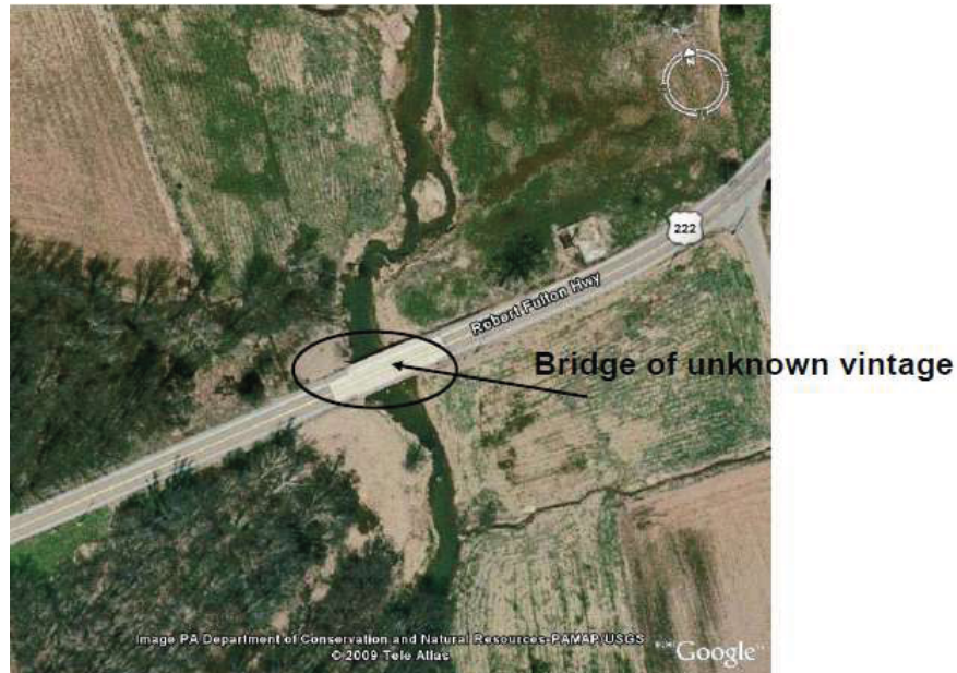
Figure 6-16 Bridge along Robert Fulton Highway
