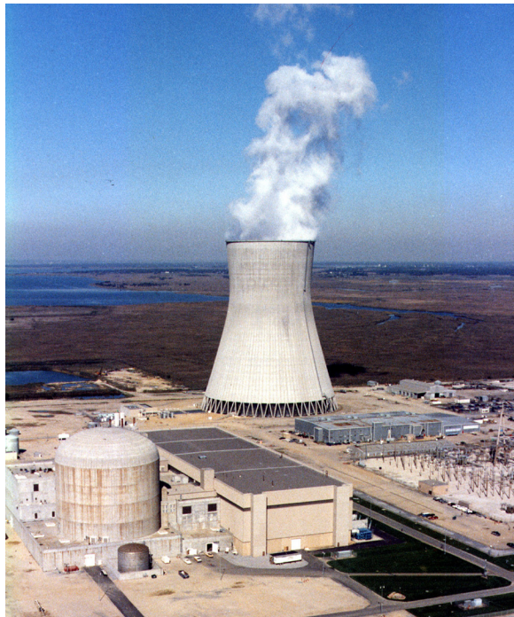
Hope Creek Nuclear Power Plant in New Jersey
