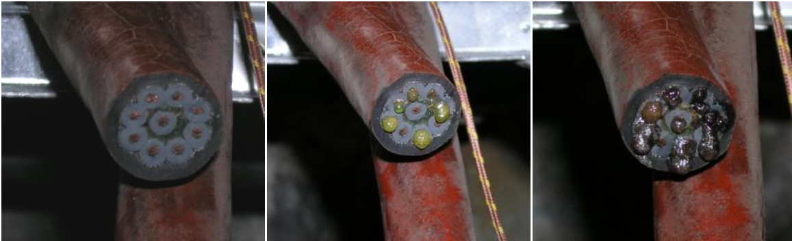
Figure 7.28: Progression of the liquid residue leaking from the cut end of the thermocouple cable: pre-test on the left, and then progressively later in the test for the center and right photos.
