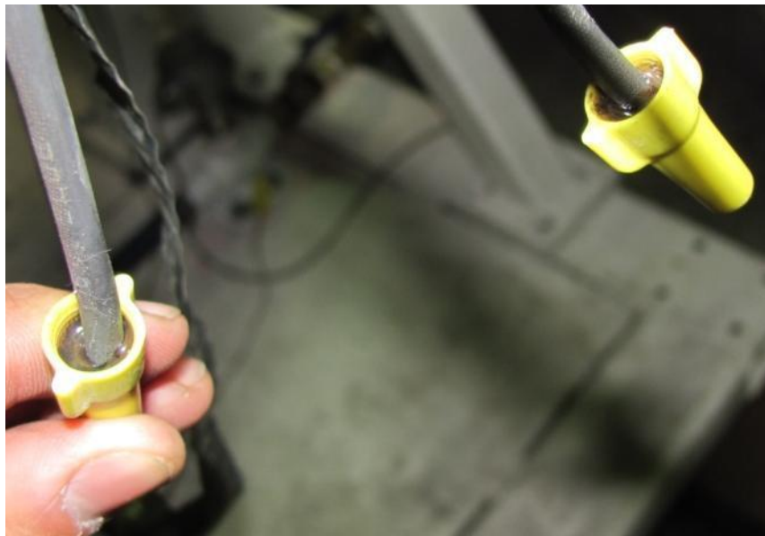
Figure 7.19: Wire nuts containing liquid formed during testing.
